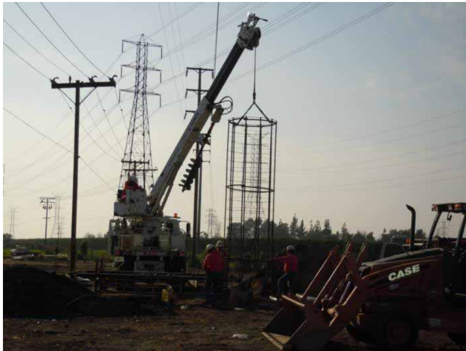
Figure 6: Crews installing foundation cage for a 66 kV riser pole, Segment 8.
