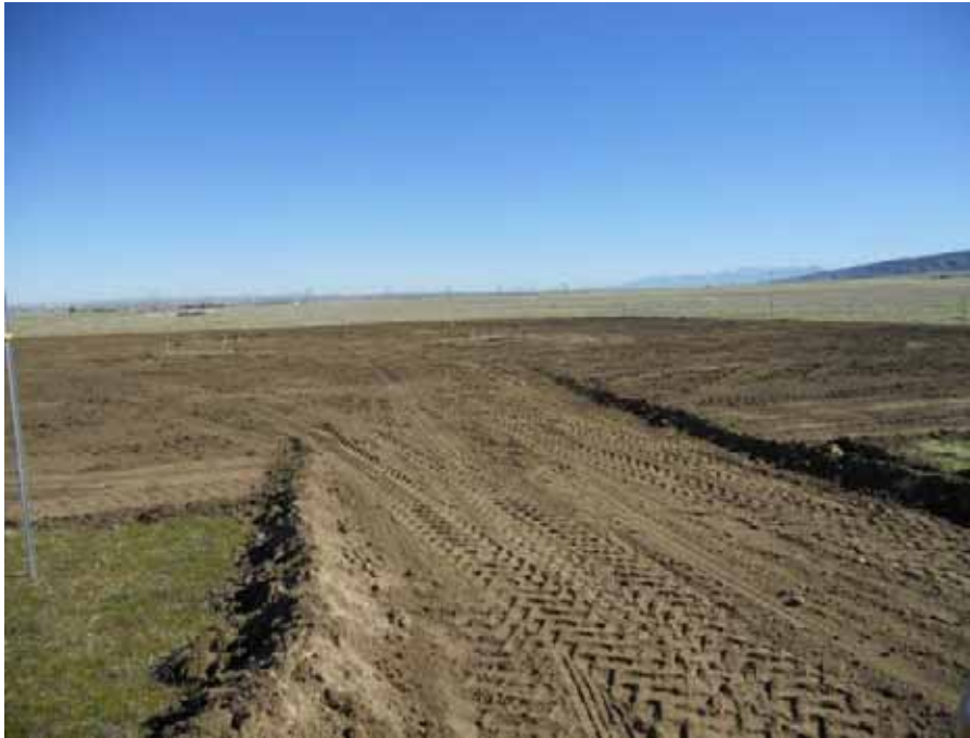
Figure 1: Site preparation for the construction of Tower 46, Segment 4.
