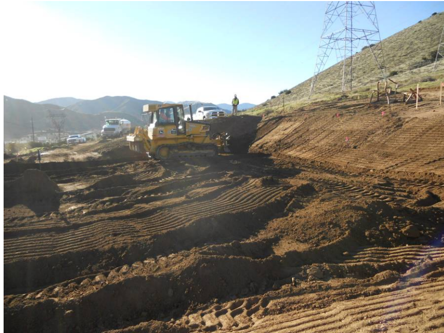
Figure 1: H&H grading disturbance site and new access road at Tower 62, Segment 5.
