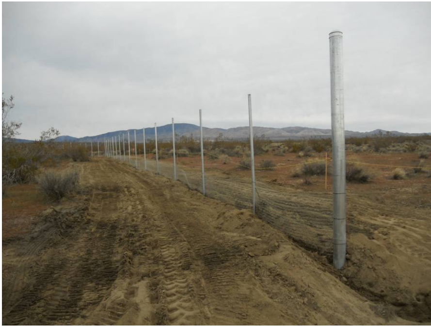
Figure 3: Tortoise fence installation at Whirlwind Substation, Segment 9.
