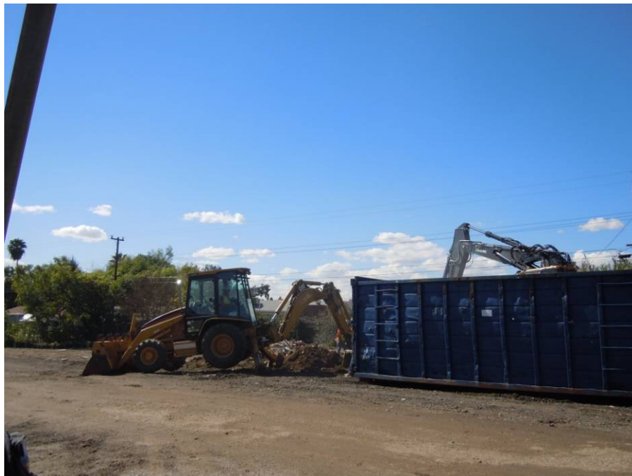
Figure 6: Crews excavating a tower foundation, Segment 7.
