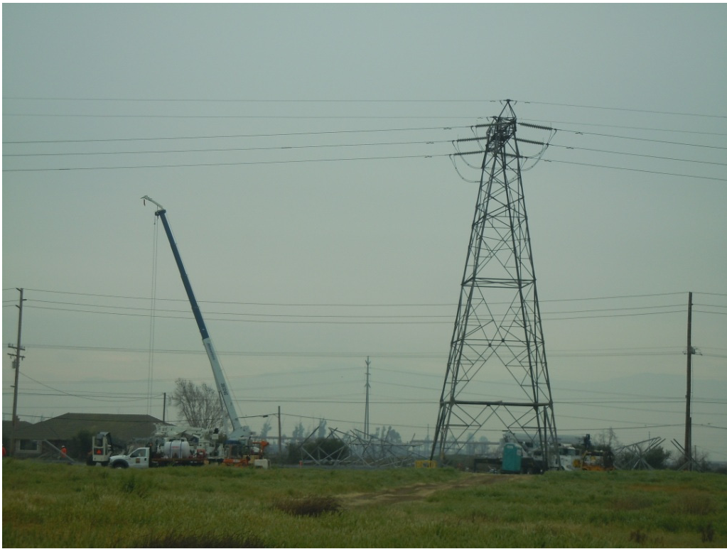
Figure 7: Crews erecting a tower, Segment 8 Phase 2.
