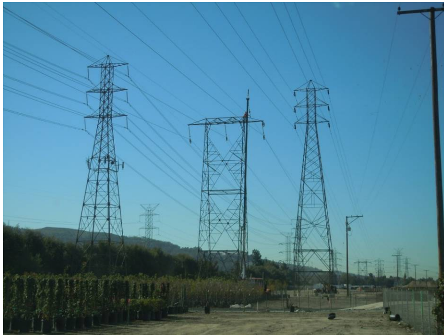
Figure 5: Crews preparing towers for wire removal, Segment 7.
