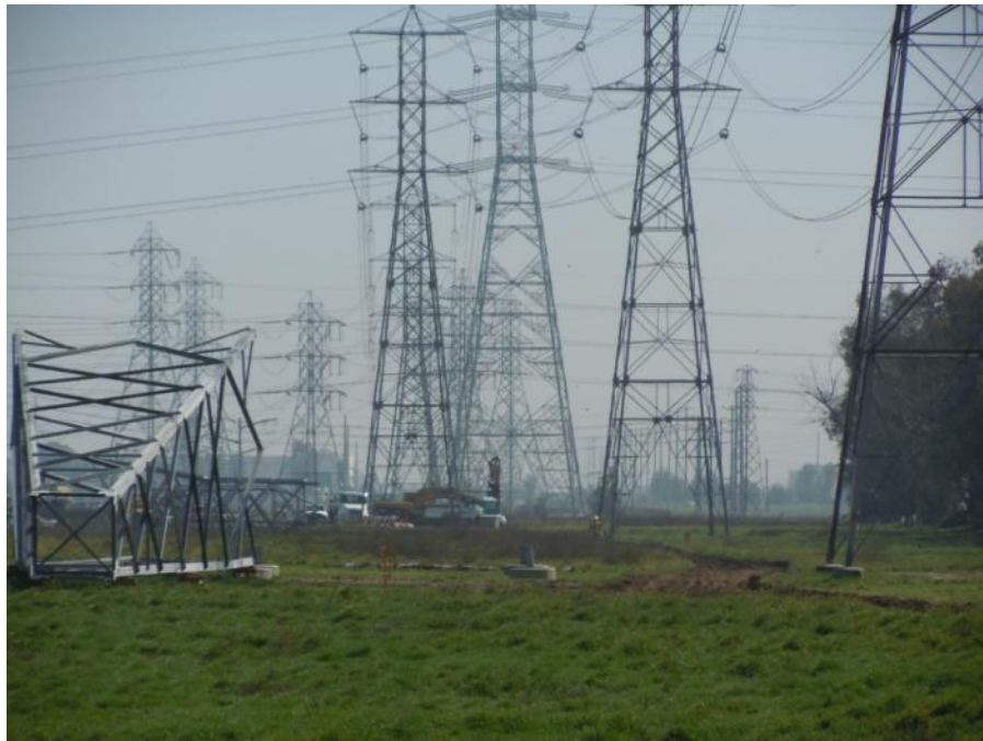
Figure 6: Crews drill a foundation for new 220 kV tower, Segment 8, Phase 2.
