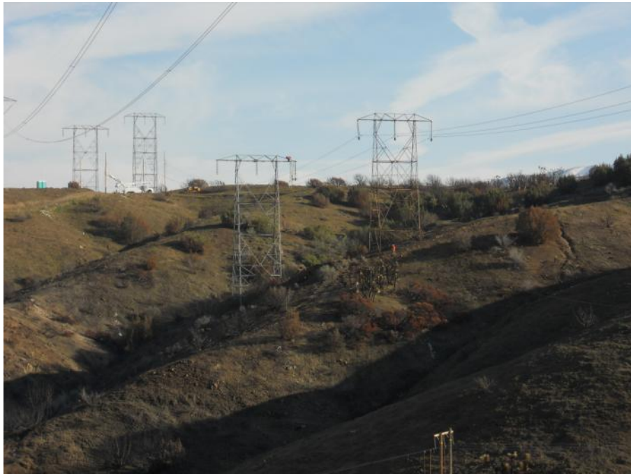
Figure 2: H&M removing wire across Godde Hill Road, Segment 5.
