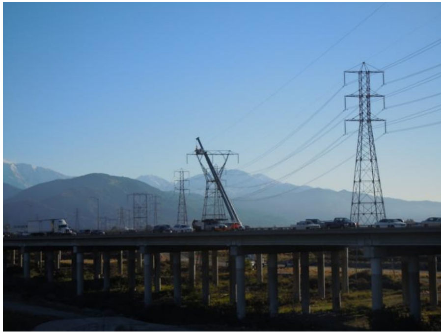
Figure 5: Crews preparing to remove conductor across Interstate 605, Segment 7.
