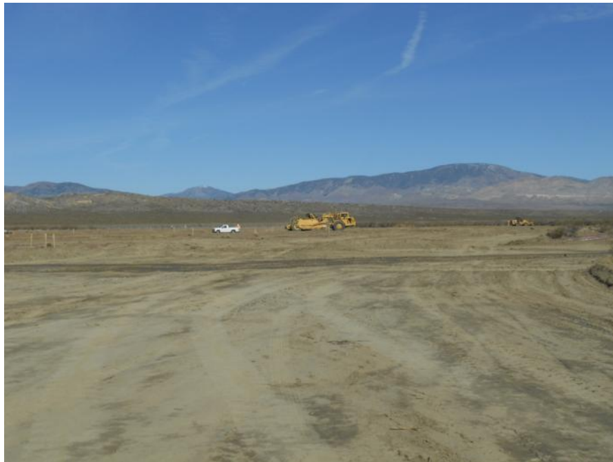
Figure 4: Grubbing and grading at Whirlwind Substation, Segment 9.
