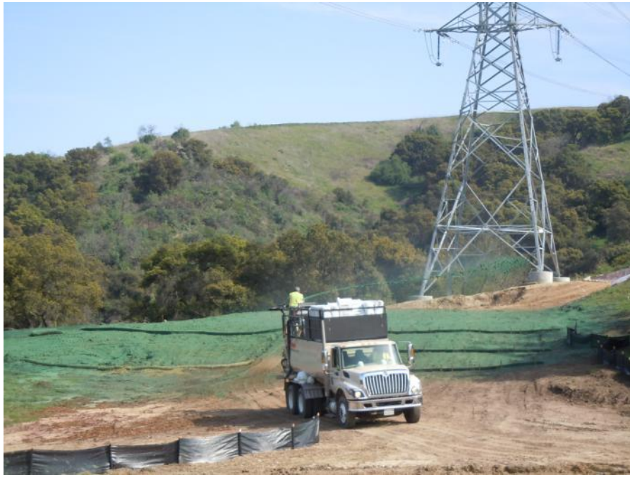
Figure 7: Crews spraying a soil binder for erosion control, Segment 8, Tonner Canyon.
