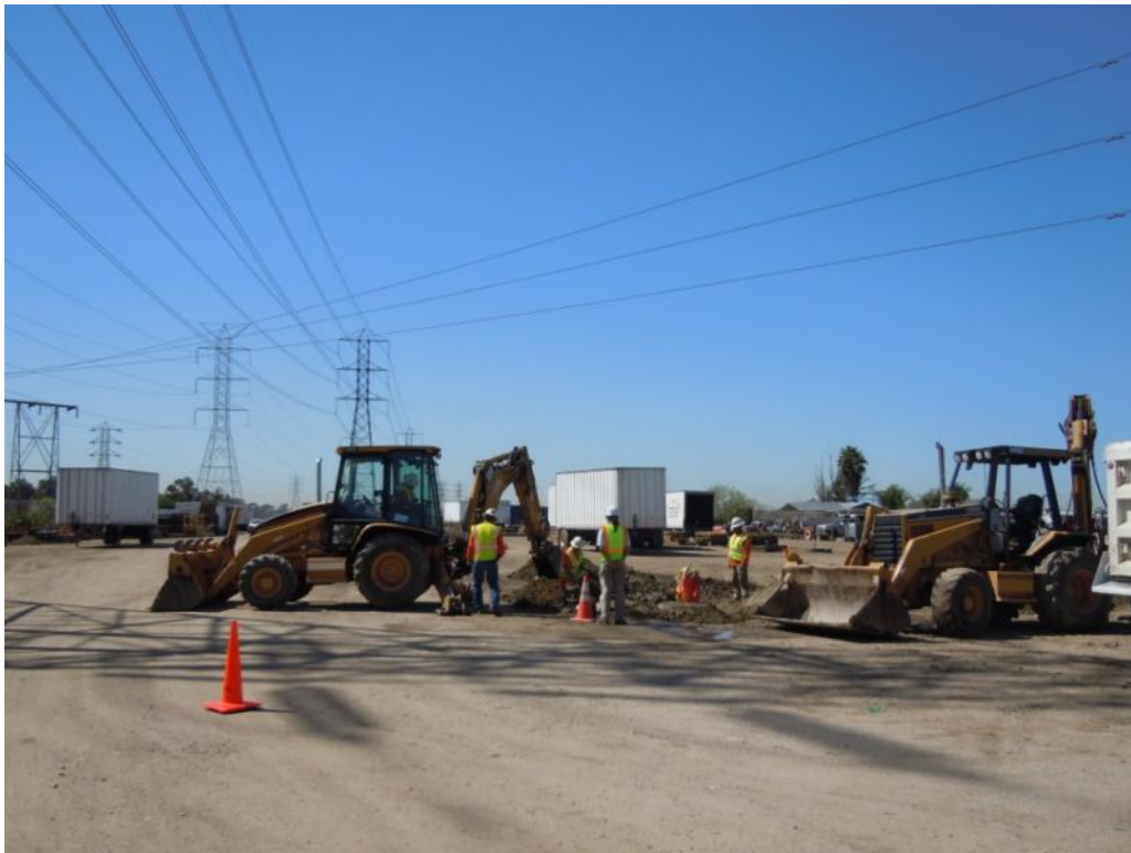
Figure 6: Crews excavating a foundation, Segment 7.
