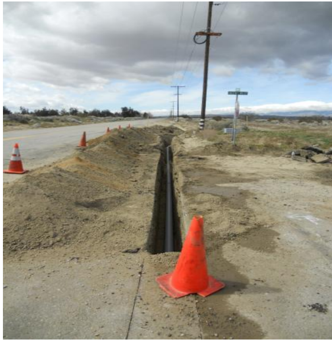
Figure 3: Segment 10 Telecom trenching along Rosamond Boulevard and 140 th Street.
