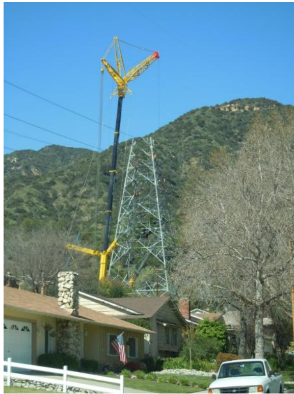
Figure 7: Crews erect Tower M54-T3a in the City of Duarte, Segment 7.
