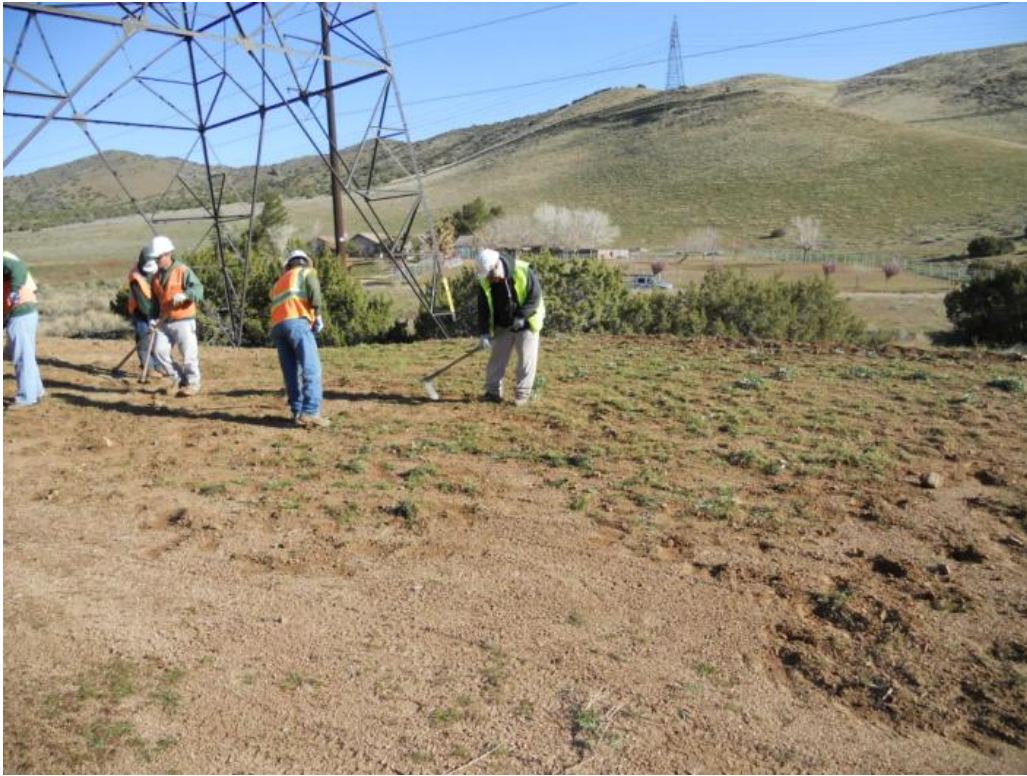
Figure 1: Nature's Image restoration crew conducting decompaction work at Tower 104-2, Segment 2.
