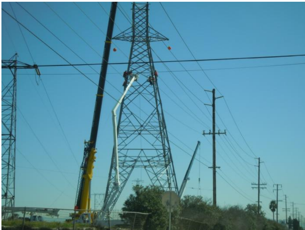
Figure 8: Crews assemble Tower M2-T3, Segment 8, Phase 2.
