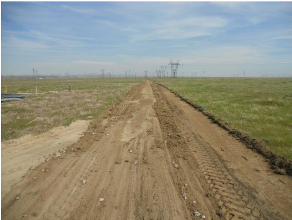
Figure 2: Heavy improvement access road widening towards the Antelope Substation, Segment 4.
