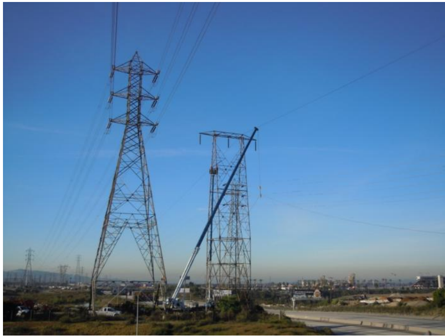
Figure 5: Crews removing conductor across Interstate 605, Segment 7.
