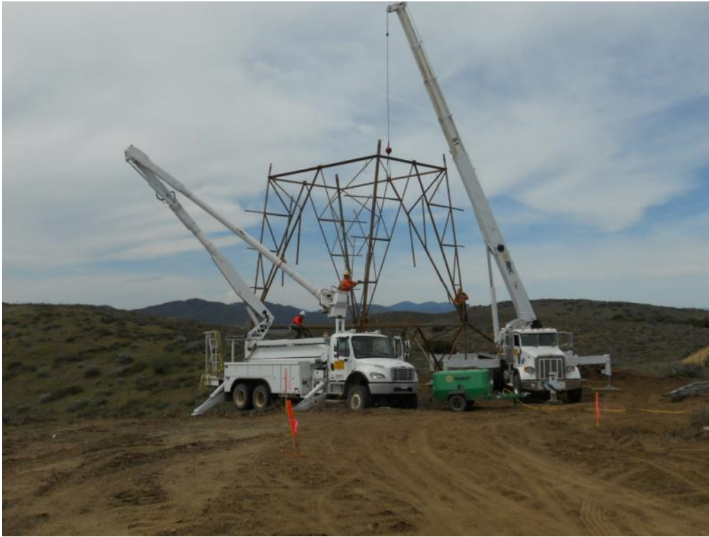
Figure 1: Wreck-out of existing 220 kV Tower M65-T1, Segment 5.
