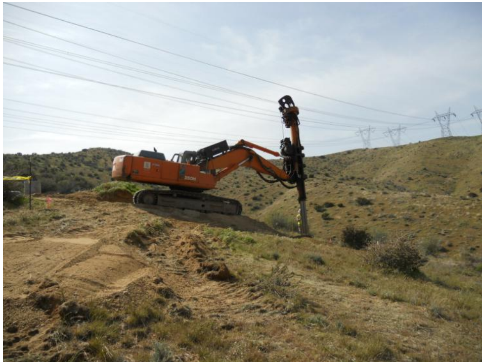
Figure 2: Woodward Brothers drilling foundations at Tower 50, Segment 5.
