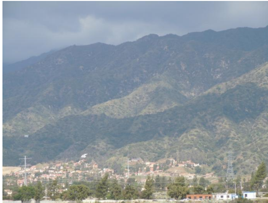
Figure 6: New tubular steel poles and lattice tower in the City of Duarte, Segment 7.
