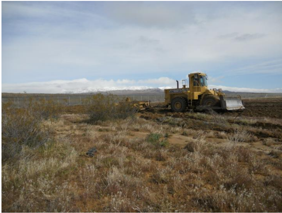
Figure 3: Grubbing of jurisdictional drainage in Whirlwind Substation, Segment 9.
