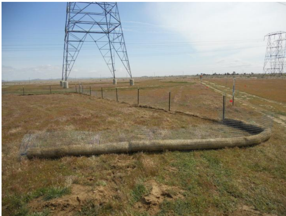
Figure 2: Tortoise fence installed around Tower 20 disturbance area, Segment 4.
