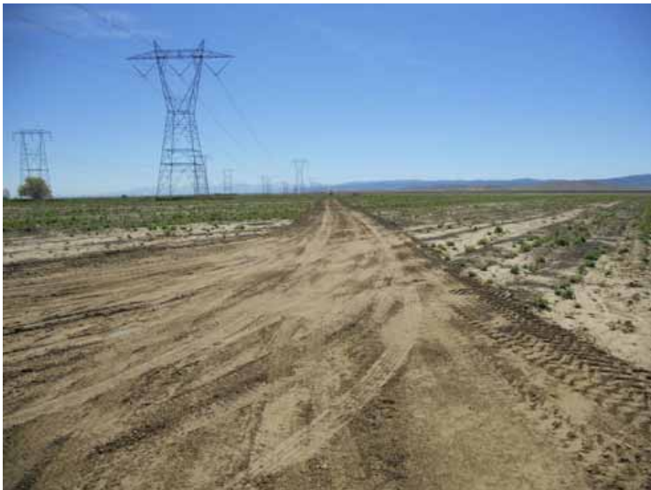
Figure 2: Newly graded access road that leads to Tower 10, Segment 4.
