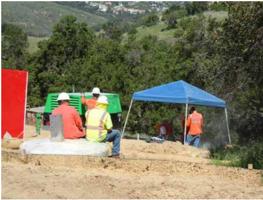
Figure 7: Tri-State crews repair a foundation within Tonner Canyon, Segment 8, Phase 1.
