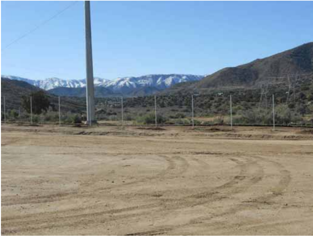
Figure 1: Perimeter fence installation at the Vincent Substation Expansion, Segment 9.
