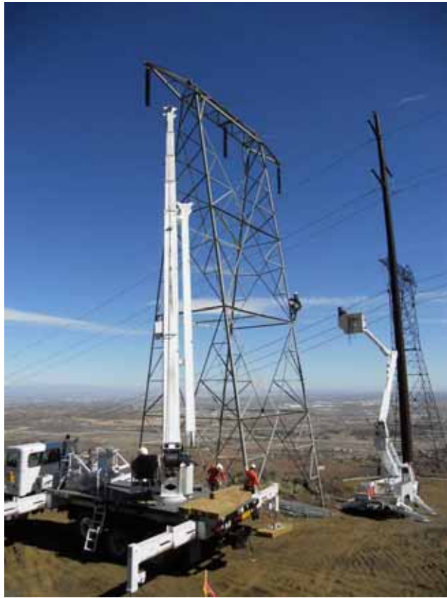
Figure 3: H&M steel crew wrecking out existing 220 kV Tower M22-T3, Segment 5.
