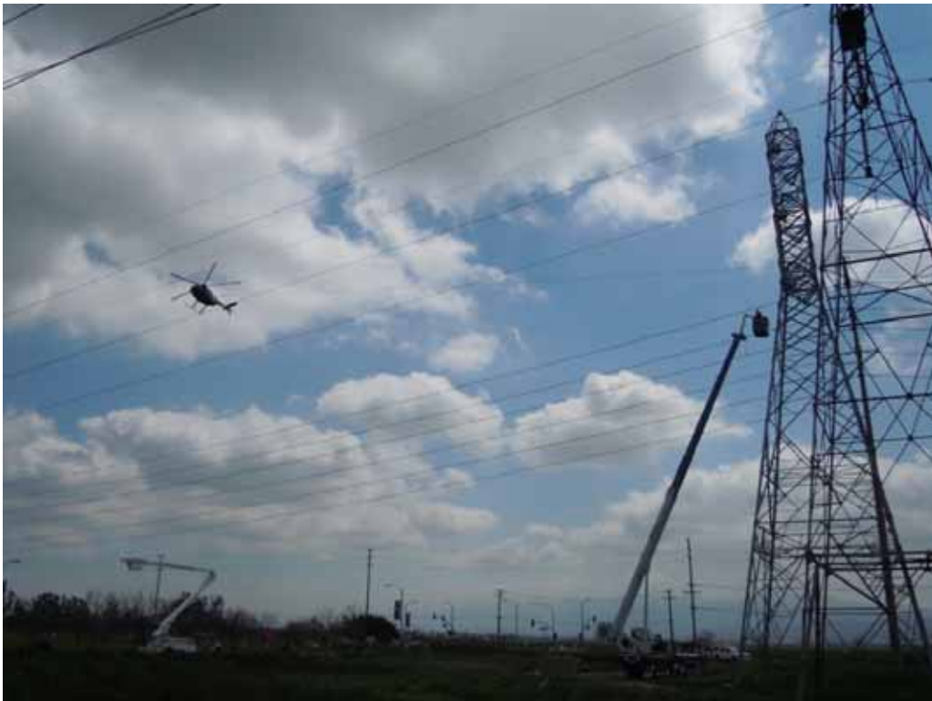
Figure 8: A helicopter pulls a sockline during wire stringing on Segment 8, Phase 2.
