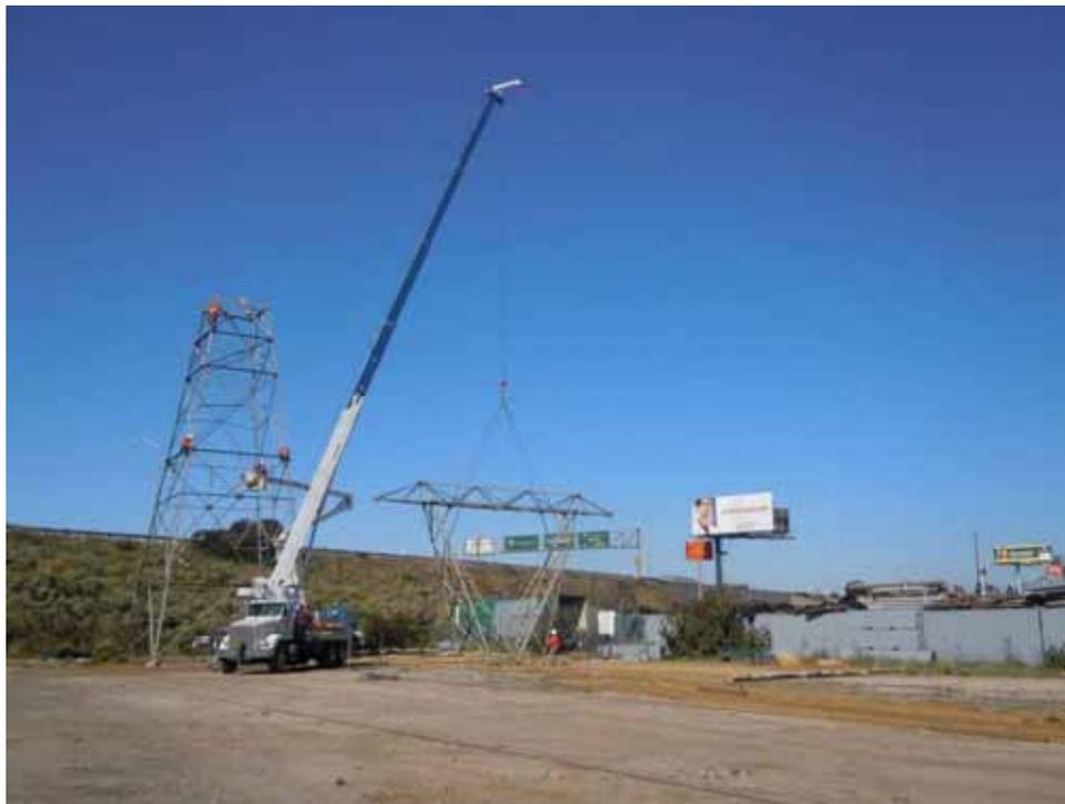
**Figure 6:** Crews disassemble a tower in the Huntington Yard, Segment 7.
