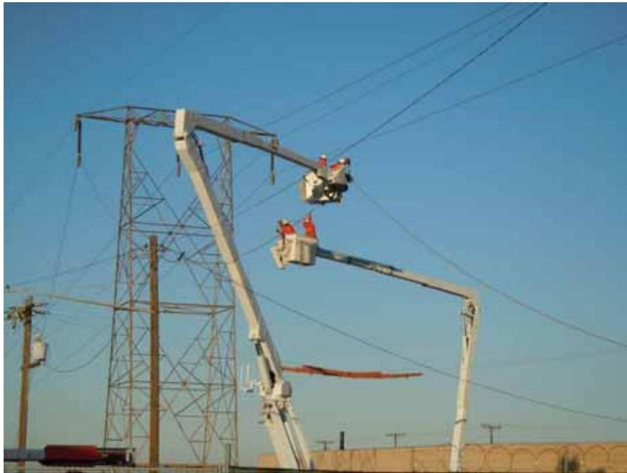
**Figure 5:** Crews remove conductor in the City of Duarte, Segment 7.
