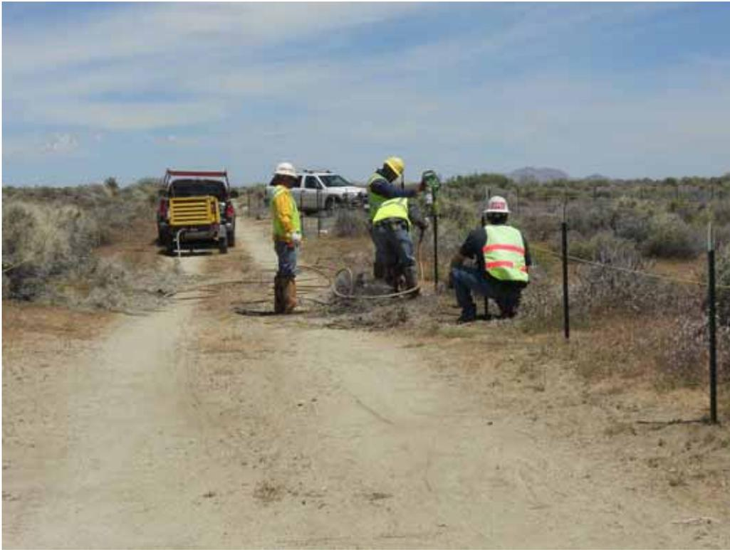
**Figure 3:** Moore Fence Company installing t-posts for the no-dig tortoise fence along General Petroleum Access Road, Segment 10.
