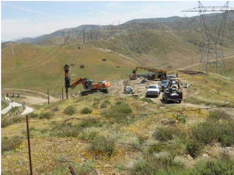
**Figure 2:** Woodward Brothers (drilling contractor) foundation drilling at Tower 45, Segment 5.
