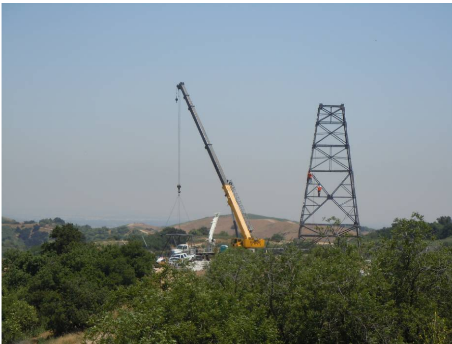
Figure 4: Crews assemble a tower in Tonner Canyon, Segment 8, Phase 1
