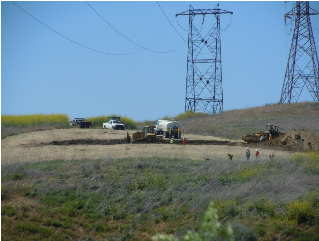
Figure 7: Crews prepare a tower crane pad, Segment 8, Phase 4.
