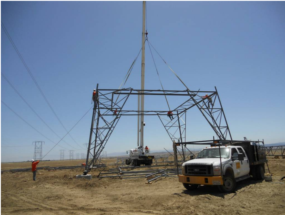
Figure 2: H&M steel crew erecting Tower 11, Segment 4.
