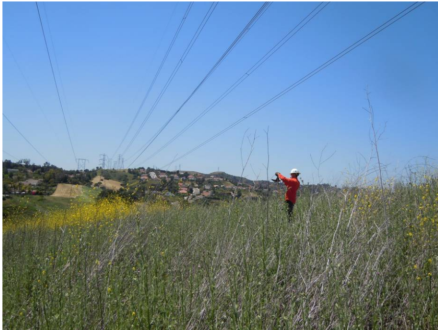
Figure 6: A Wilson environmental crew member brushcuts a tower site, Segment 8 Phase 4.
