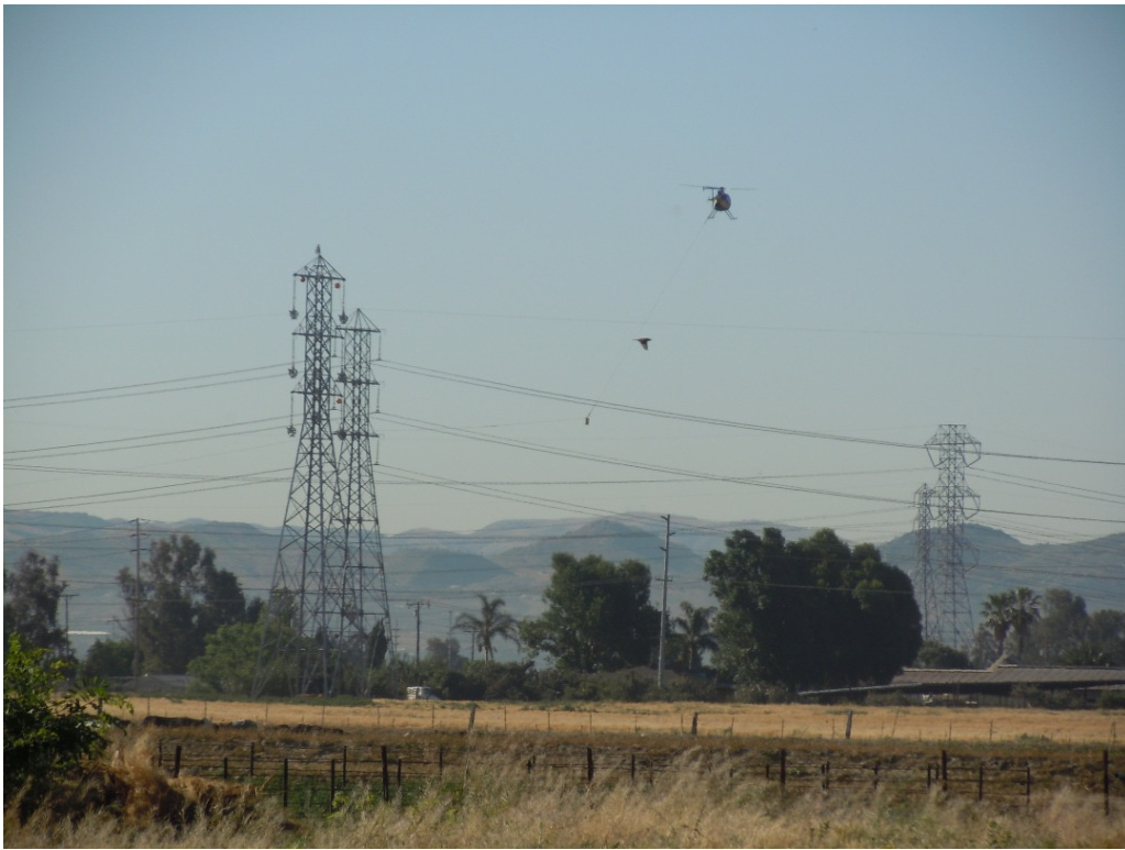
Figure 5: A helicopter pulls a sockline, Segment 8, Phase 2.
