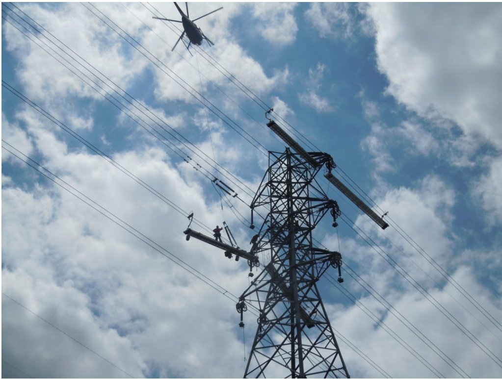
Figure 7: A helicopter delivers an insulator to a new tower, Segment 8, Phase 4.
