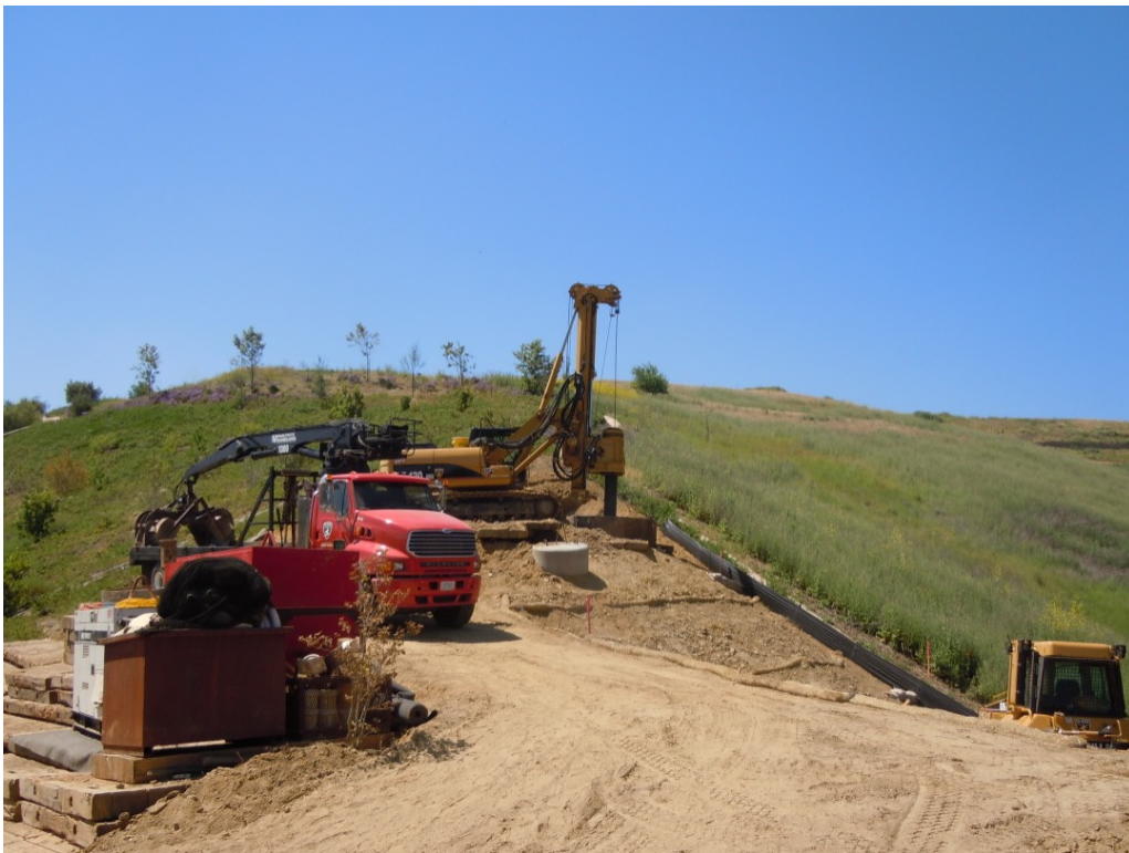
Figure 6: Foundation drilling at Tower M60-T2, Segment 8, Phase 1.
