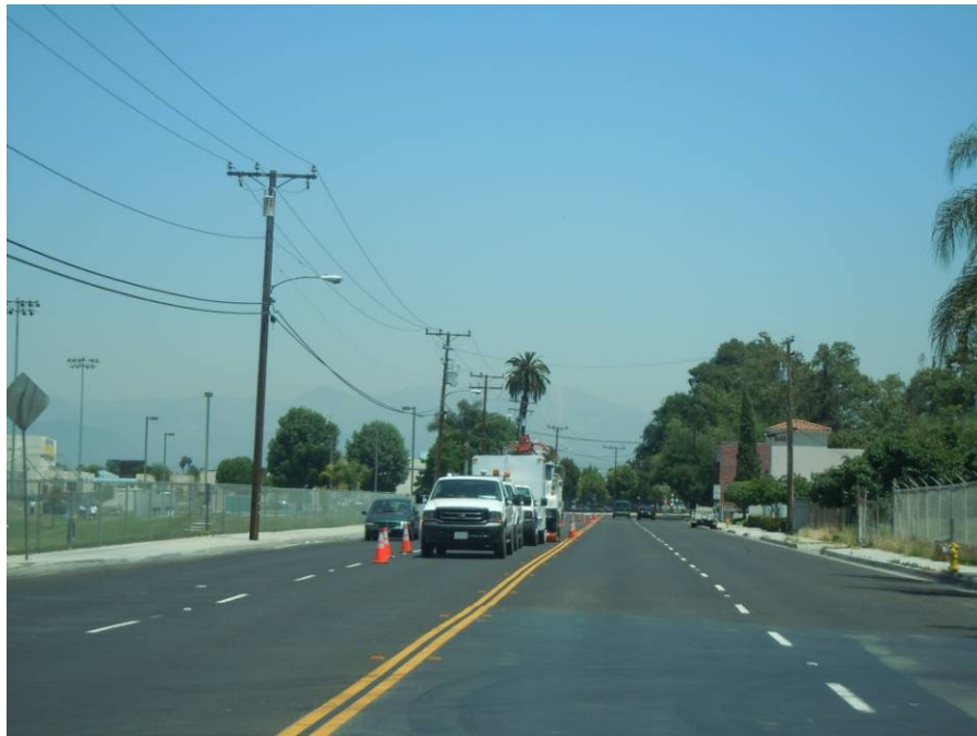
Figure 4: SCE crews staged at a vault on the underground Rio Hondo–Amador-Jose-Mesa line, Segment 7, 66 kV
