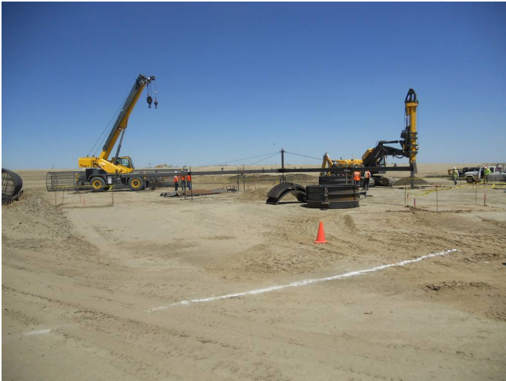
Figure 2: KV Structures drilling Tower 92 inside the Whirlwind Substation, Segment 10.
