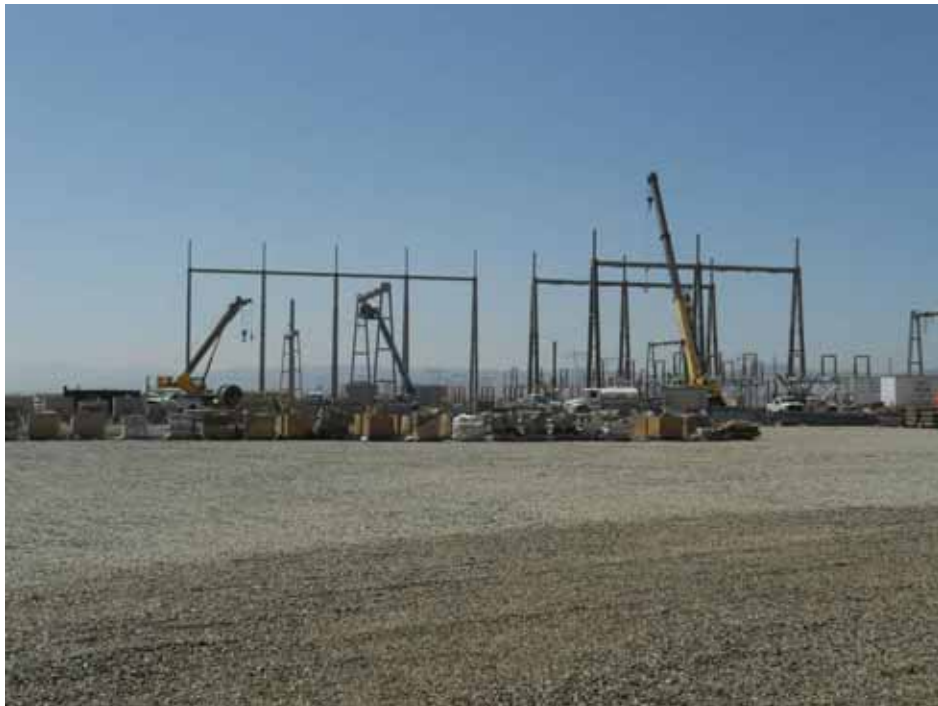
Figure 4: Steel erection in the 220 kV area of Whirlwind Substation, Segment 9.
