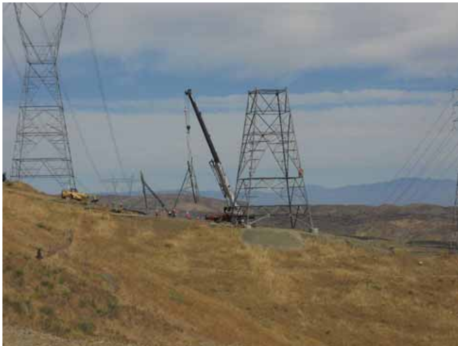
Figure 2: H&M steel crew erecting Tower 43, Segment 5.
