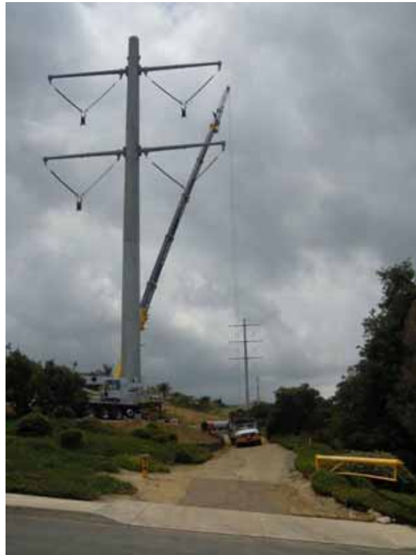
Figure 8: Crews set a TSP, Segment 8, Phase 1.
