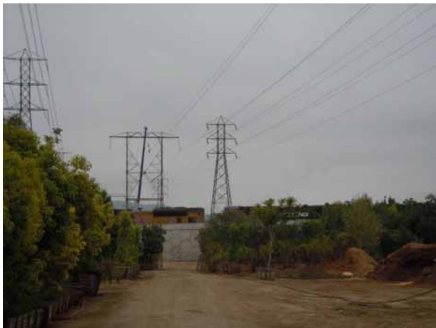
Figure 6: Crews remove conductor, Segment 7.
