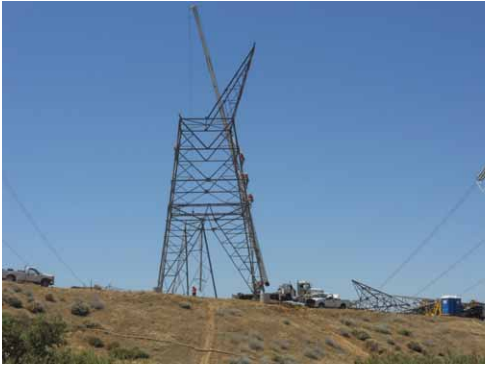
Figure 3: H&M steel crew assembling and erecting Tower 16, Segment 5.
