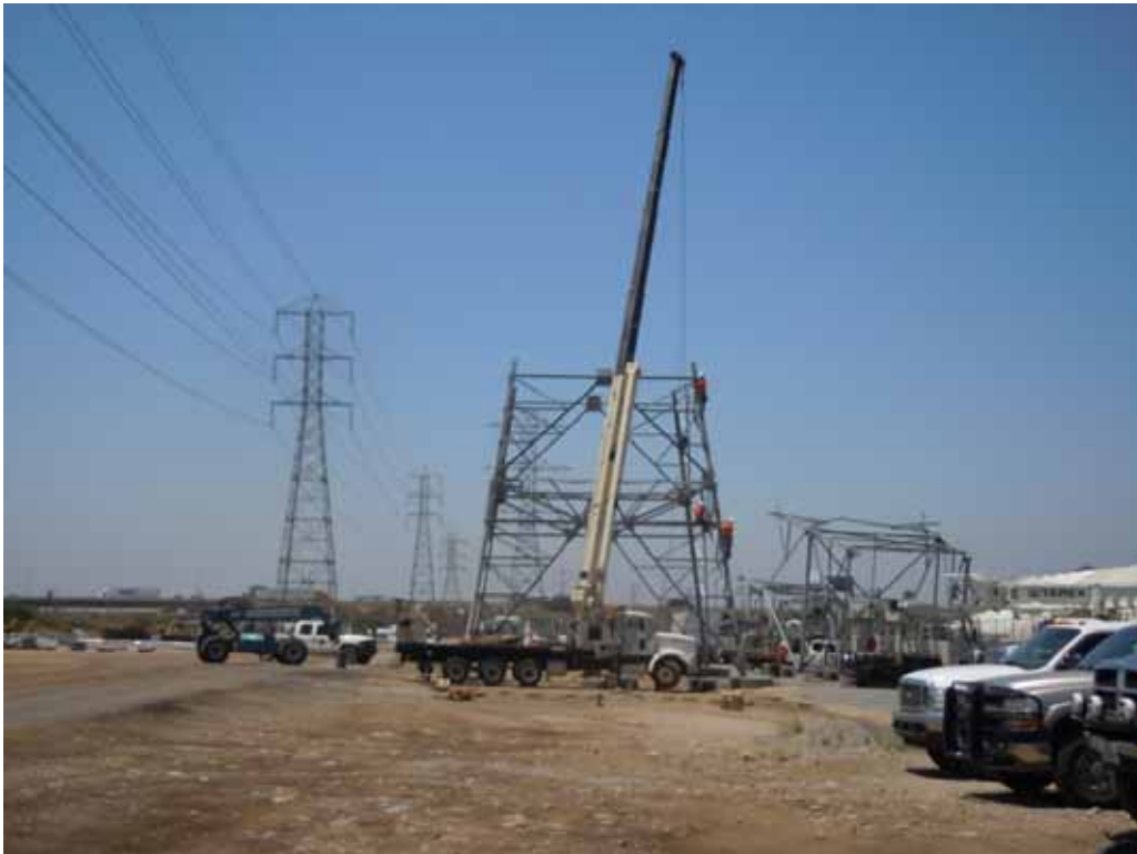
Figure 4: A Wilson crew assembles a tower in the Huntington Yard, Segment 7.
