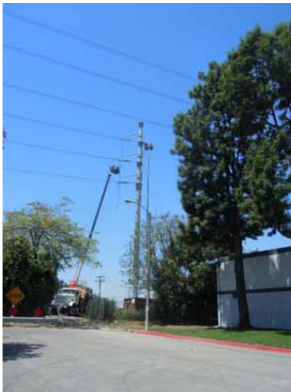
Figure 6: Crews string a shoofly pole near I-605, Segment 8 Phase 4.
