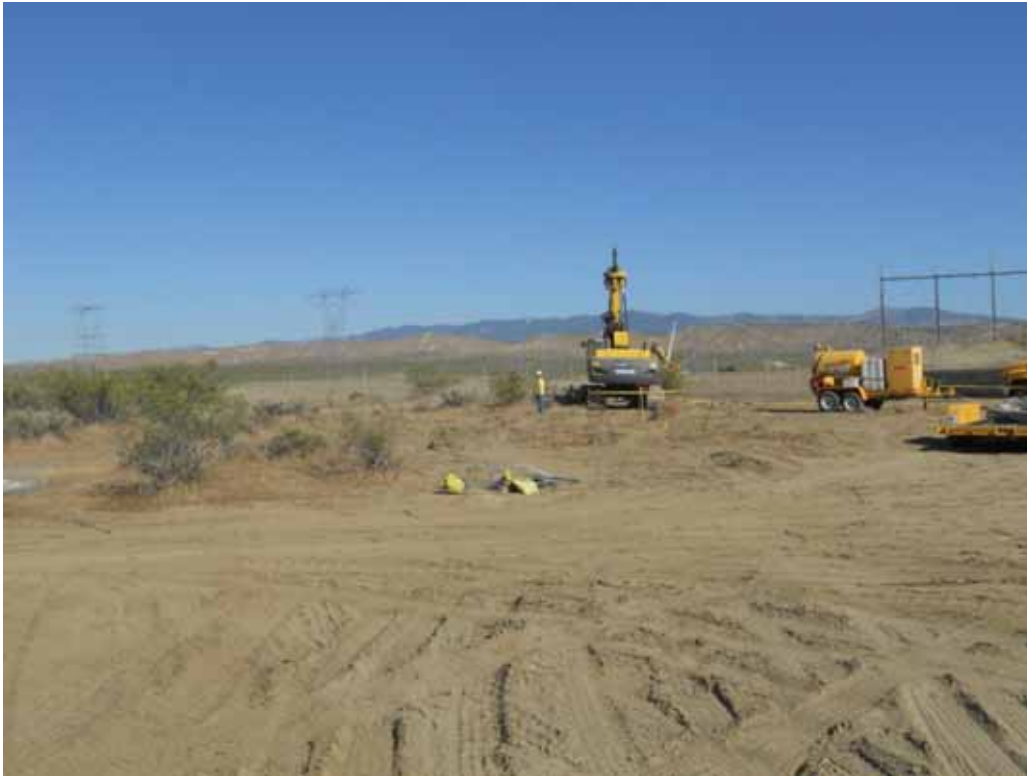
Figure 1: KV Structures drilling Tower 1 (just outside Whirlwind Substation), Segment 4.
