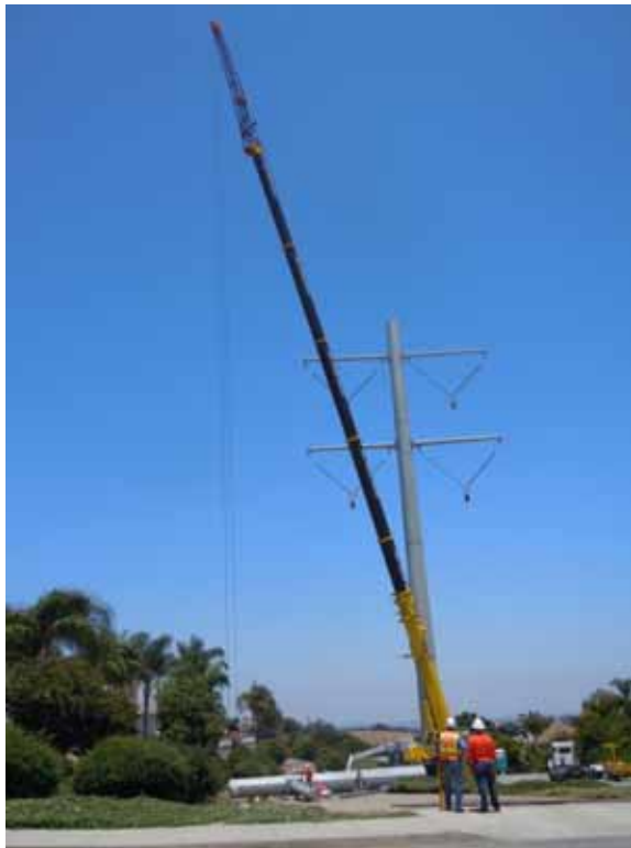
Figure 5: Crews erect a TSP in Chino Hills, Segment 8 Phase 1.
