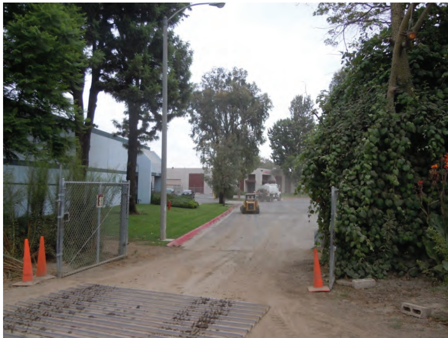
Figure 8: A Wilson employee sweeps Pellisier Place to remove trackout, Segment 8 Phase 4
