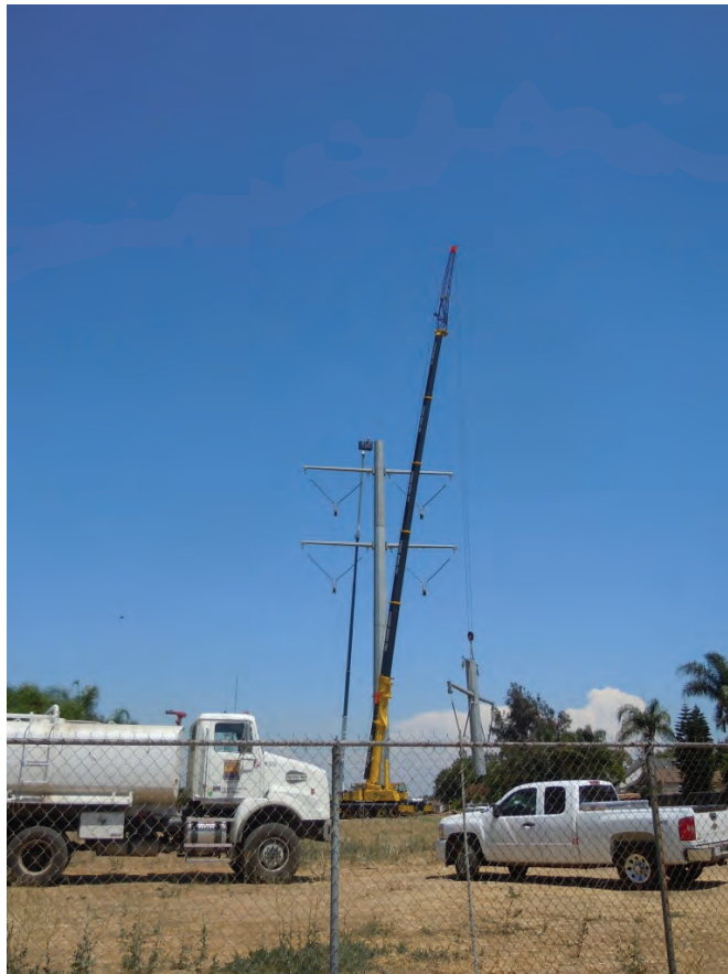
Figure 6: A crew sets a TSP within Chino Hills, Segment 8 Phase 1.
