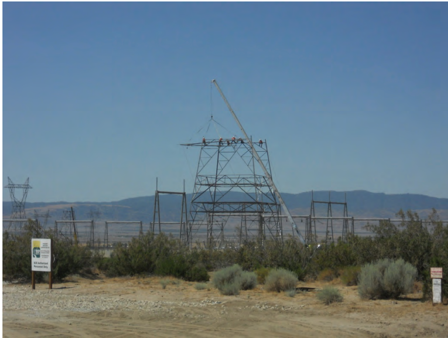
Figure 2: H&M steel crew erecting Tower 91 (just outside Whirlwind Substation), Segment 10.
