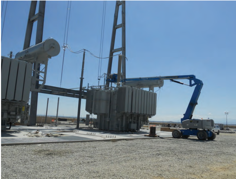
Figure 1: Conductor pulling into the transformers inside the Antelope Substation, Segments 1-3.
