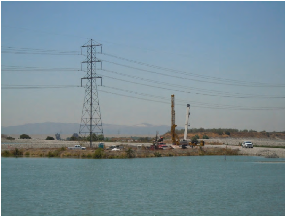
Figure 5: A Tri-State crew drills a foundation within USACE land, Segment 7.
