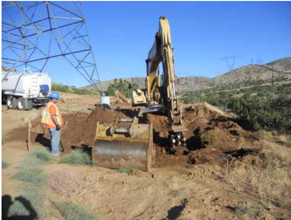
Figure 2: H&H Grading backfilling 220 kV foundation removal area near Tower 58, Segment 5.
