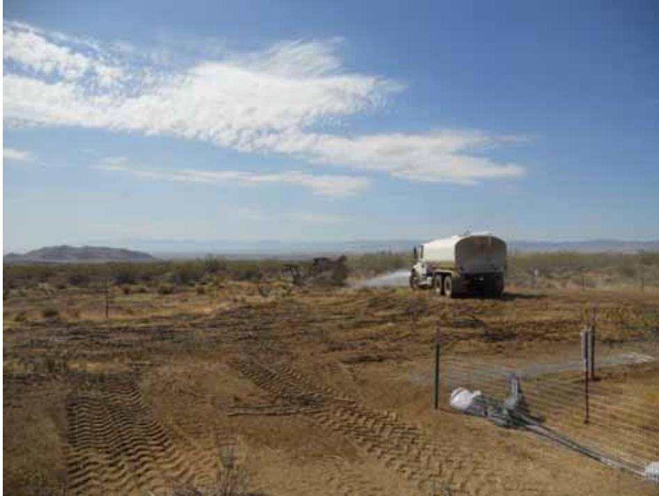
Figure 5: Water truck spraying behind the chipper at Tower 50 (after chipping had commenced), Segment 10.
