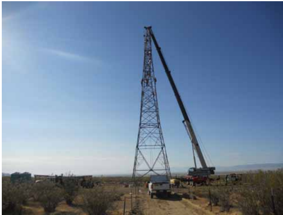
Figure 3: H&M steel crew erecting Tower 71, Segment 10.
