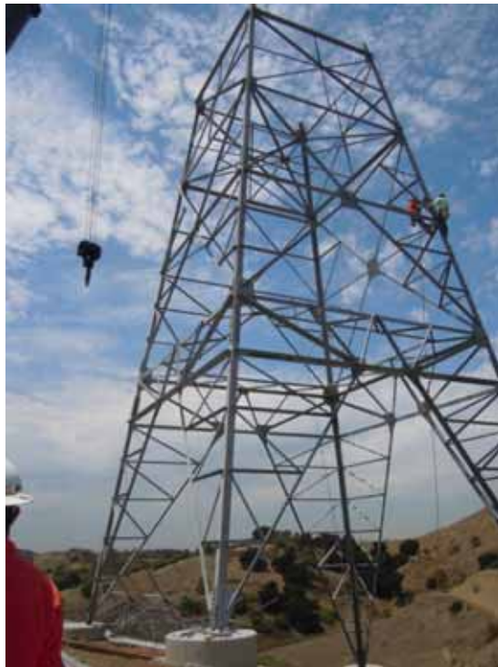
Figure 8: A crew assembles a TSP within Chino Hills, Segment 8 Phase 1.
