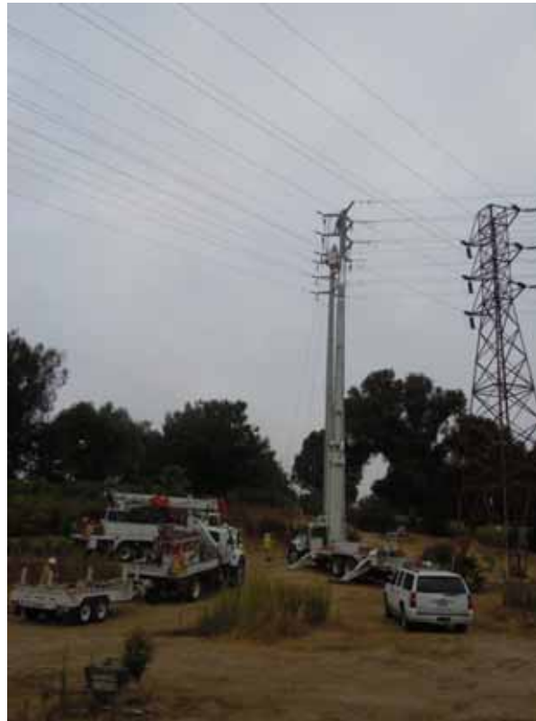
Figure 6: SCE crews string wire on various 66 kV circuits, Segment 7.
