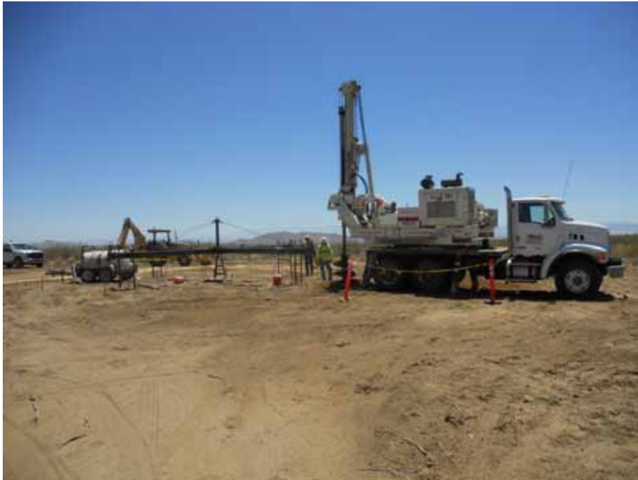
Figure 1: KV Structures drilling Tower 47, Segment 10.
