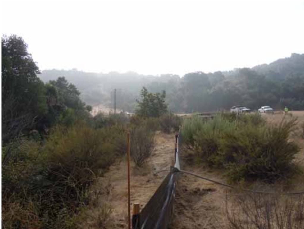
Figure 10: Conductor removed across the I-57 freeway sits atop the bank of Brea Creek, Segment 8 Phase 1.
