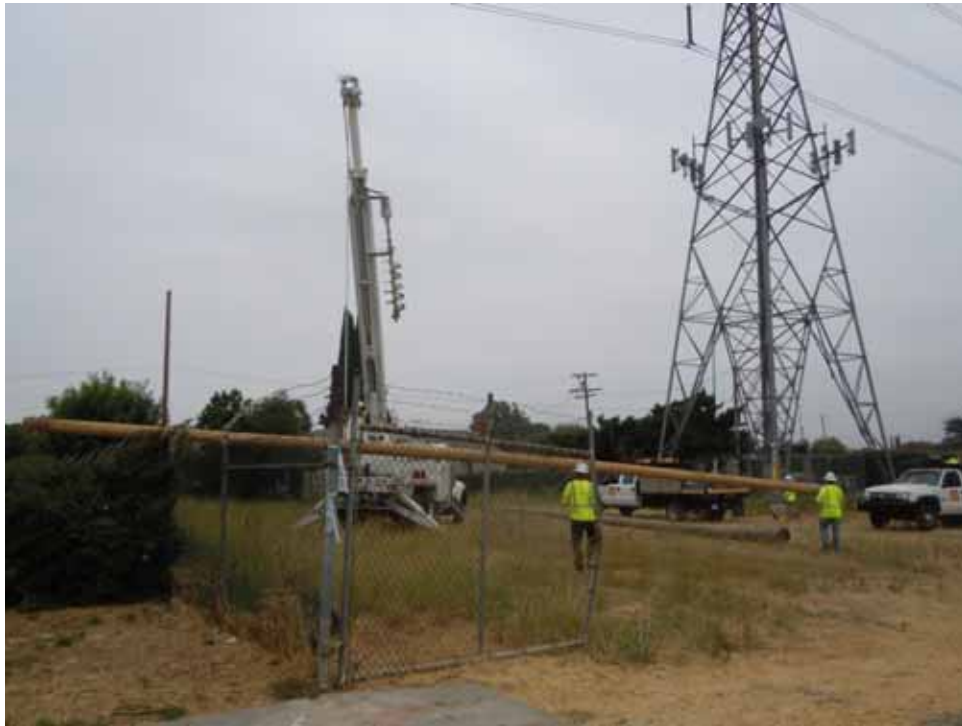
Figure 5: Crews prepare to install a guard pole site, Segment 11A.
