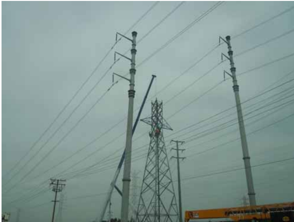
Figure 7: Crews assemble a tower at the I-605 Shoofly, Segment 8 Phase 4
