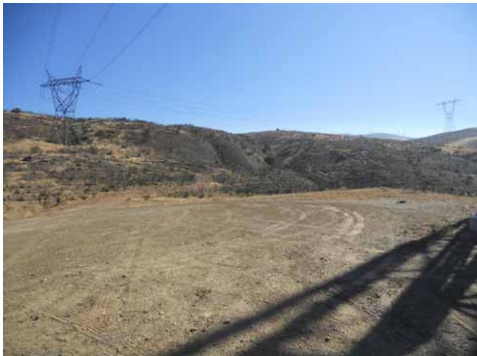
Figure 4: An approved TEWS area adjacent to Tower 30, Segment 5.
