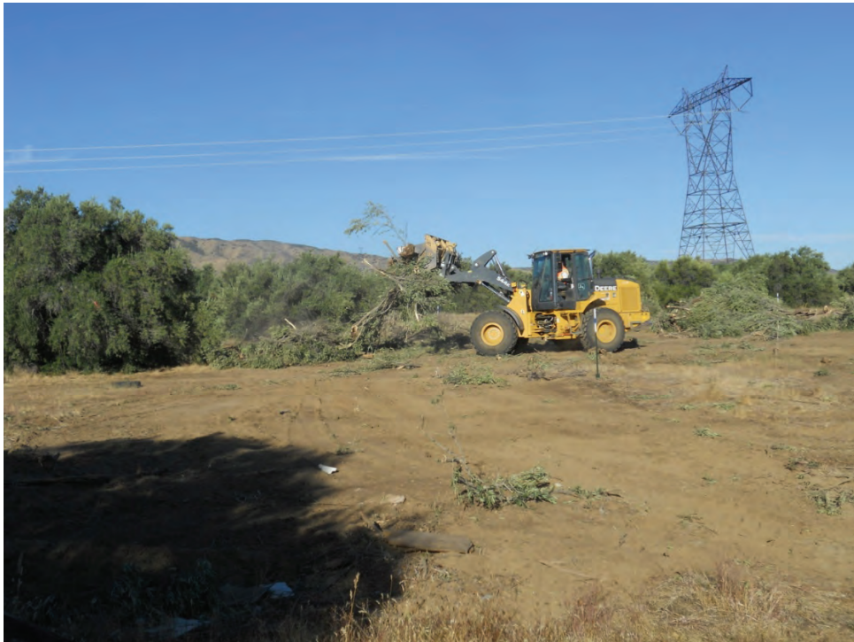
Figure 4: Olive tree removal near Towers 8 and M90-T1X, Segment 5.
