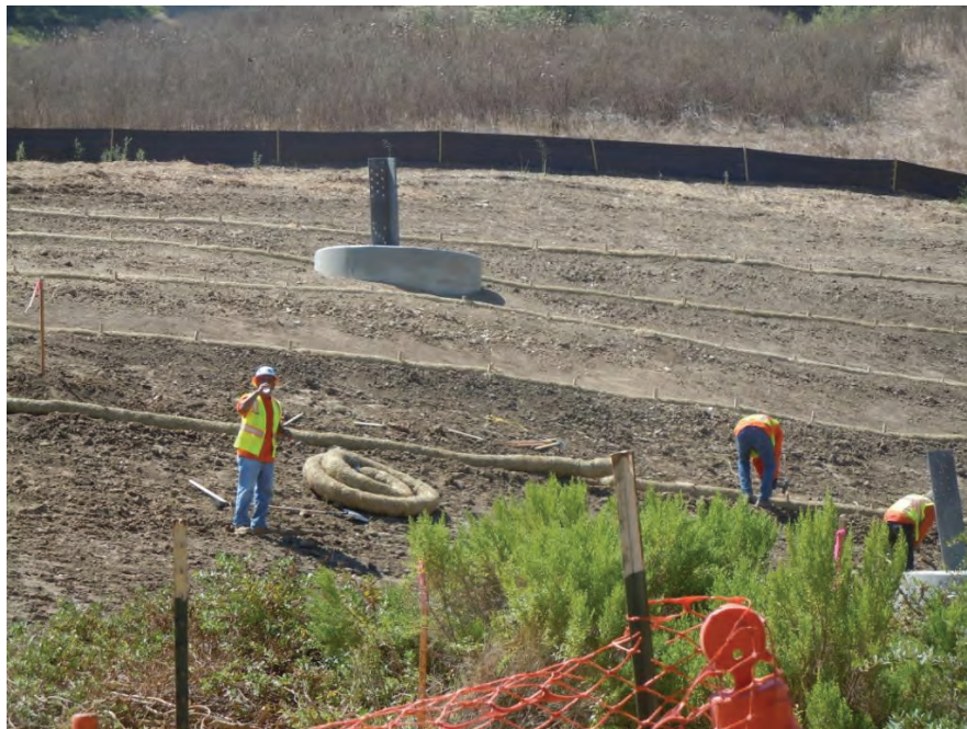
Figure 8: DCX crews install erosion control BMPs, Segment 8 Phase 1.
