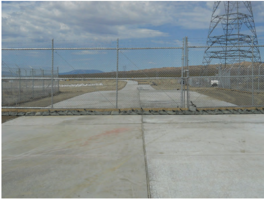
Figure 3: Concrete driveway at main gate to Whirlwind Substation, Segment 9.
