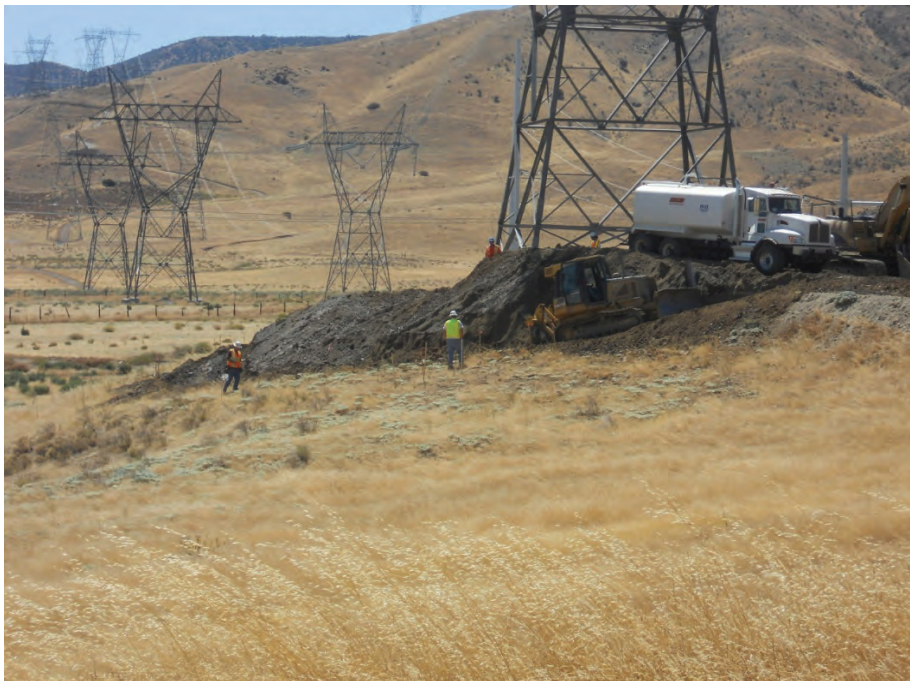
Figure 2: H&H grading the new access road at Tower 37, Segment 5.
