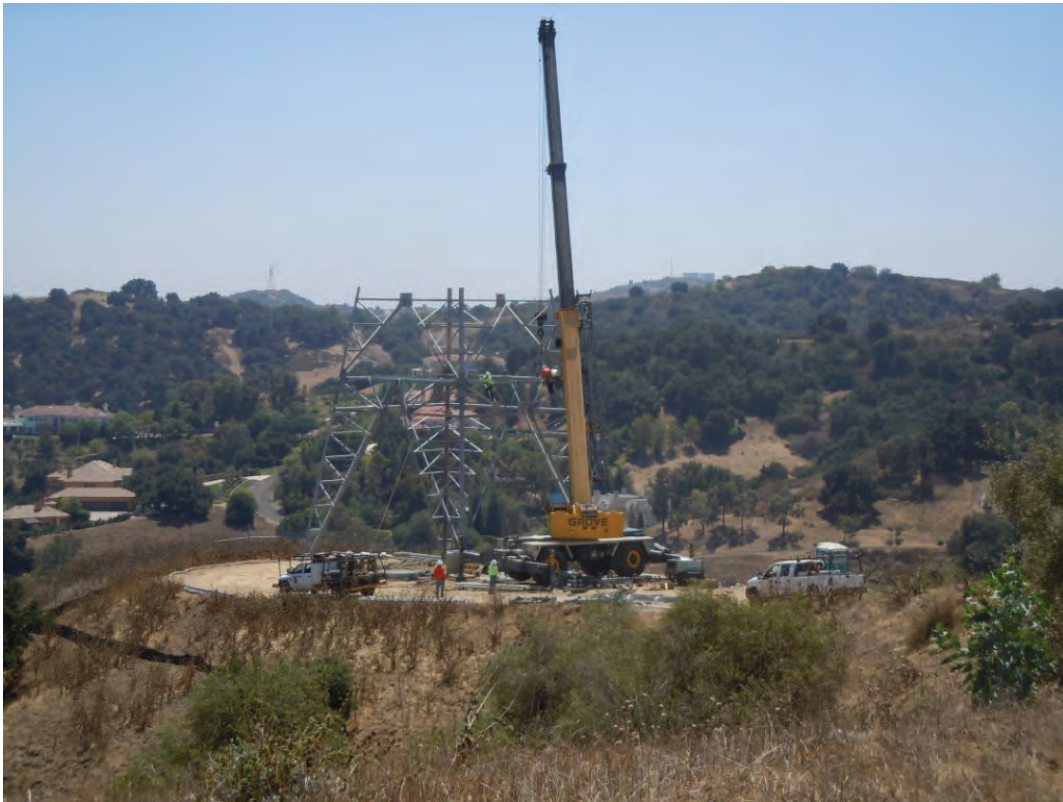
Figure 7: A Wilson crews assembles a tower, Segment 8 Phase 1.
