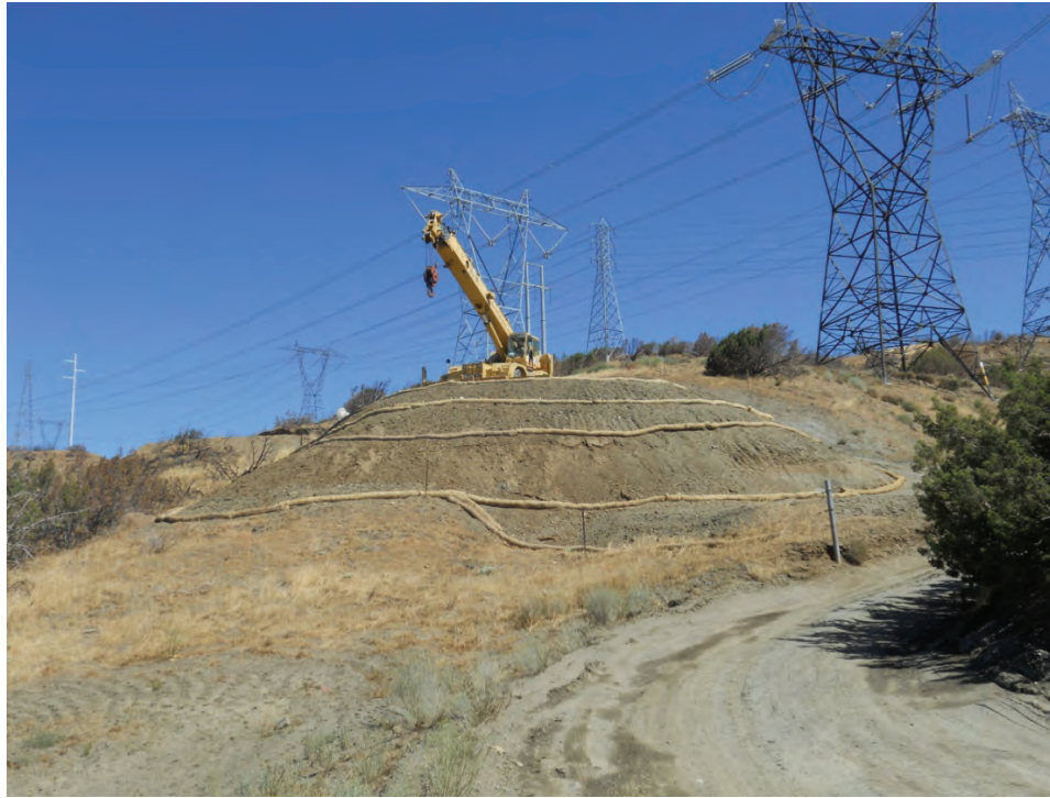
Figure 1: Crane pad site for Tower 28A with fiber roll BMP's, Segment 5.
