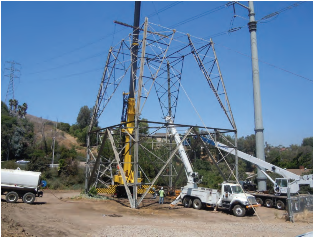
Figure 9: A Wilson crew removes a tower within Fullerton Yard, Segment 8, Phase 4.
