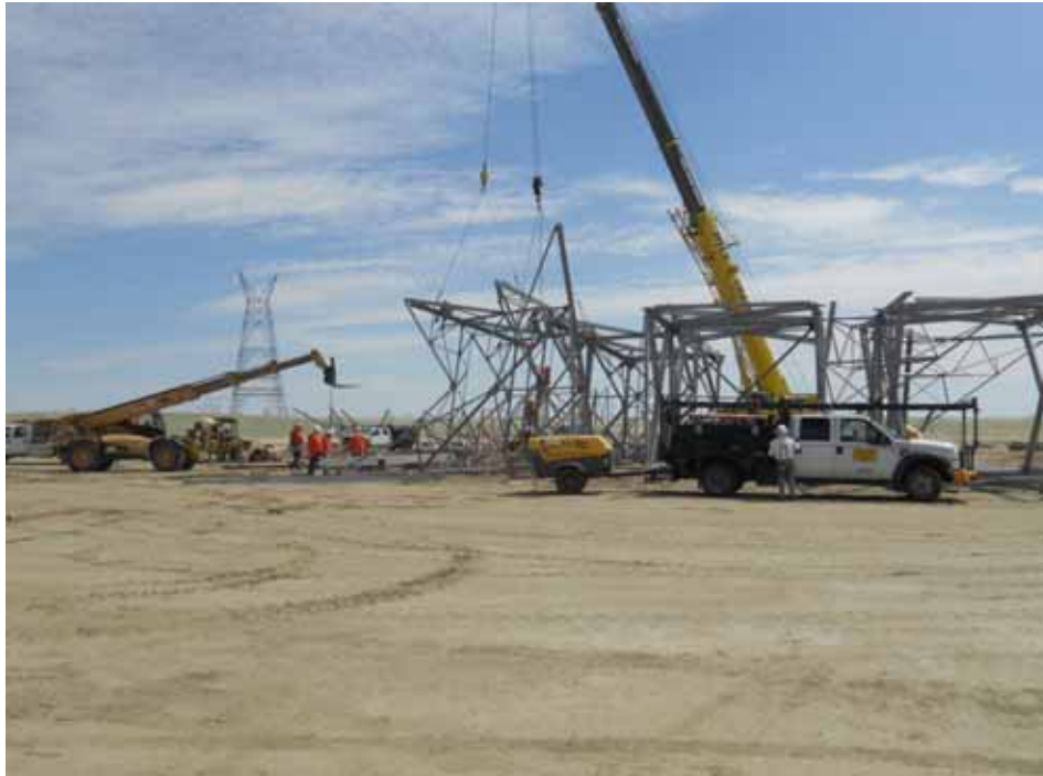
Figure 1: H&M steel crew assembling Tower 92 inside Whirlwind Substation, Segment 10.
