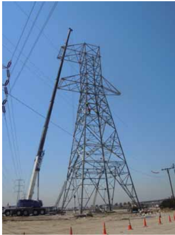
Figure 7: A Wilson crew assembles a tower, Segment 7.
