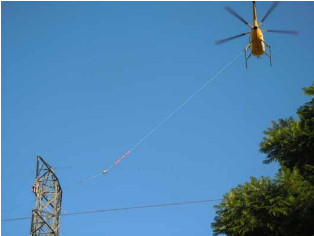
Figure 6: A helicopter pulls sockline through a traveler, Segment 11A.
