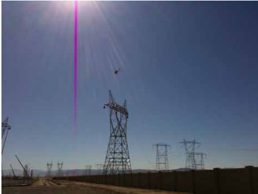
Figure 1: Helicopter being used for wire stringing preparation on Tower M73-T3B, Segment 4.
