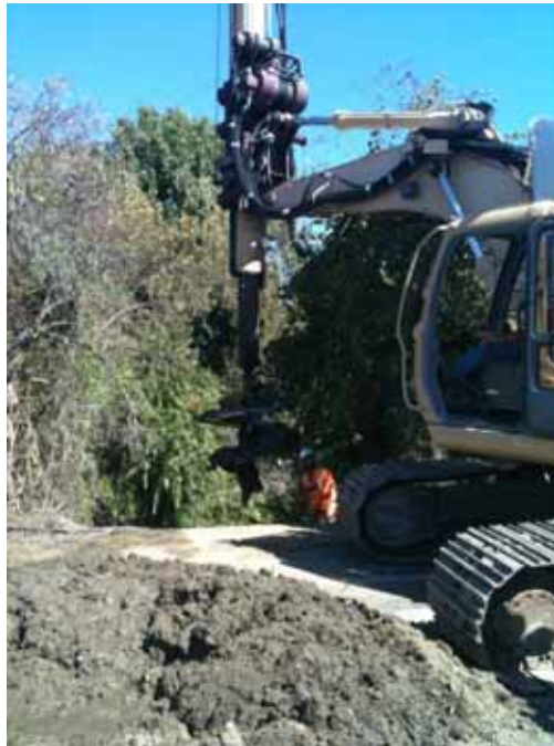
Figure 6: Foundation drilling along San Gabriel Boulevard with spill pile, Segment 8.
