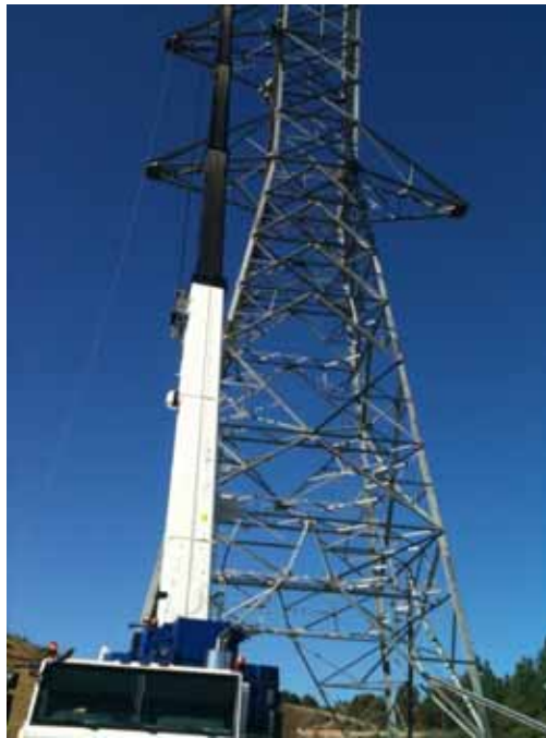
Figure 10: Crews assemble a tower within Chino Hills, Segment 8 Phase 1.
