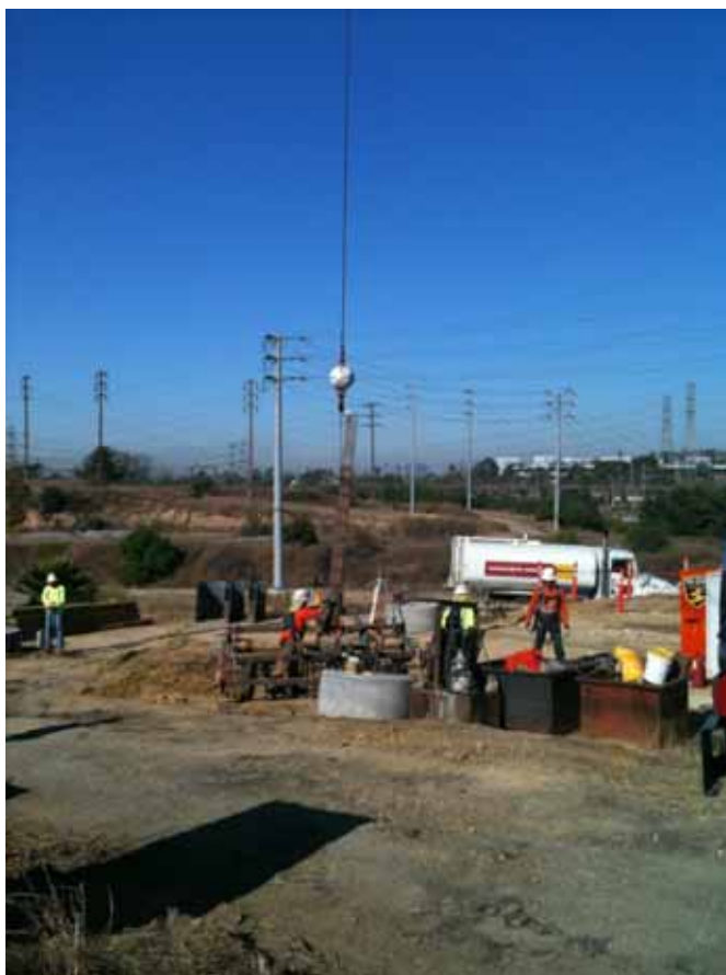
Figure 8: Crews lower a stub angle into a foundation, Segment 7.
