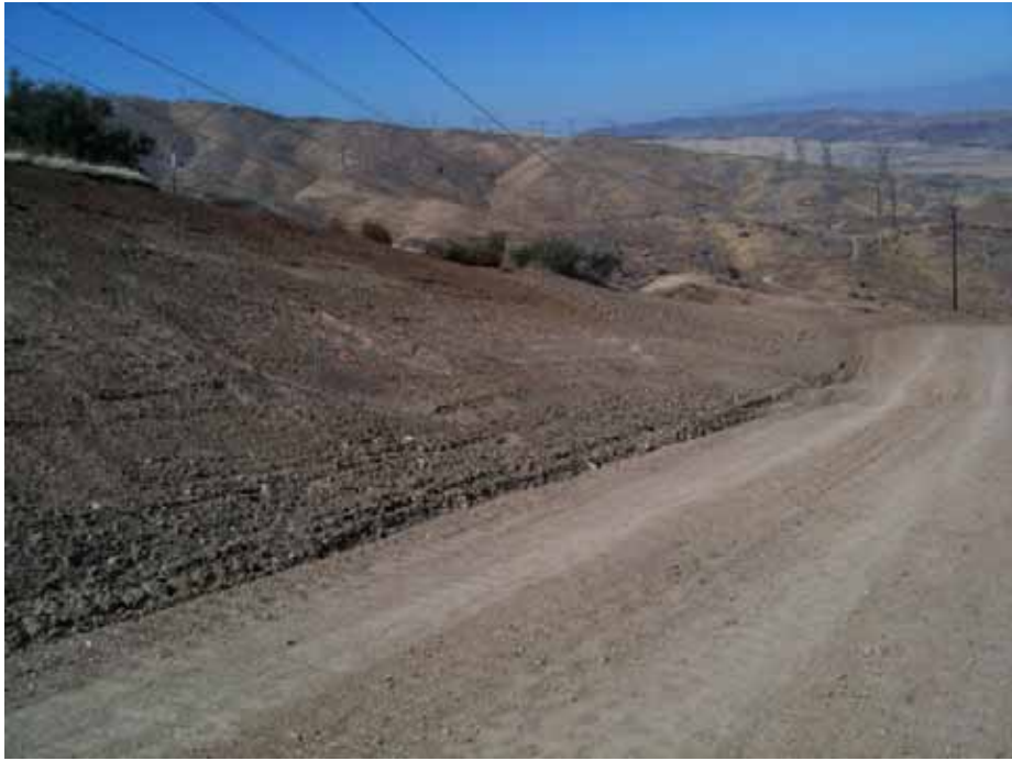
Figure 5: Disturbance area near Tower 49 that lacks BMP's (i.e. fiber rolls), Segment 5.
