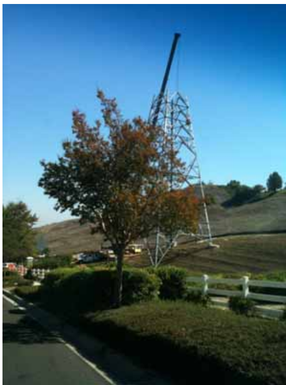
Figure 11: Crews assemble a tower within Chino Hills, Segment 8 Phase 1.
