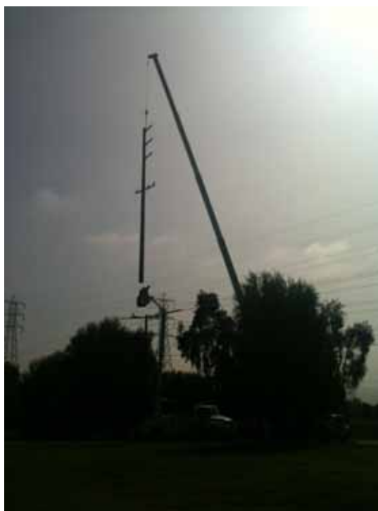
Figure 7: Crews set a lightweight steel pole, Segment 7 66 kV.
