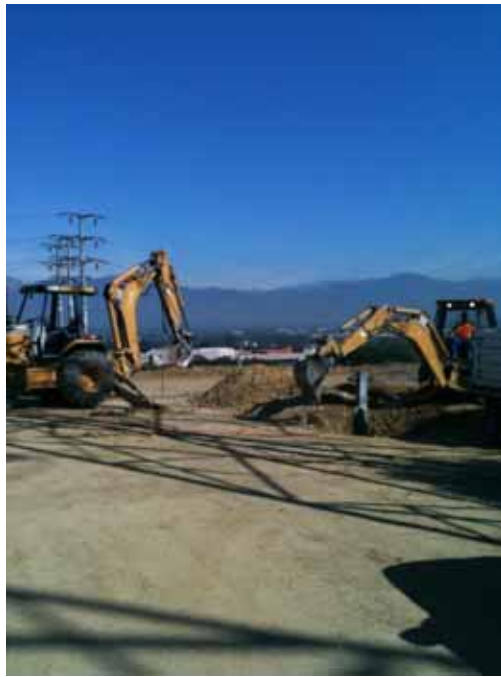
Figure 9: Foundation demolition within Montebello Hills, Segment 7.
