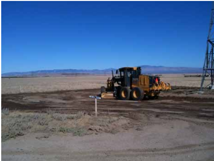
Figure 2: H&H Grading re-contoured Tower 52 disturbance site, Segment 4.
