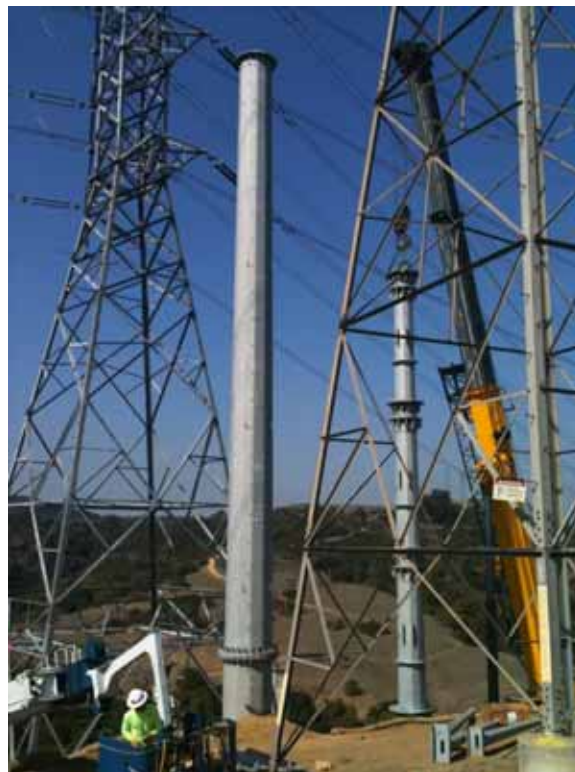
Figure 6: Crews dismantle a shoofly pole, Segment 8.
