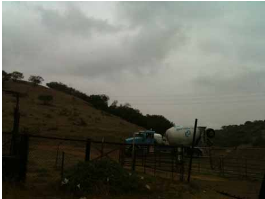
Figure 7: A concrete truck parked outside of an approved access road, Segment 8.
