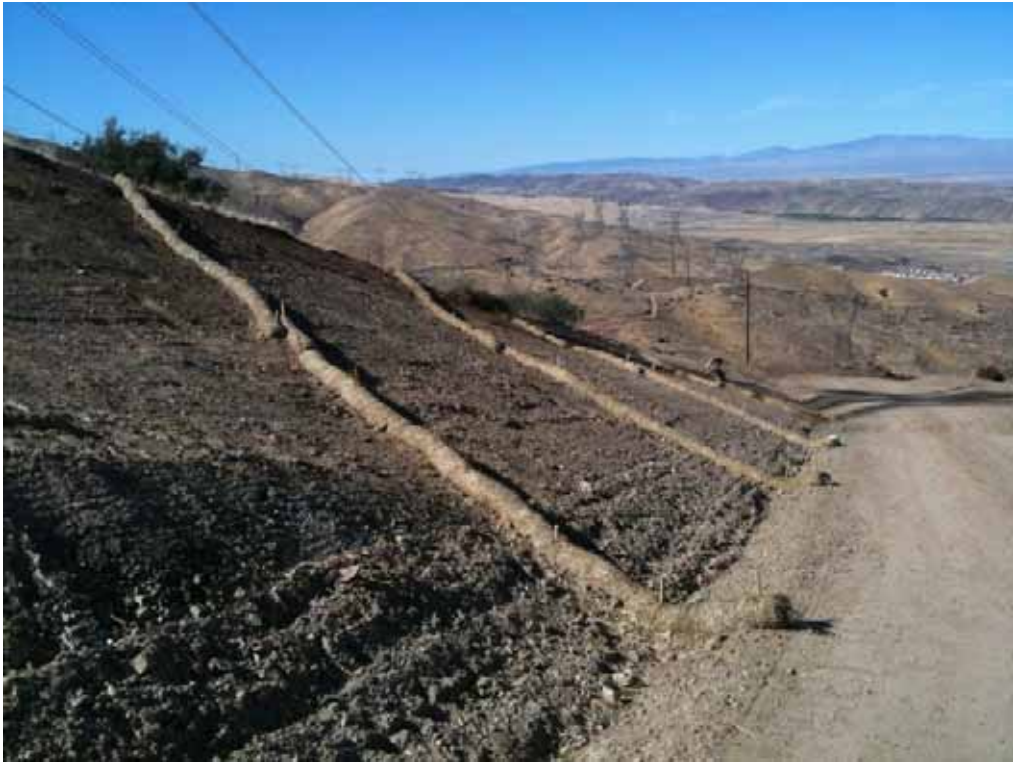
Figure 3: Fiber rolls installed in the disturbance area near Tower 49, Segment 5.
