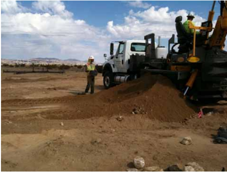
Figure 1: Paleontological monitor onsite during foundation drilling of Tower 29, Segment 10.
