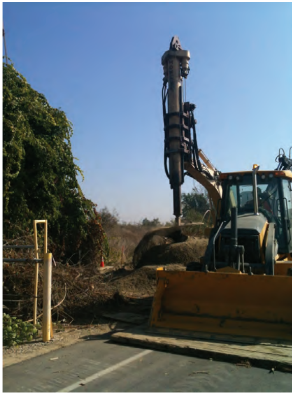
Figure 5: Foundation drilling along Siphon Road in Whittier Narrows, Segment 8 66 kV.
