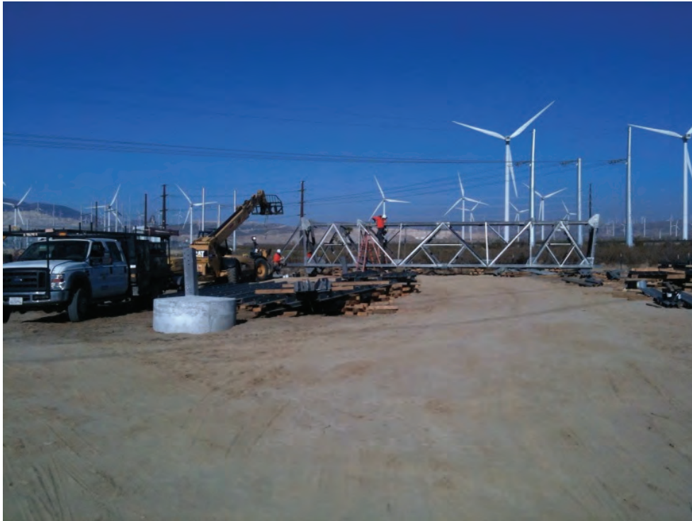
Figure 1: H&M steel crew assembling Tower 8, Segment 10.
