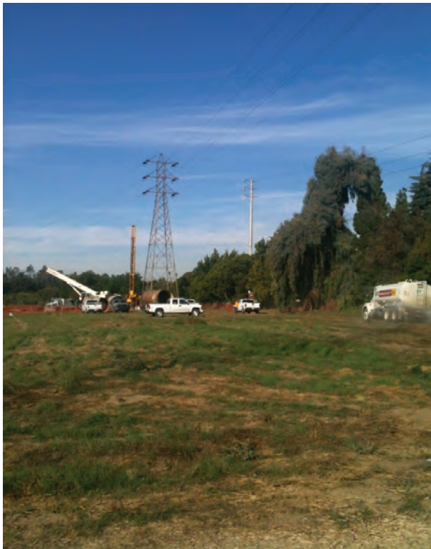
Figure 6: Foundation drilling at M40-T2 with watering for fugitive dust, Segment 7.
