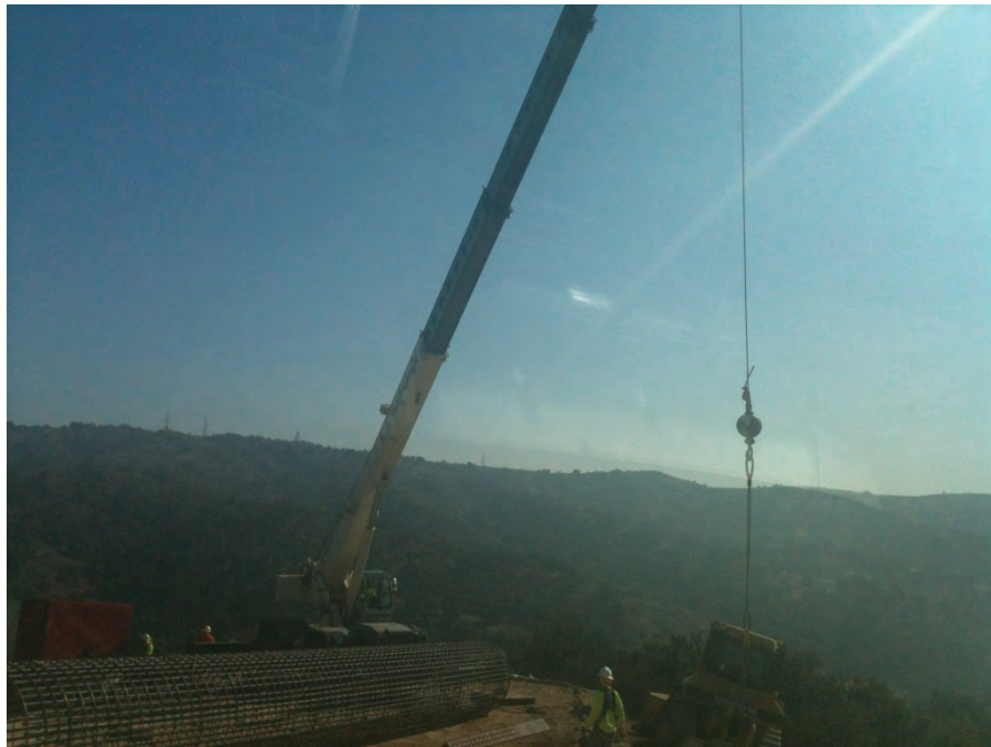
Figure 7: Tri-State crews prepare a rebar cage in Tonner Canyon, Segment 8 Phase 1.
