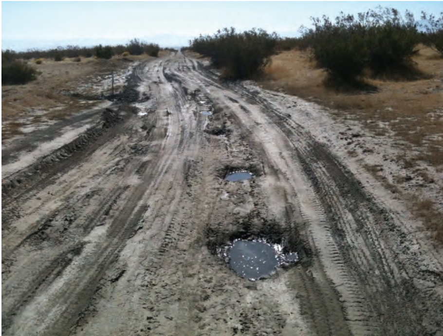
Figure 4: Potholes along 160 th road in desert tortoise habitat, Segment 10.
