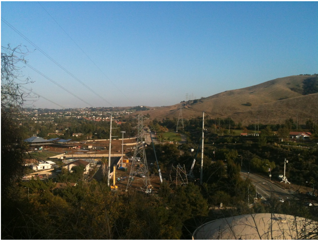
Figure 5: Wilson crews transfer conductor at the Fullerton Shoofly, Segment 8 Phase 4.
