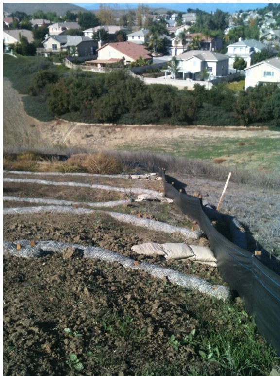
Figure 6: Fiber rolls and silt fencing after a rain event, Segment 8 Phase 1.
