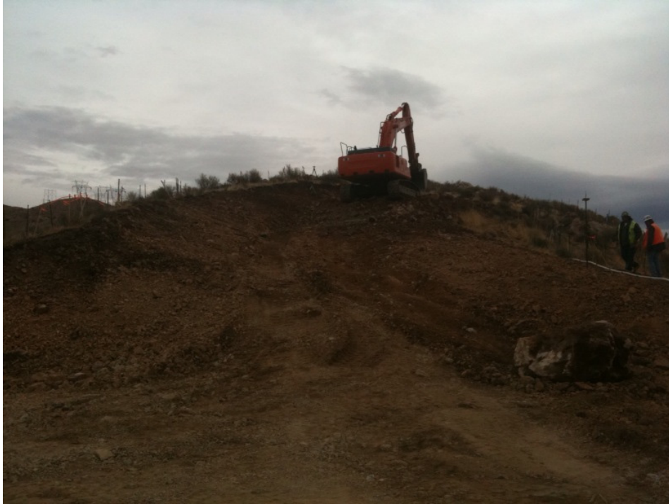
Figure 1: Cattracts grading Tower 68, Segment 5.
