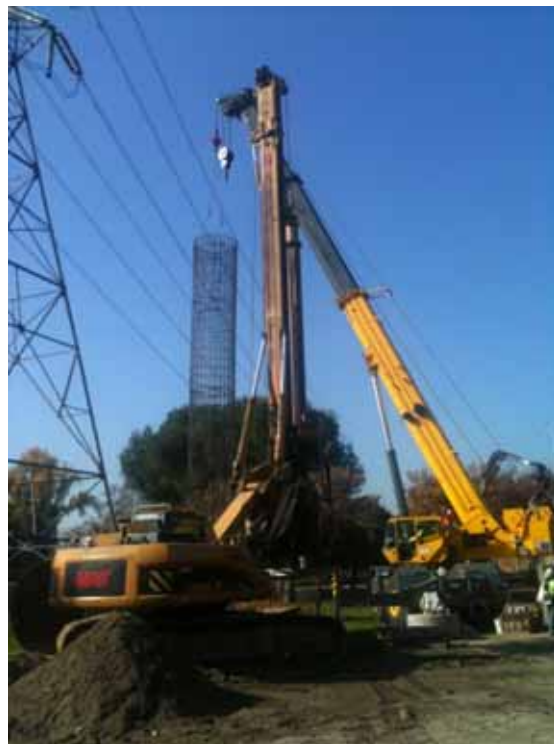
Figure 8: Crews load a rebar cage at M39-T4, Segment 7.
