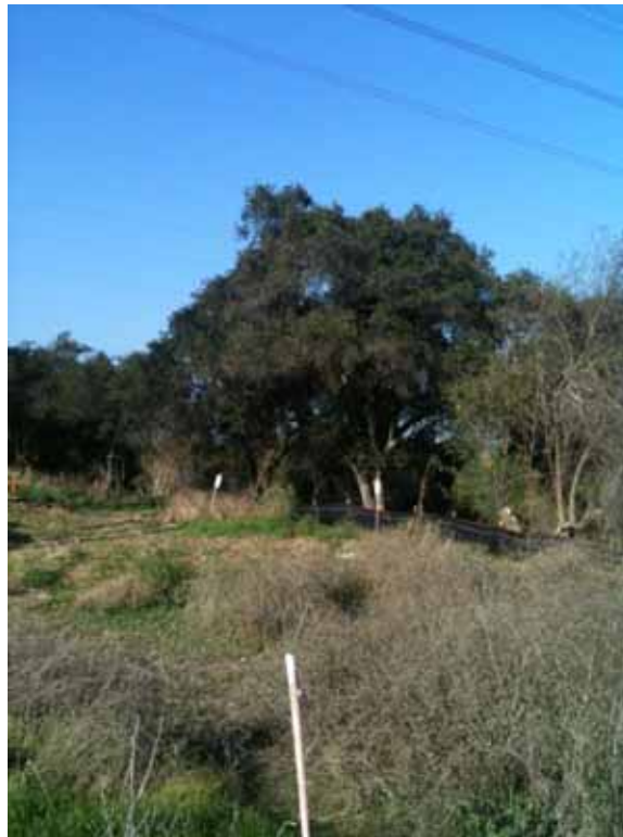
Figure 10: A silt fence at San Gabriel Junction inside the dripline of an oak tree.
