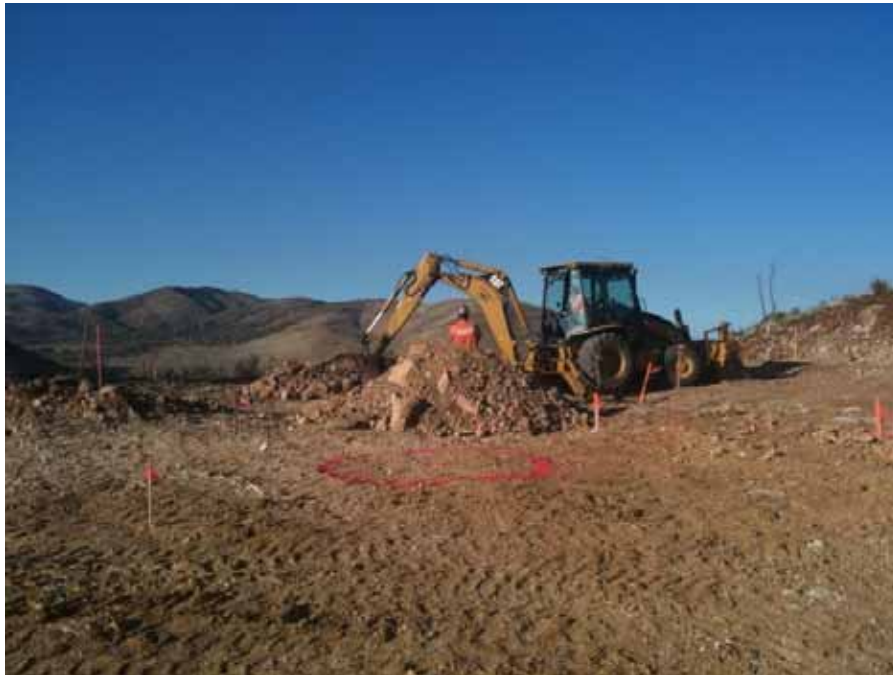
Figure 3: Crux conducting preliminary digging at Tower 68, Segment 5.
