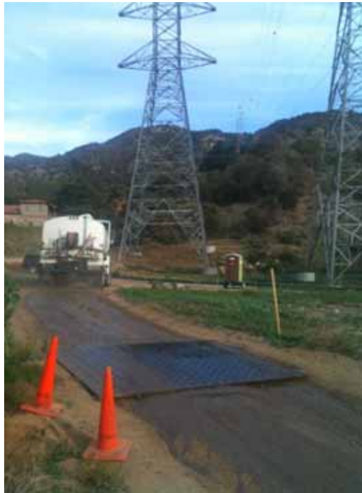
Figure 9: A water truck at Tower M54-Ta, Segment 7.
