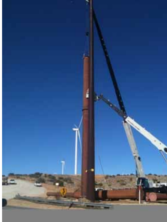
Figure 2: TSP erection along Oak Creek Road, Wilderness Line, Antelope Transmission Segment.
