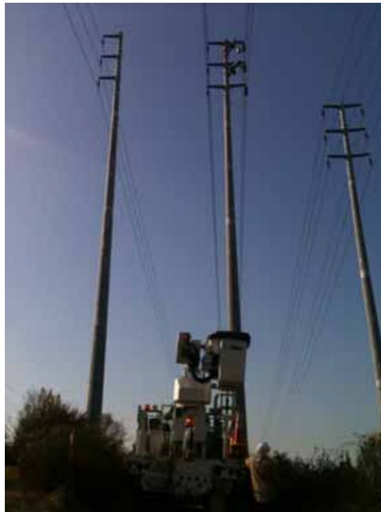
Figure 6: SCE crews install new insulators within Montebello Hills.
