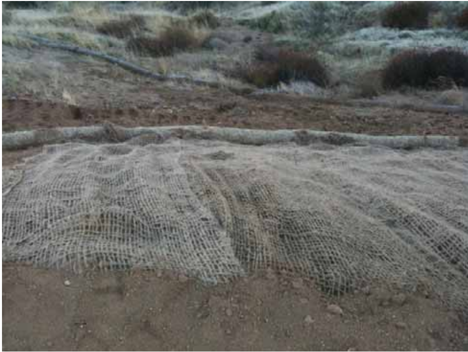
Figure 5: BMP repair at Tower 50 (jute netting was installed), Segment 5.
