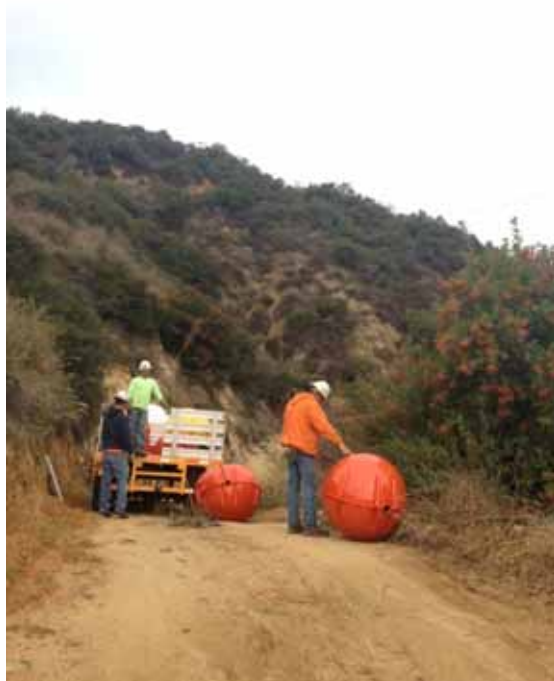
Figure 7: Crews unload marker balls to be hung on Segment 7 spans.
