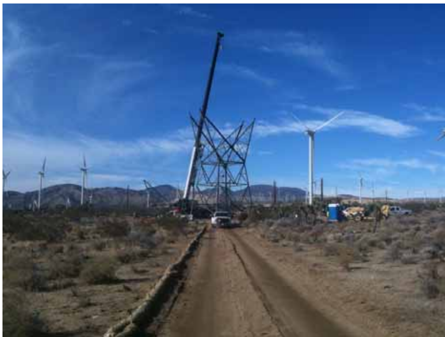
Figure 4: H&M steel crew erecting Tower 3, Segment 10.
