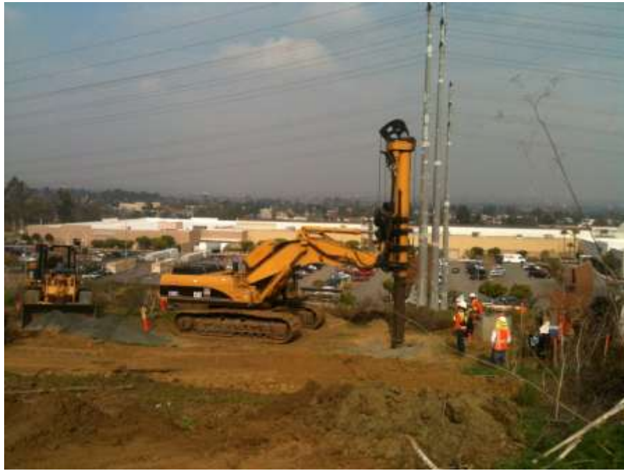
Figure 5: Crews drill a foundation within Montebello Hills, Segment 7.
