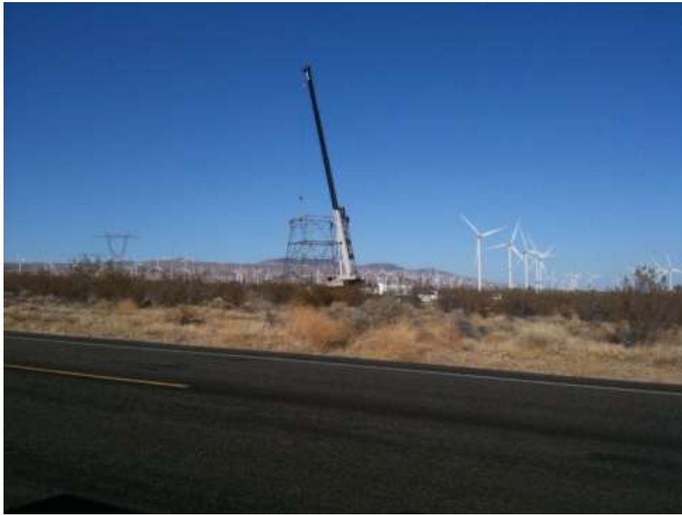
Figure 3: H&M steel crew erecting Tower 25, Segment 10.
