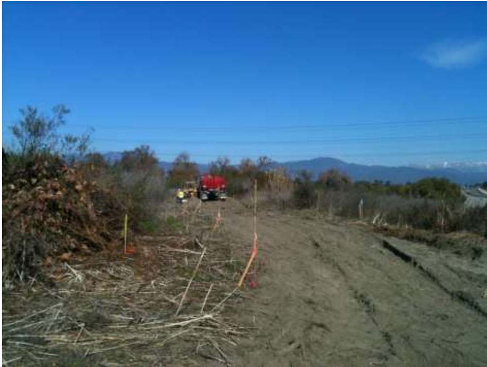
Figure 4: A water truck waters a newly bladed access road, Segment 8, 66 kV.
