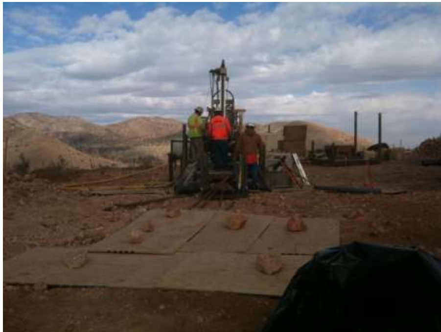
Figure 2: Crux micro-pile drilling at Tower 68, Segment 5.
