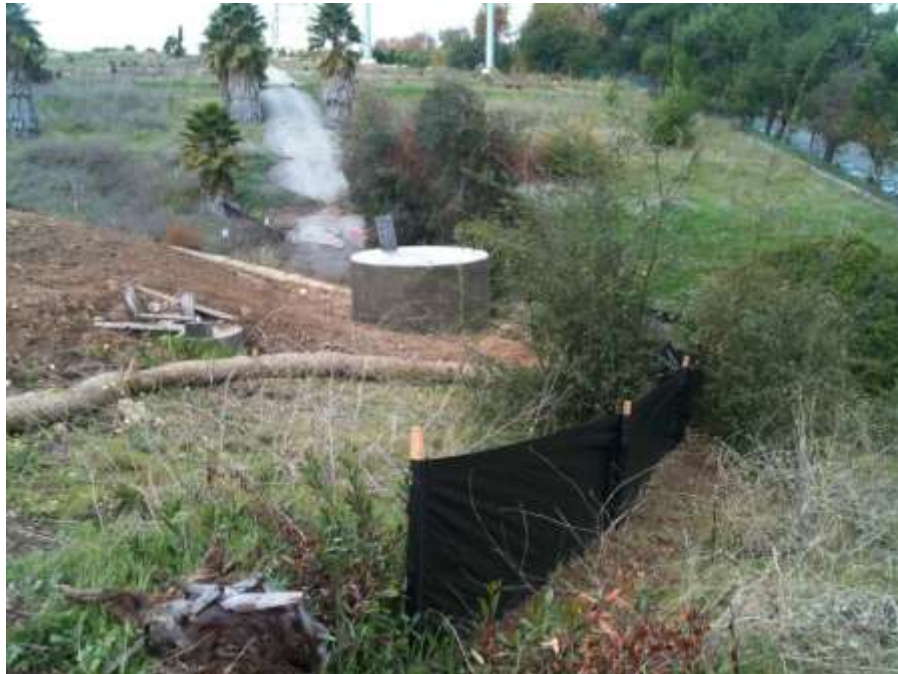
Figure 6: BMPs surrounding a foundation leg, Segment 7.
