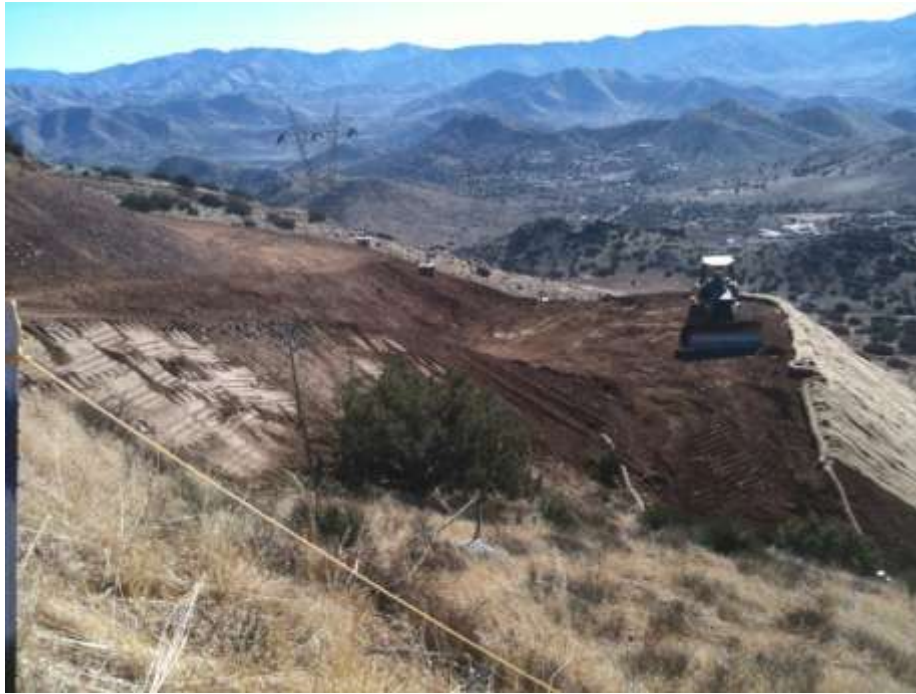
Figure 1: Completed foundation work at Tower 55A, Segment 5.
