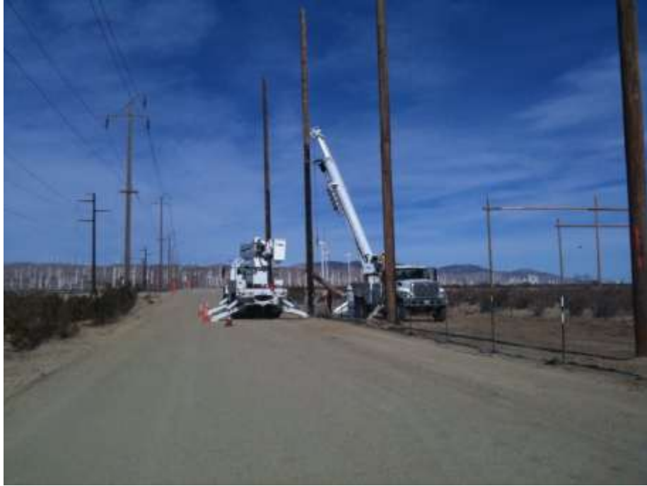
Figure 3: H&M crew installing guard poles between Towers 7 and 8, Segment 10.
