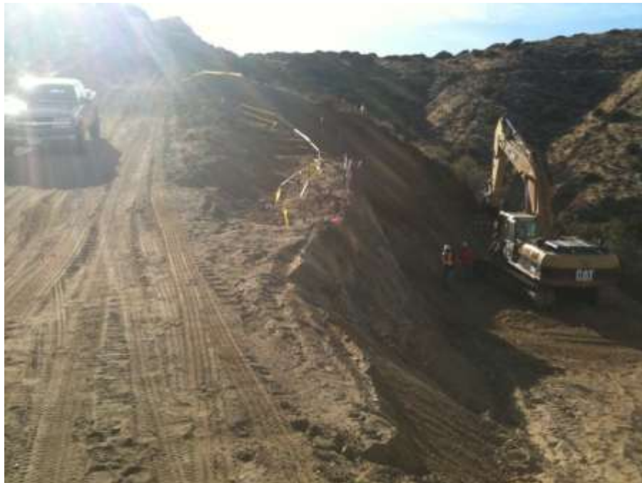
Figure 2: Cattracs grading at Tower 19 for slope stabilization, Segment 5.
