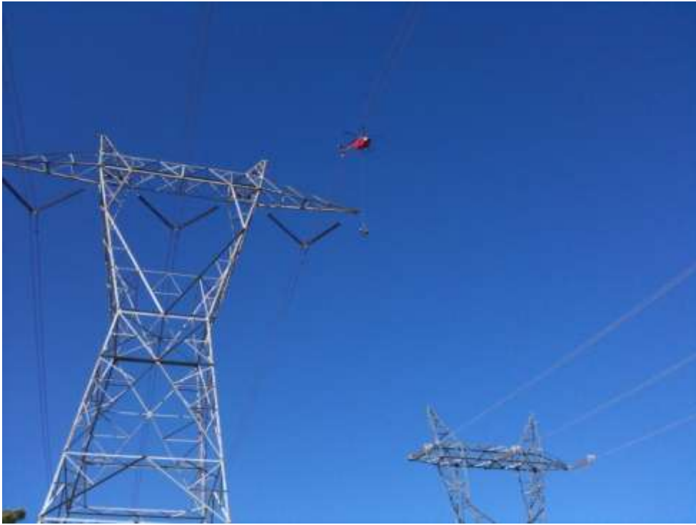
Figure 1: Helicopter use during wire stringing activity between Towers 57 and 63, Segment 5.
