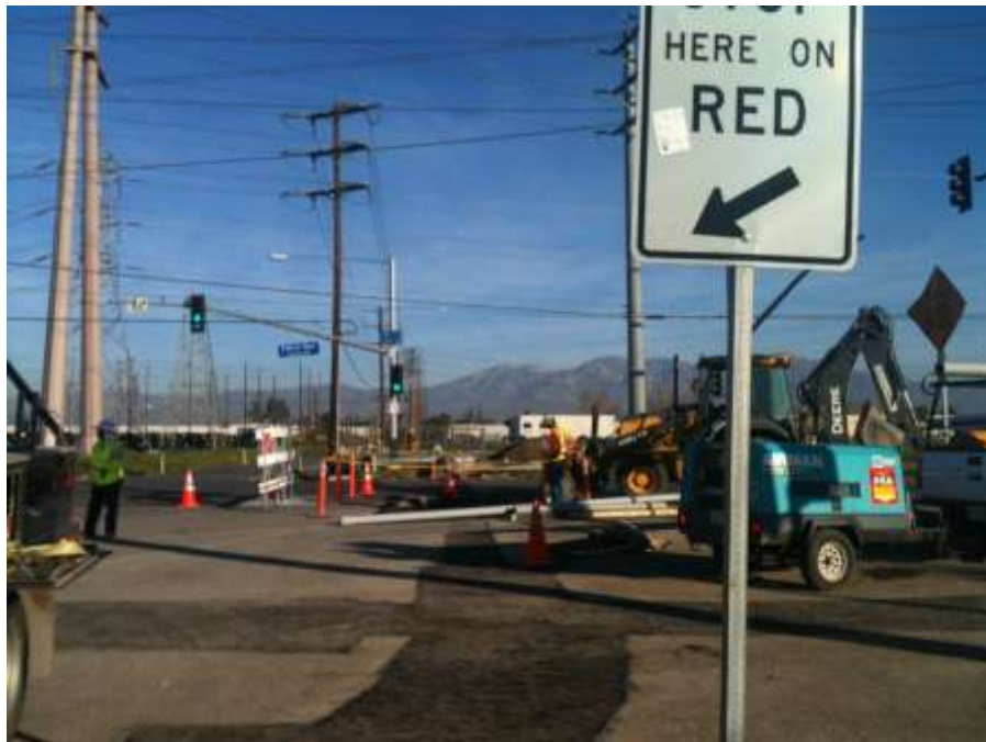
Figure 4: Crews install conduit across Edison Avenue, Segment 8, 66 kV.
