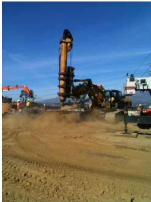
Figure 6: Crews drill a foundation hole within Montebello Hills, Segment 7.
