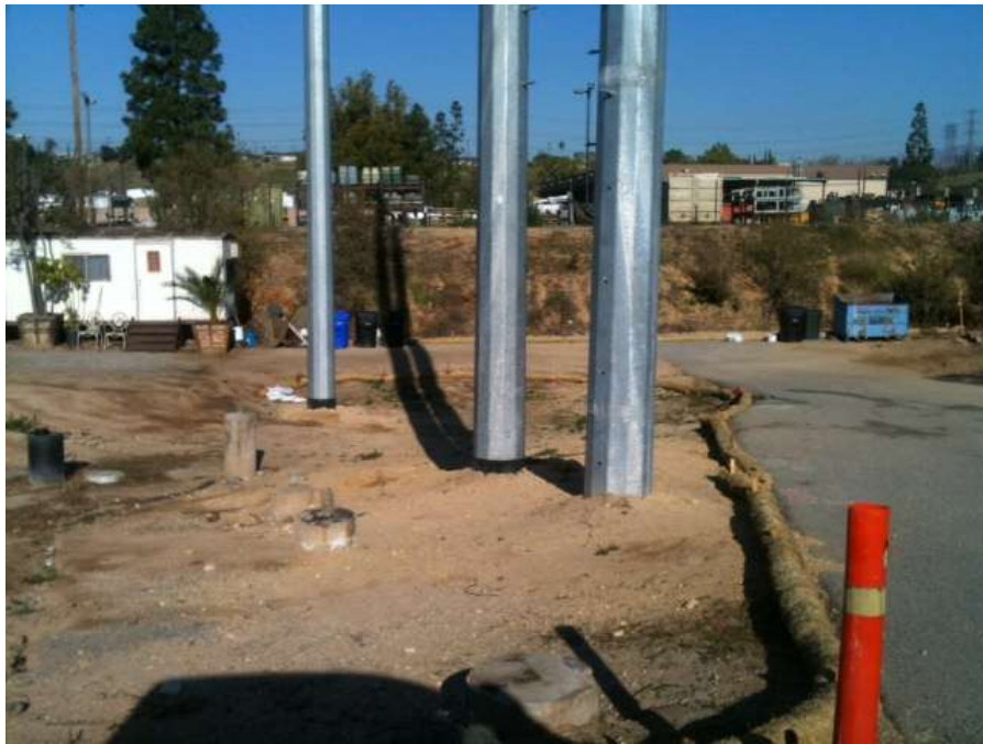
Figure 6: Newly installed fiber rolls, Segment 7.
