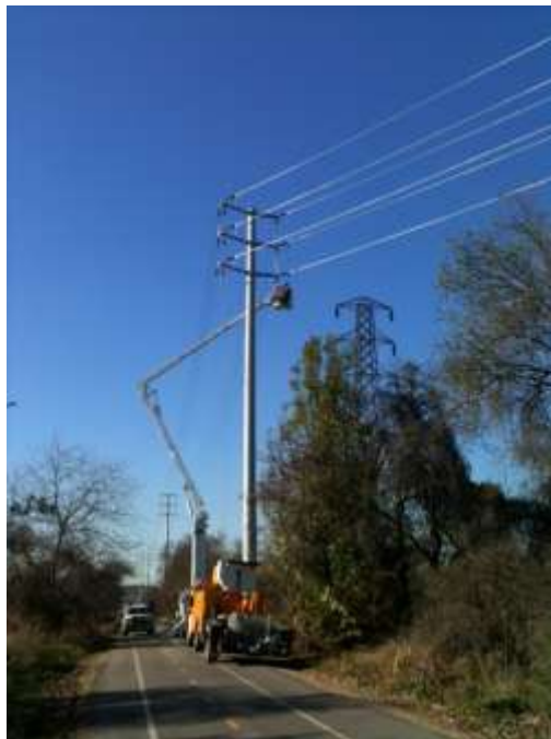
Figure 4: Crews install conductor along Siphon Road, Segment 8 66 kV.
