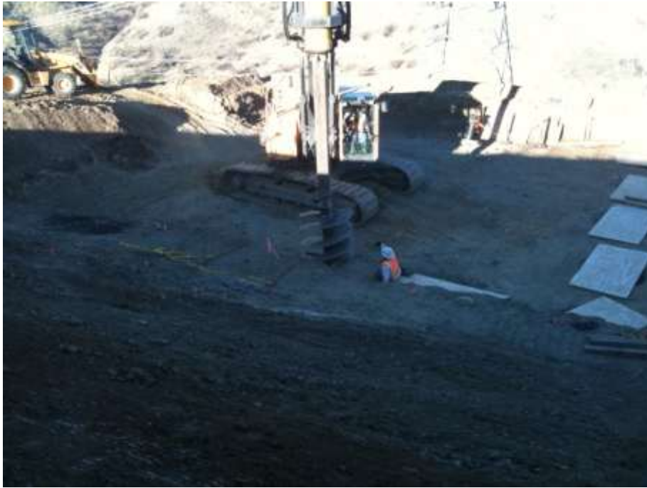
Figure 1: kV Structures drilling Tower 30, Segment 5.
