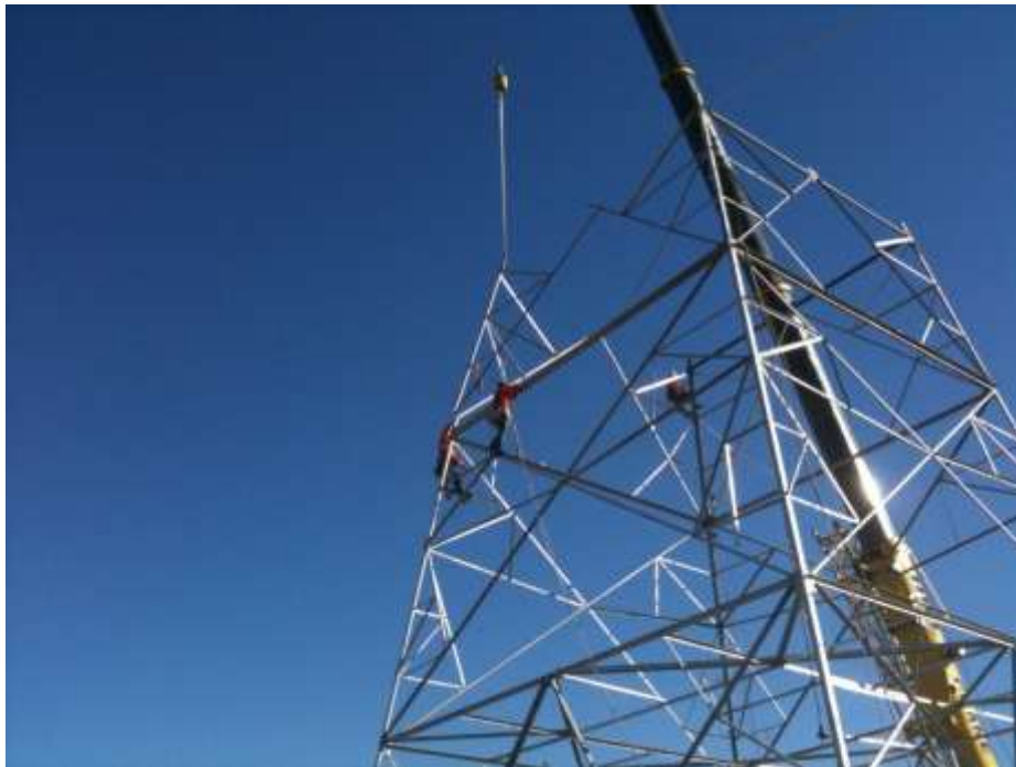
Figure 2: H&M steel crew erecting one of the last Segment 10 towers.
