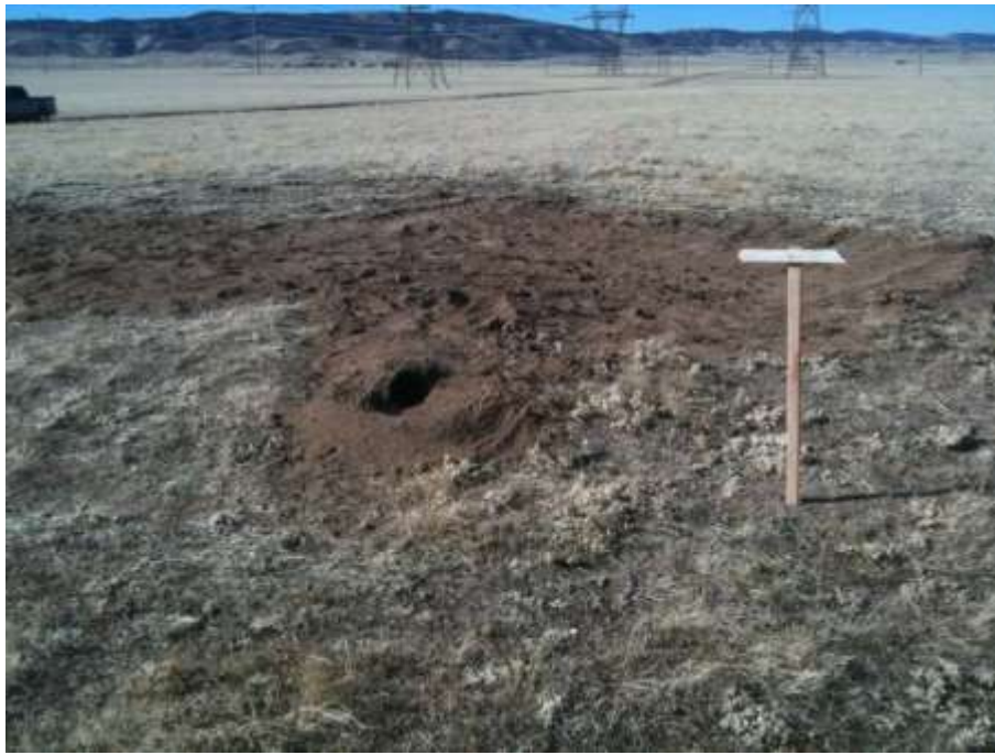
Figure 3: Artificial burrowing owl burrow construction, Segment 4.
