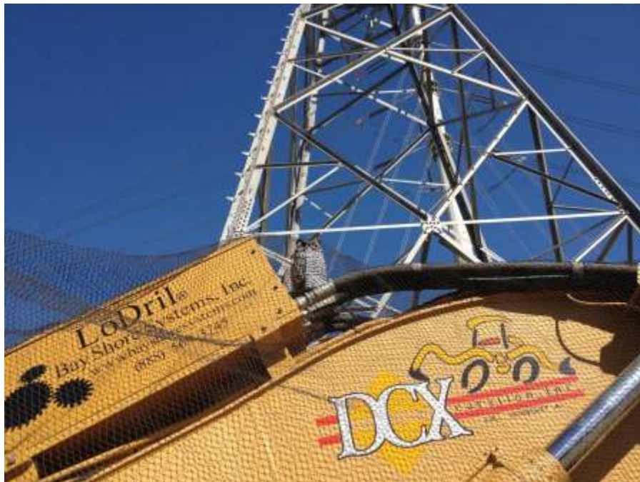
Figure 6: Bird netting and artificial owl deterrents, Segment 8 Phase 4.
