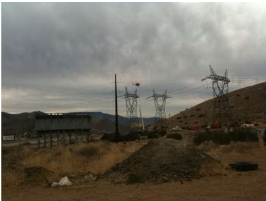
Figure 2: Wire work with a helicopter near Tower 65, Segment 5.
