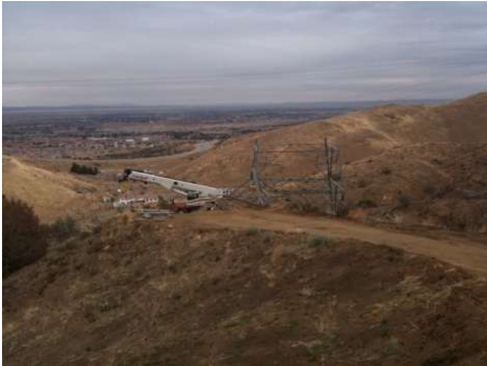
Figure 1: H&M steel crew assembling and erecting Tower 25, Segment 5.
