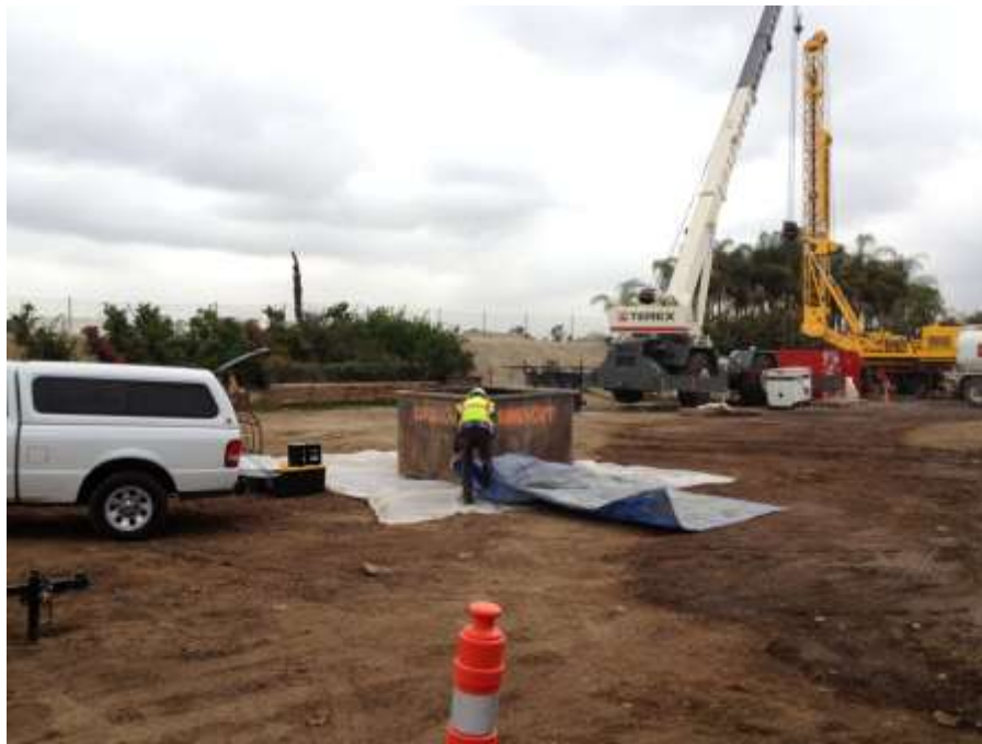
Figure 5: A concrete washout station being established during drilling operations, Segment 7.
