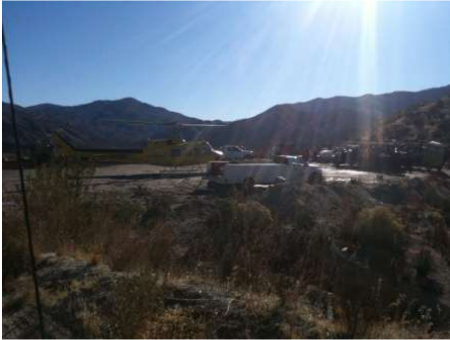
Figure 3: Wikiup helicopter landing zone for wire work, Segment 6B.
