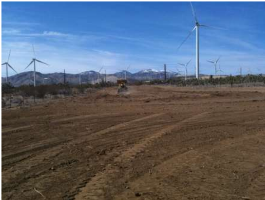
Figure 2: H&H Grading conducted site clean-up at WSS near Tower 3, Segment 10.
