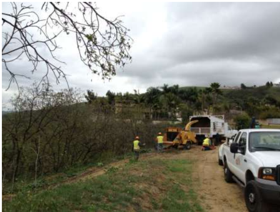
Figure 6: Tree removal at Tower MA1-T2 in Rowland Heights, Segment 8 Phase 4.
