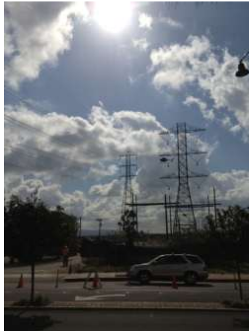
Figure 4: Helicopter stringing sockline and traffic control, Segment 7.
