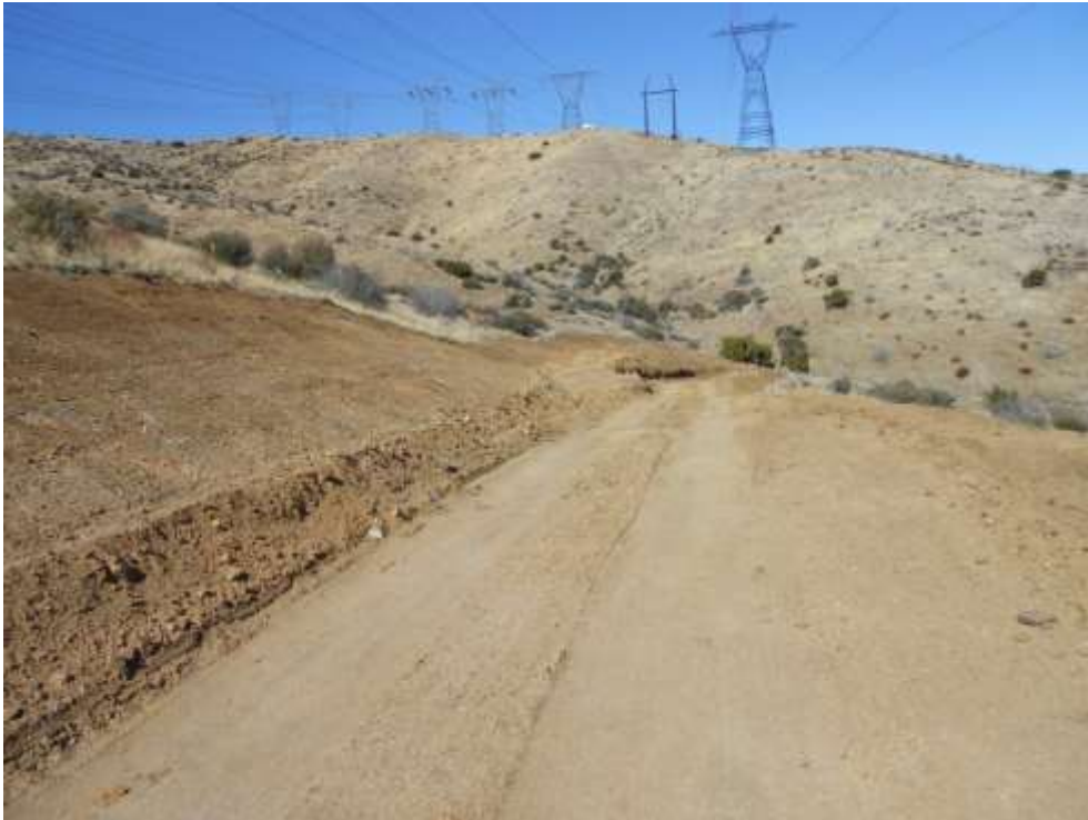
Figure 1: New access road to Midway-Vincent Upgrade Tower 86A, Segment 5.
