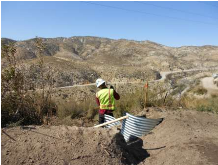
Figure 2: A crew member installs a roadside drain, Segment 6B.
