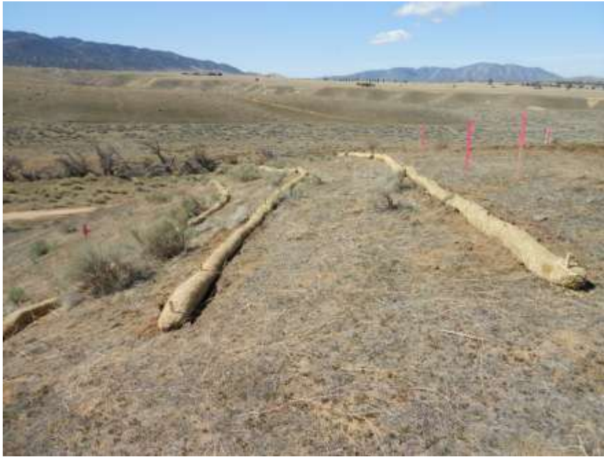
Figure 1: Straw wattle installation at Tower 7, Segment 3B.
