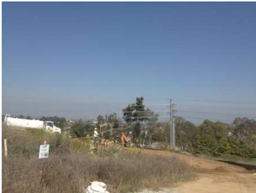
Figure 6: A crew member waters the pad at a tower site, Segment 7.
