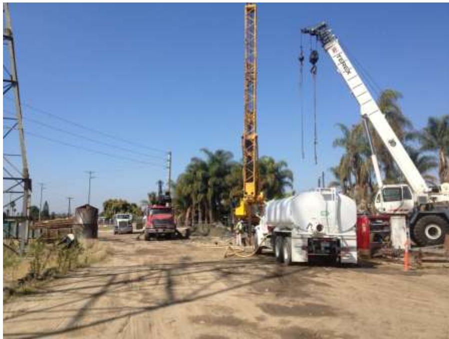
Figure 7: A crew member adds water to a foundation hole, Segment 7.
