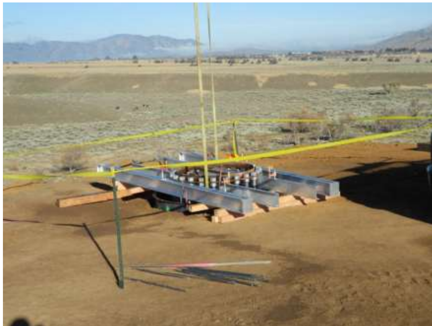
Figure 2: TSP foundation for Structure 7, Segment 3B.
