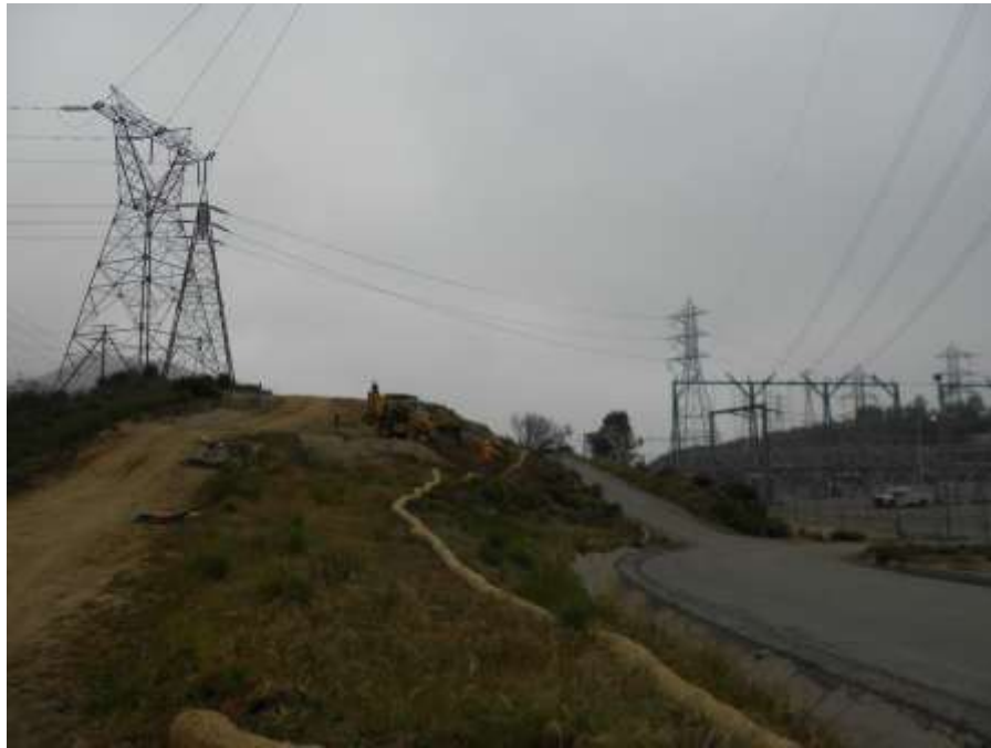
Figure 5: A crew repairs a hillside after erosion, Segment 11D.
