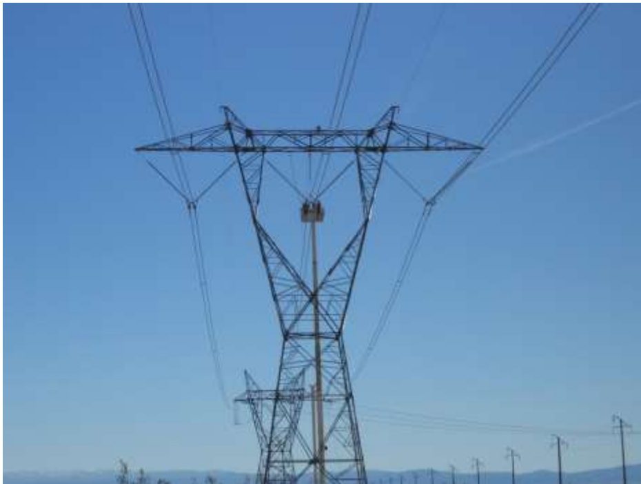
Figure 2: H&M wire crew adjusting insulators on Tower 42, Segment 10.
