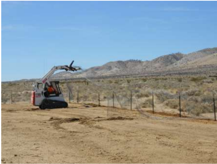
Figure 3: Moore Fence Company removing desert tortoise fence at Tower 17, Segment 10.
