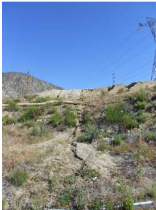
Figure 4: Erosion following a rain event, Segment 11D.
