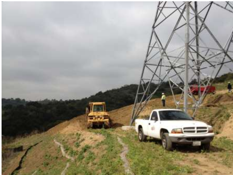
Figure 4: A DCX crew blades a tower pad, Segment 8, Phase 4.
