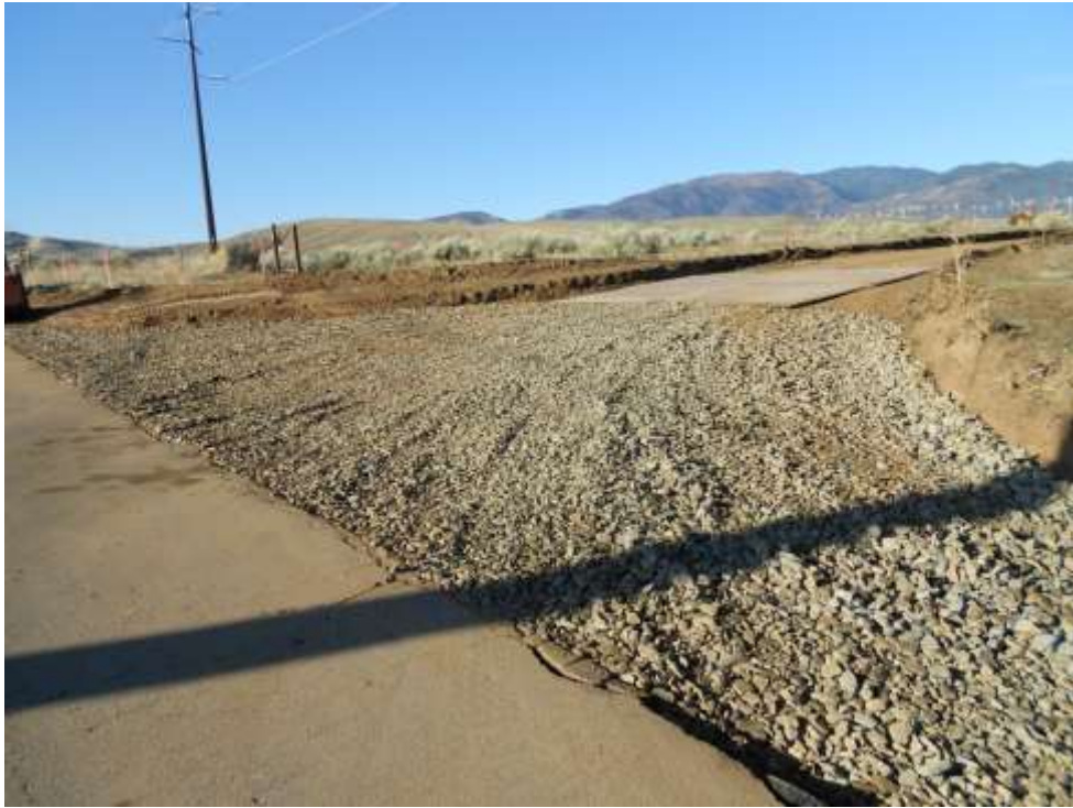
Figure 1: Gravel road entrance to Constructs 5 thru 7, Segment 3B.
