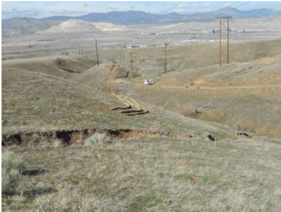
Figure 2: Straw wattle BMP's at Structure 14, Segment 3B.
