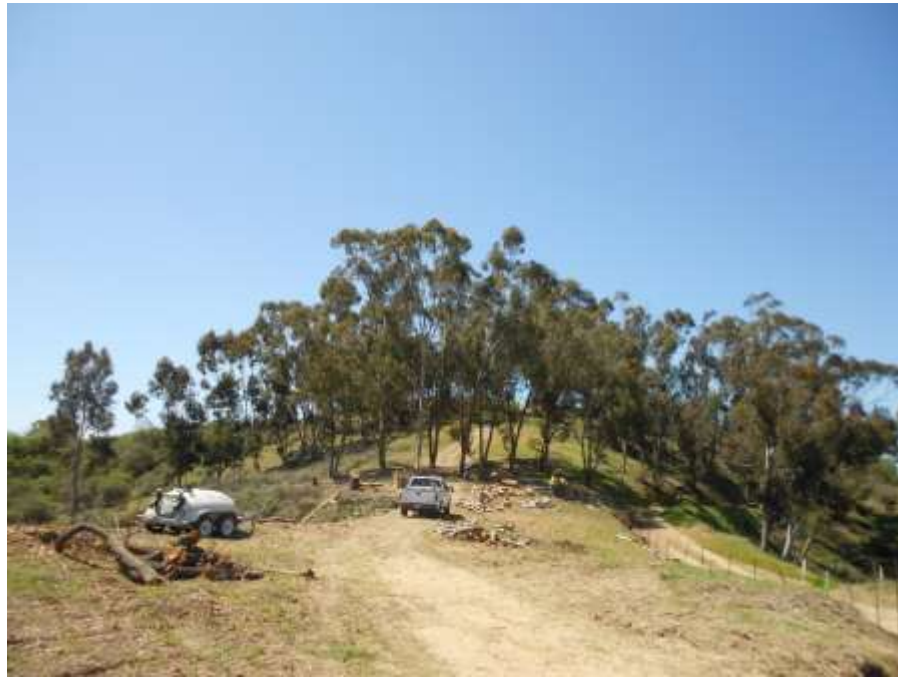
Figure 5: A DCX crew clears vegetation at Tower M49-T4, Segment 8, Phase 4.
