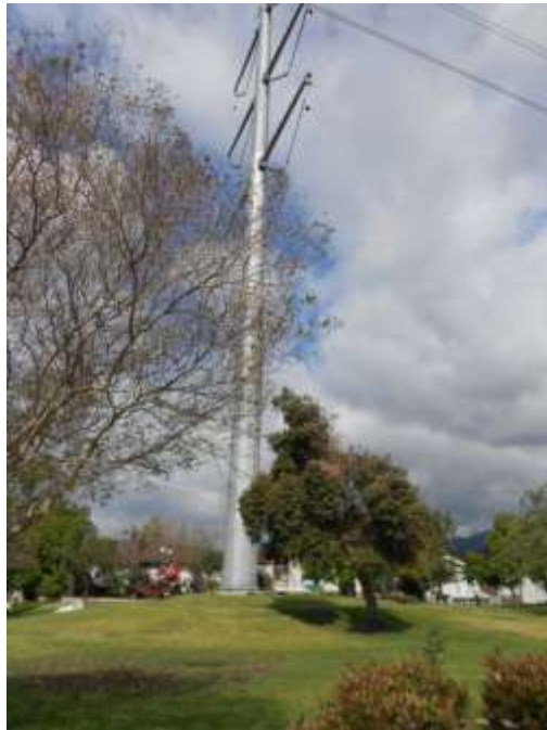
Figure 4: A crew installs counterpoise at Tower M28-P2, Segment 7.
