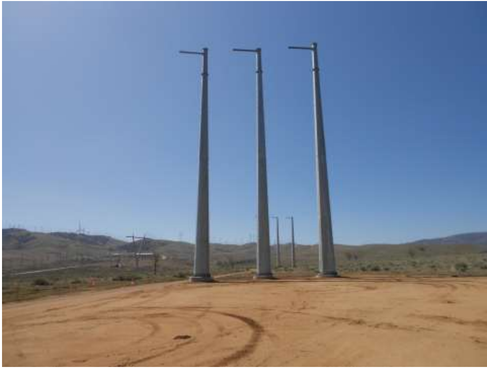
Figure 1: View of 3-pole Construct 1, Segment 3B.
