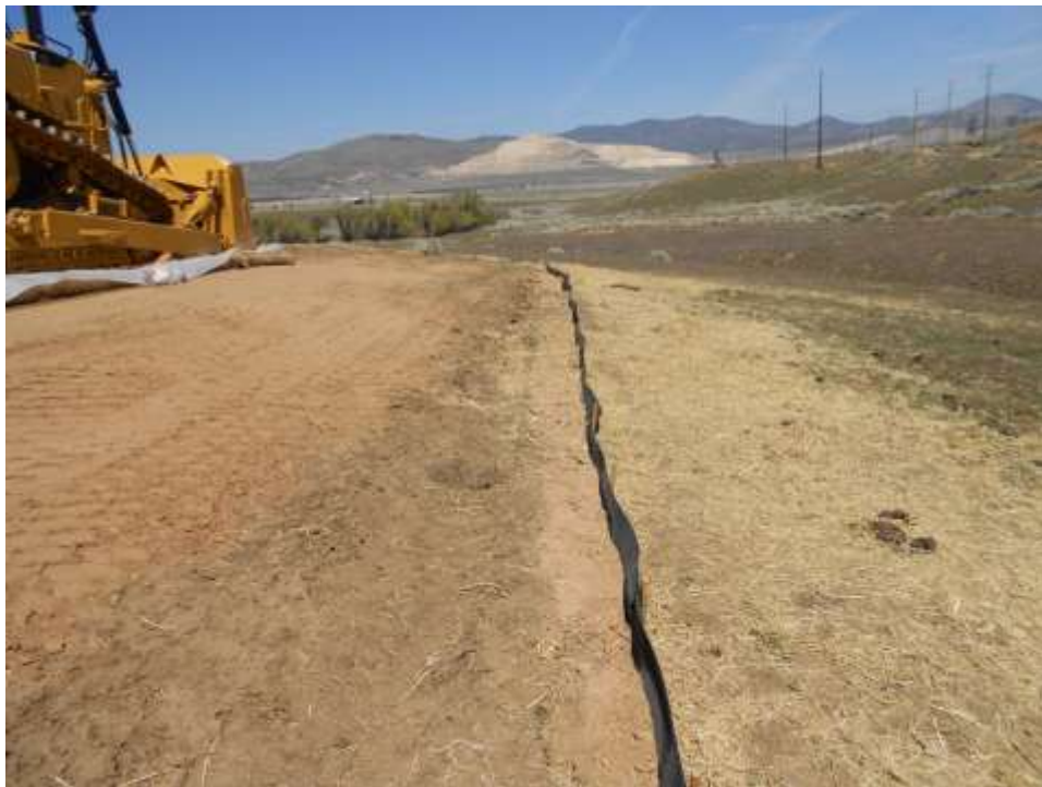
Figure 2: Newly installed Pro Wattle BMP's at Structure 9, Segment 3B.
