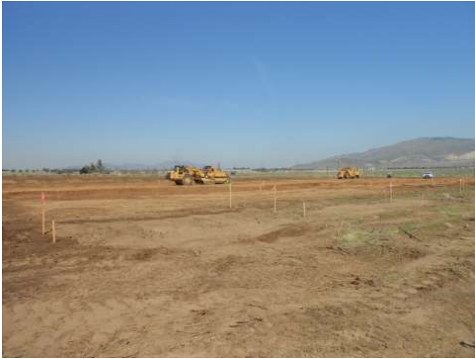
Figure 1: Grading activity at Highwind Substation, Segment 3B.
