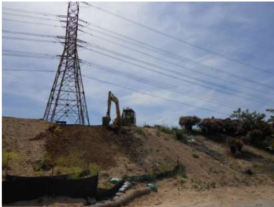
Figure 4: A crew repairs an eroded slope at Tower M42-T4, Segment 7.
