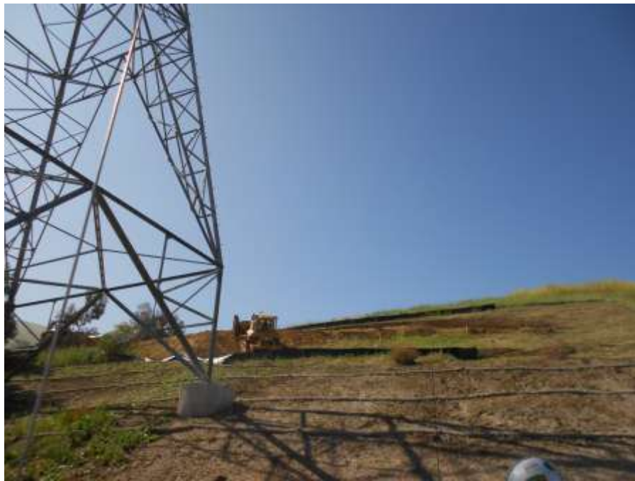
Figure 5: A crew grades a tower pad within Pathfinder Park, Segment 8 Phase 4.
