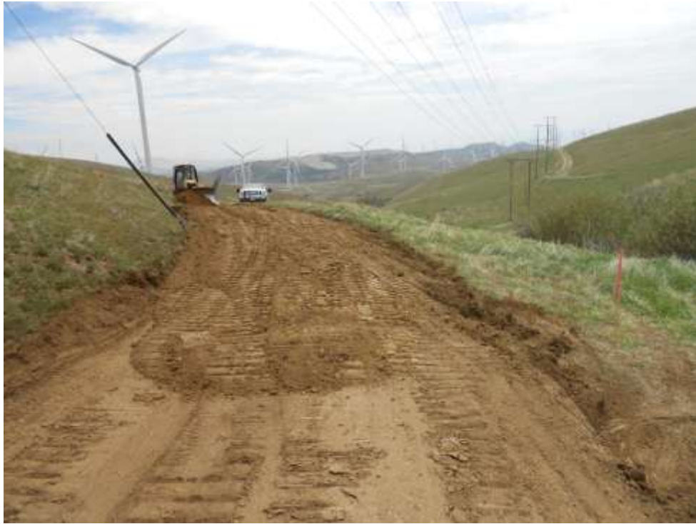
Figure 1: Grading new access road to Structure 27, Segment 3B.
