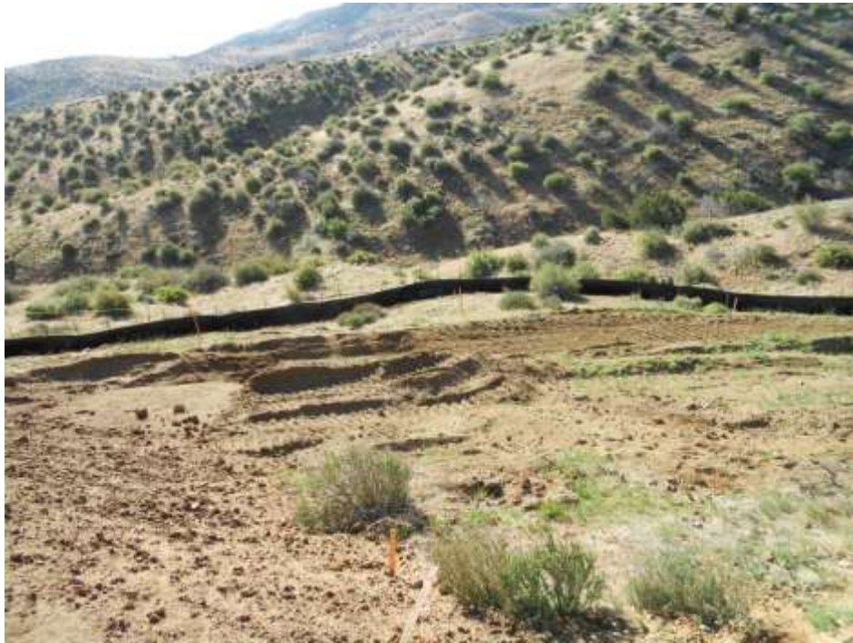
Figure 3: Silt fence installation to prevent further erosion at Construct 86A, Segment 5.
