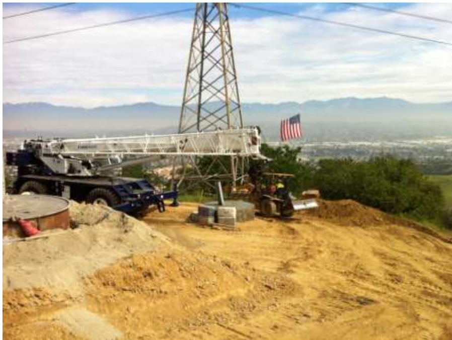
Figure 6: A crew grades a tower pad, Segment 8, Phase 4.
