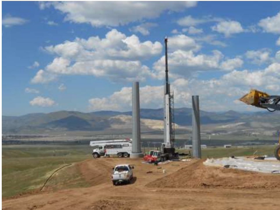
Figure 2: Erecting 3-pole Structure 14, Segment 3B.
