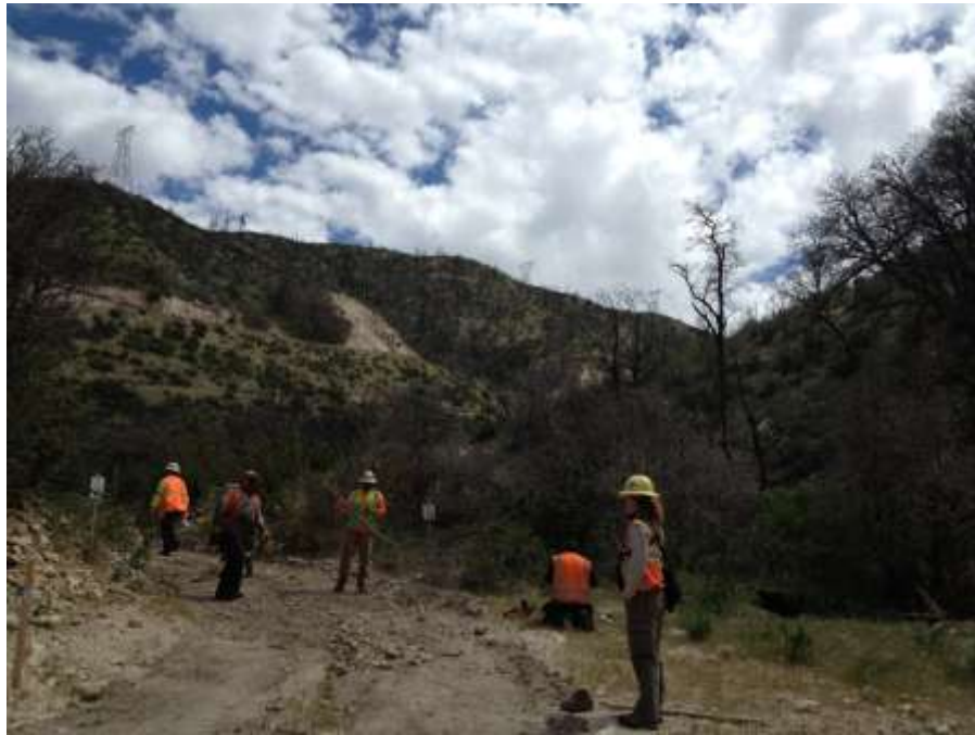
Figure 4: A crew removes vegetation along an access road, Segment 6B.
