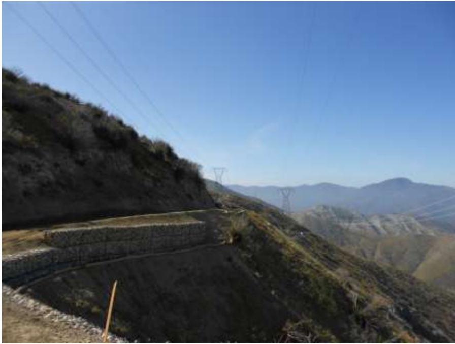
Figure 3: Newly installed gabion walls on Loop Road F, Segment 6B.
