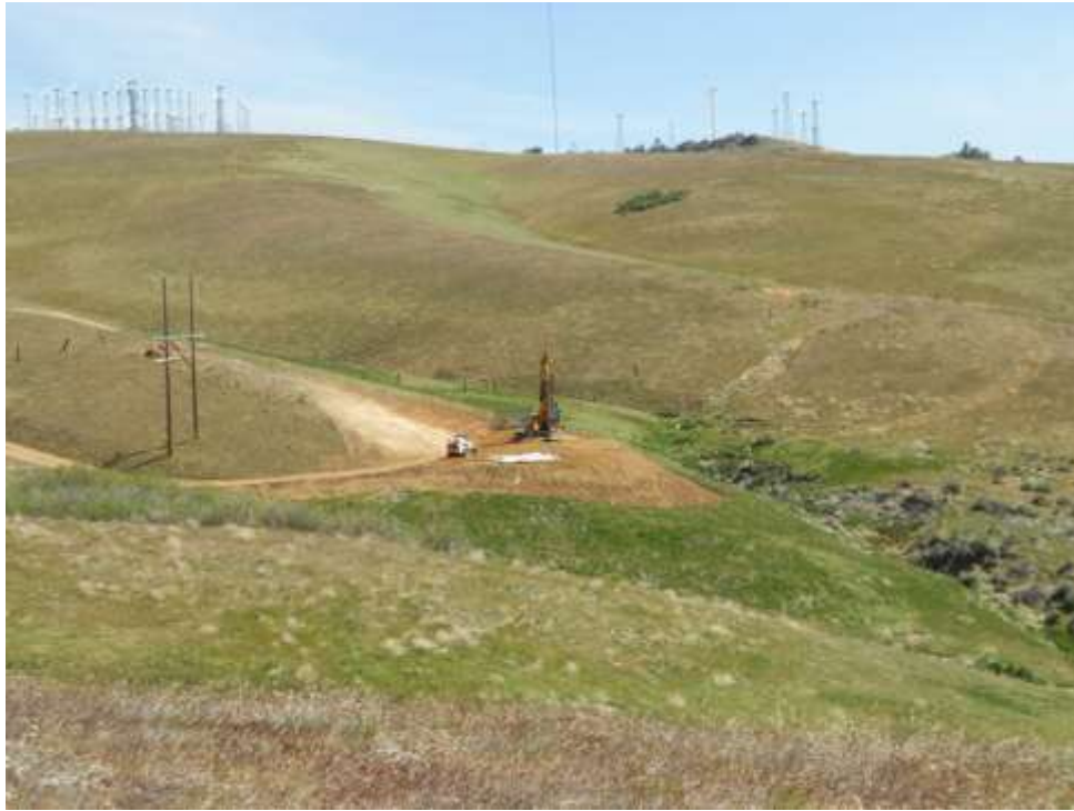
Figure 1: Drilling Structure 27, Segment 3B.
