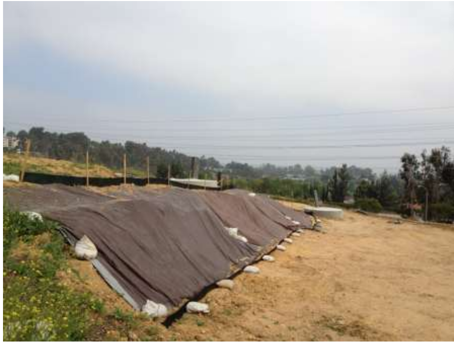
Figure 5: Newly installed BMPs, Segment 7.
