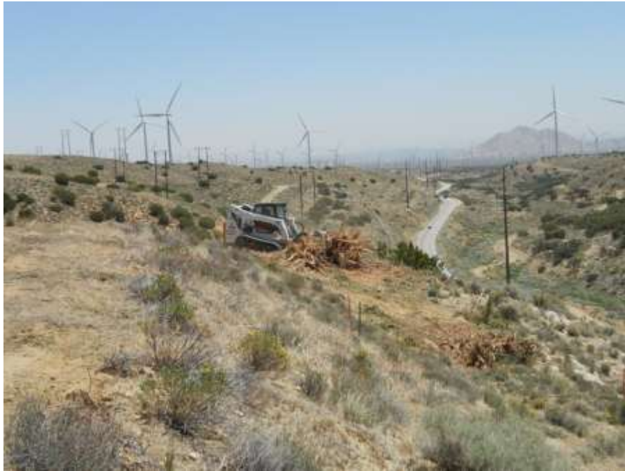
Figure 1: Grubbing activity at Structure 47, Segment 3B.
