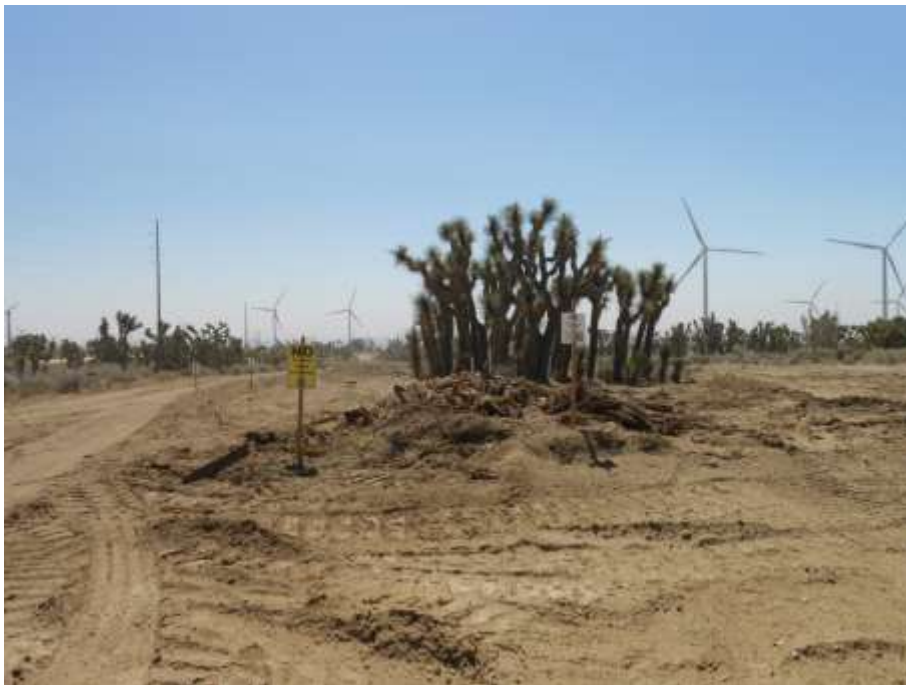
Figure 2: Environmentally Sensitive Area (ESA) buffer established for an active bird nest near Construct 66, Segment 3B.
