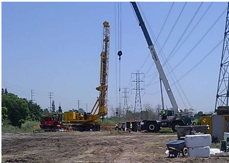
Figure 6: A crew drills a foundation, Segment 7.
