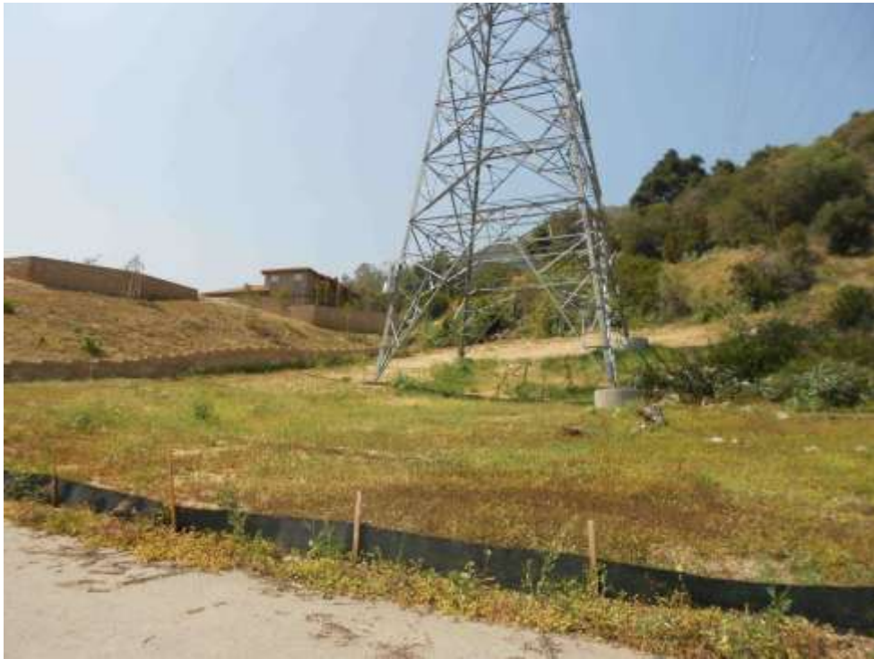
Figure 5: Watering of hydroseeded areas continued, Segment 7.
