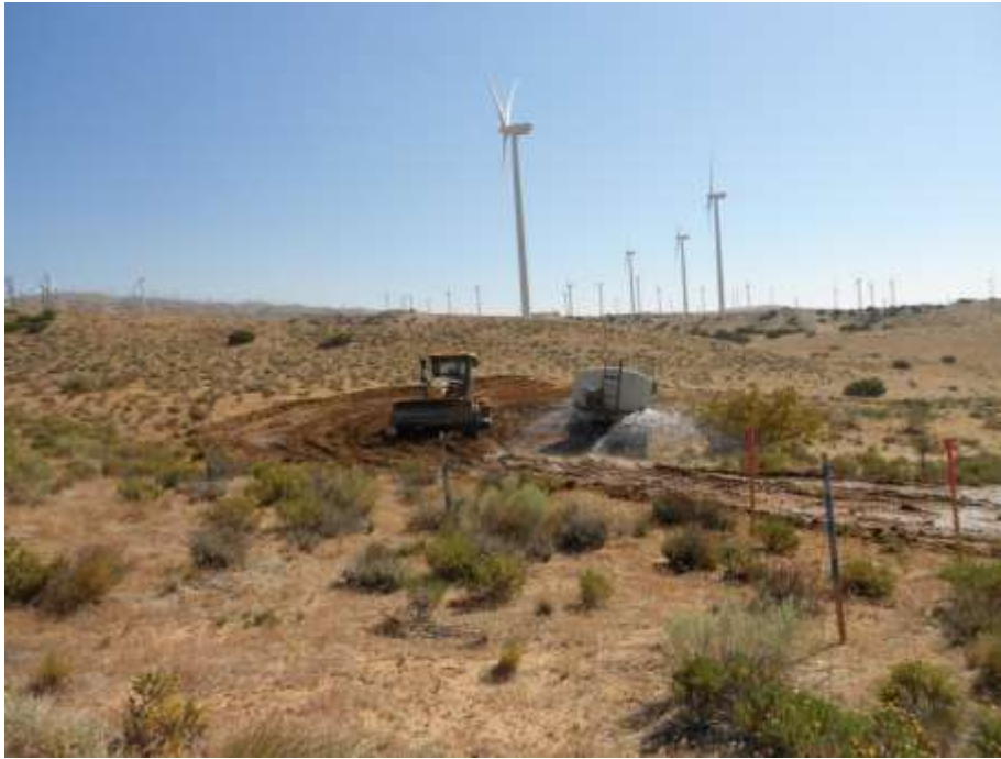
Figure 1: Grading activity at Structure 56, Segment 3B.
