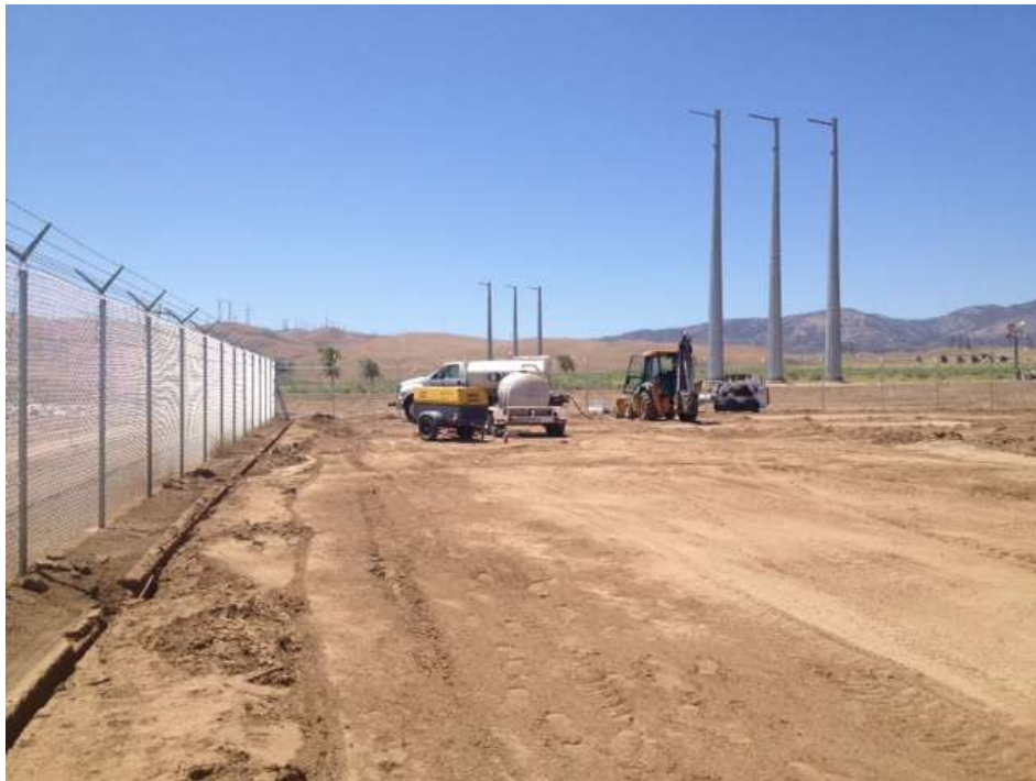
Figure 2: Perimeter fence installation at Highwind Substation, Segment 3B.
