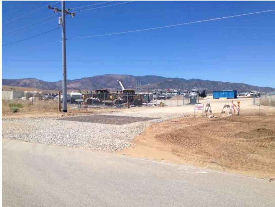
Figure 1: New shifted entrance to the Highwind Material Yard, Segment 3B.
