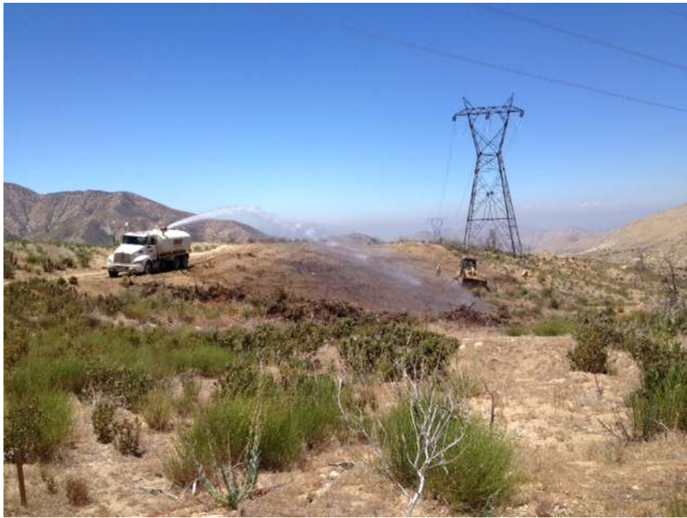
Figure 3: Grading of wire setup site (WSS) at Construct 22, Segment 6A.
