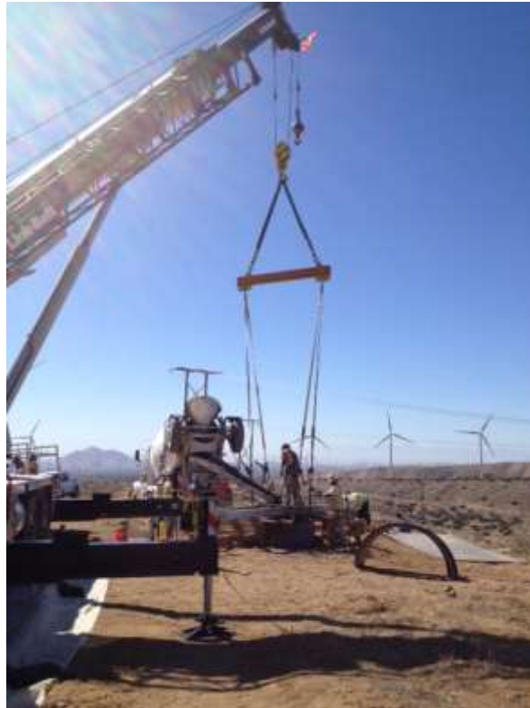
Figure 1: Concrete pour at Construct 50, Segment 3B.
