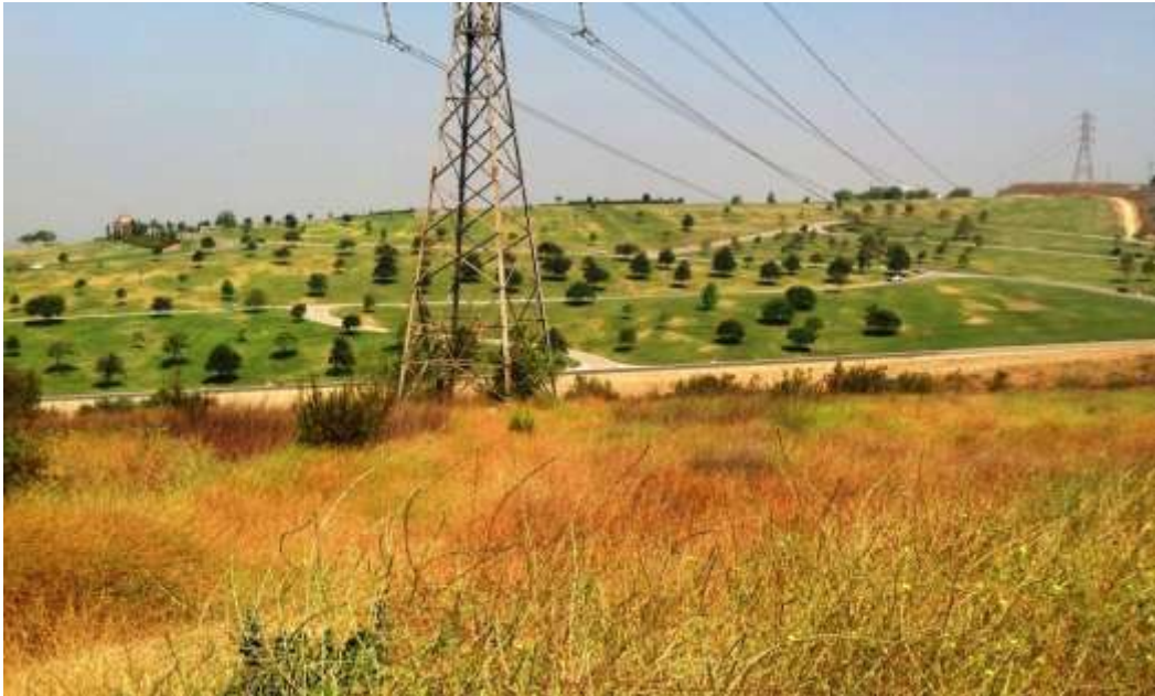
Figure 4: Least Bell's vireo nest buffer signs were installed near Rose Hills, Segment 8, Phase 4.
