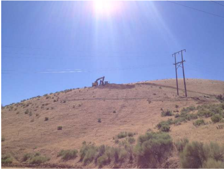
Figure 1: Grading at Construct 15, Segment 3B.
