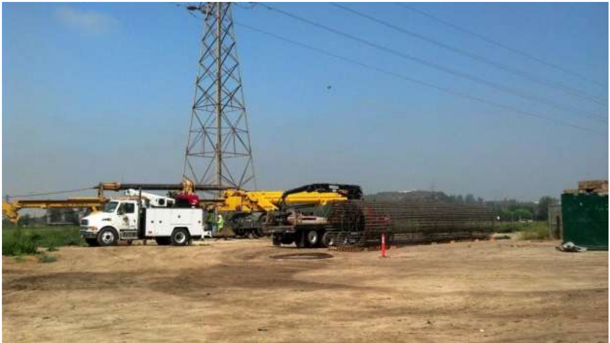
Figure 5: Tri-State preparing to set foundation cages on Segment 8, Phase 4.
