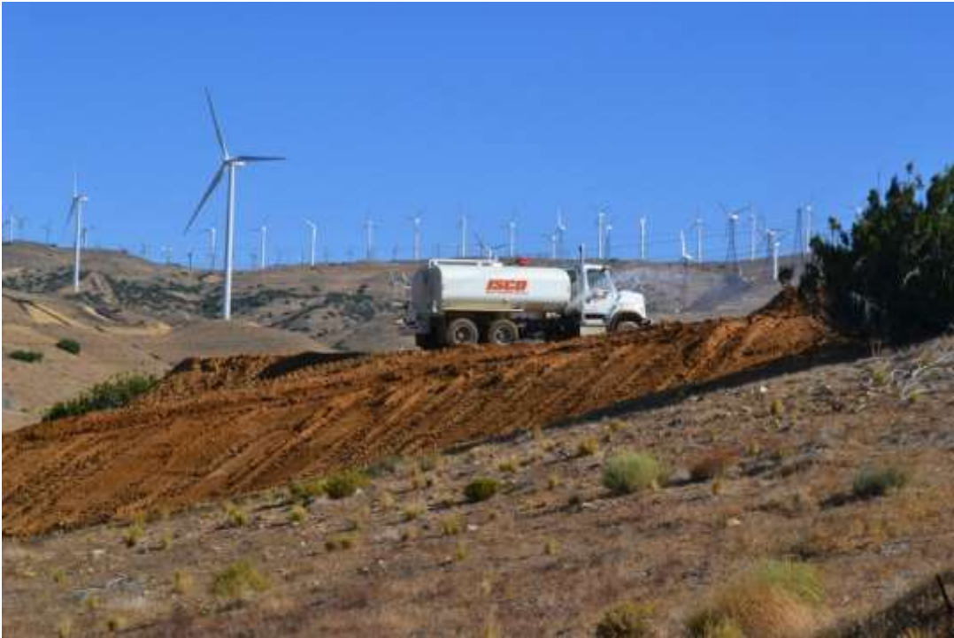
Figure 1: Grading and site preparation at Construct 57, Segment 3B.
