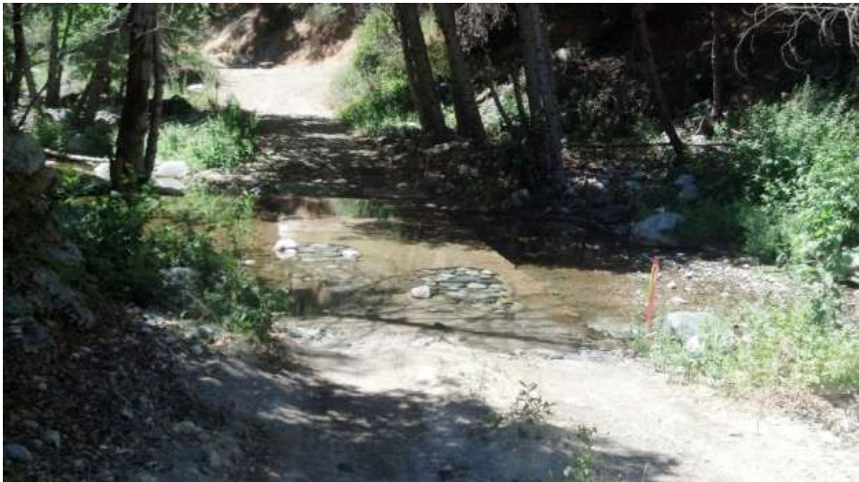
Figure 4: Wet crossing along Forest Service Road 2N23, Segment 6C. SCE has added river rock to the crossing, but a more permanent solution will be necessary for continued access across this feature.
