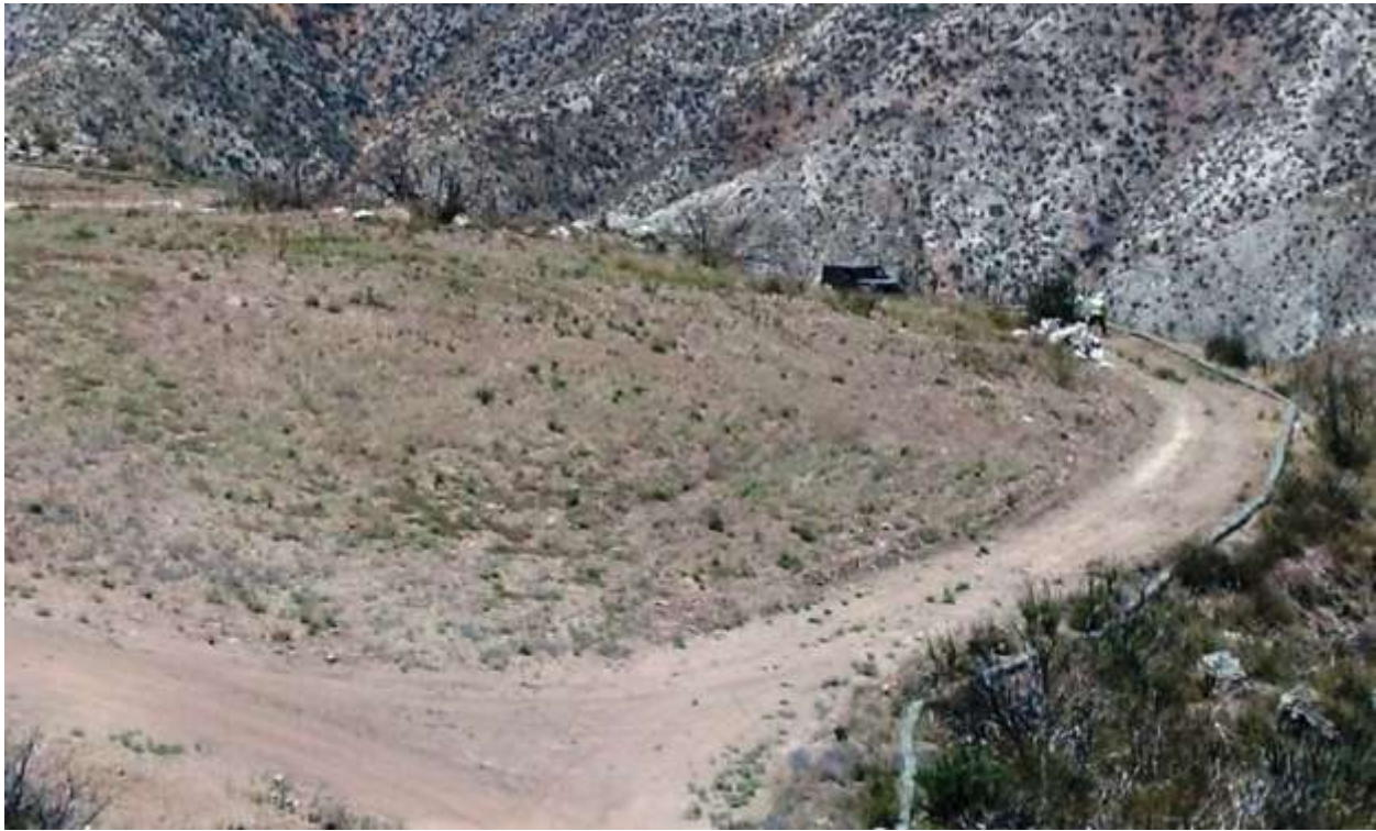
Figure 3: BMP installation along Loop Roads C and F.
