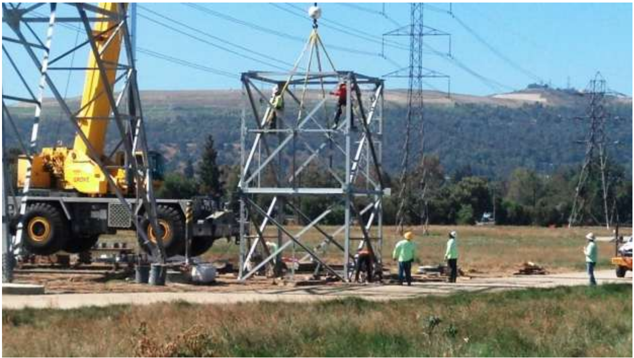
Figure 7: Tower assembly at Construct 36/1 on Segment 7.
