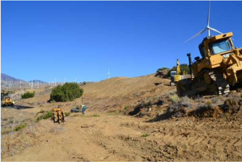
Figure 1: Grubbing and site preparation at Construct 48, Segment 3B.
