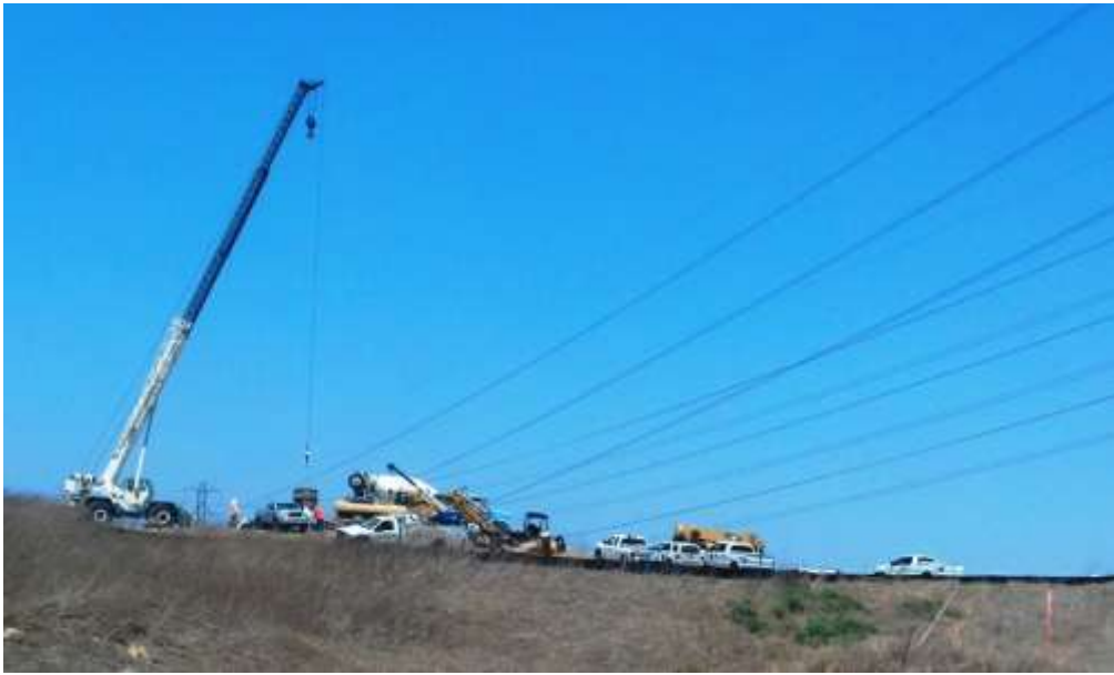
Figure 5: Setting foundation cages at Construct 51/2, Segment 8, Phase 4.
