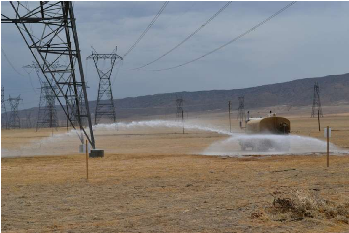
Figure 3: Soil binder application, Segment 4.
