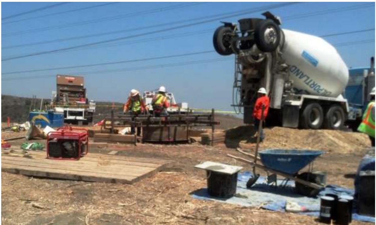
Figure 6: Pouring foundations at Construct 51/2, Segment 8, Phase 4.
