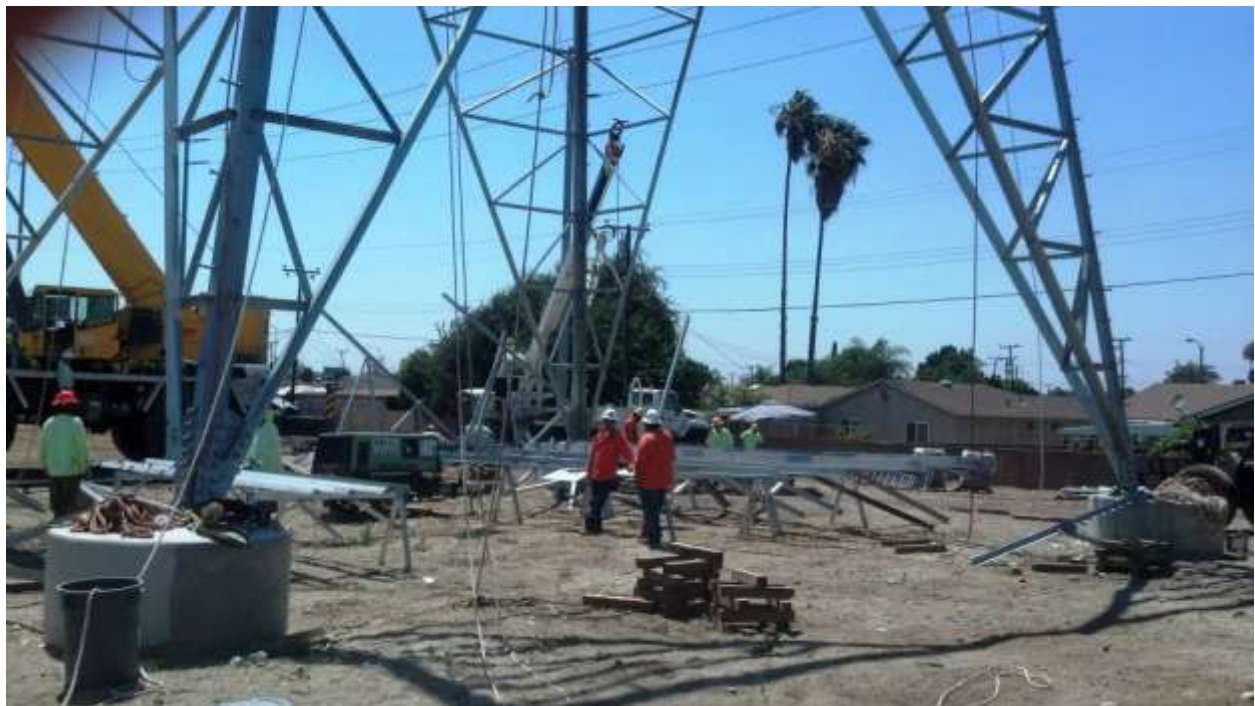
Figure 4: Tower erection at Construct 38/1, Segment 7.
