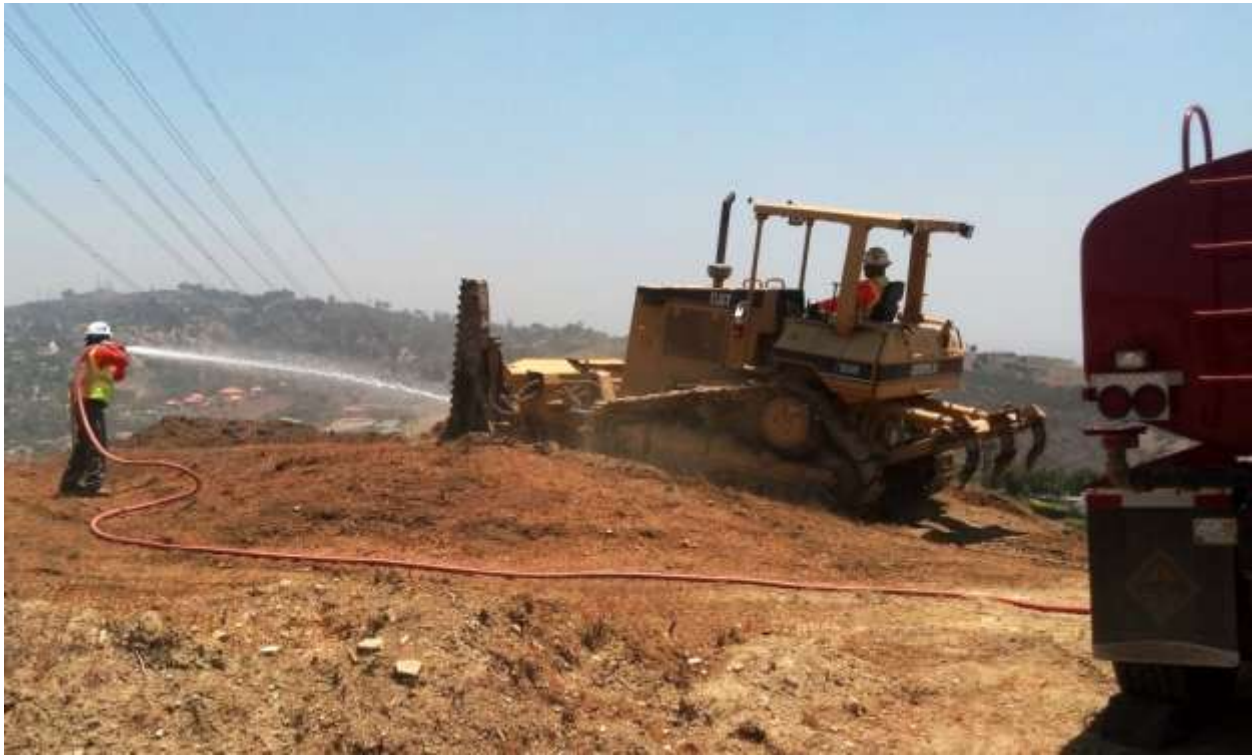
Figure 7: Dust control during pad recontouring at Construct 47/3, Segment 8, Phase 4.
