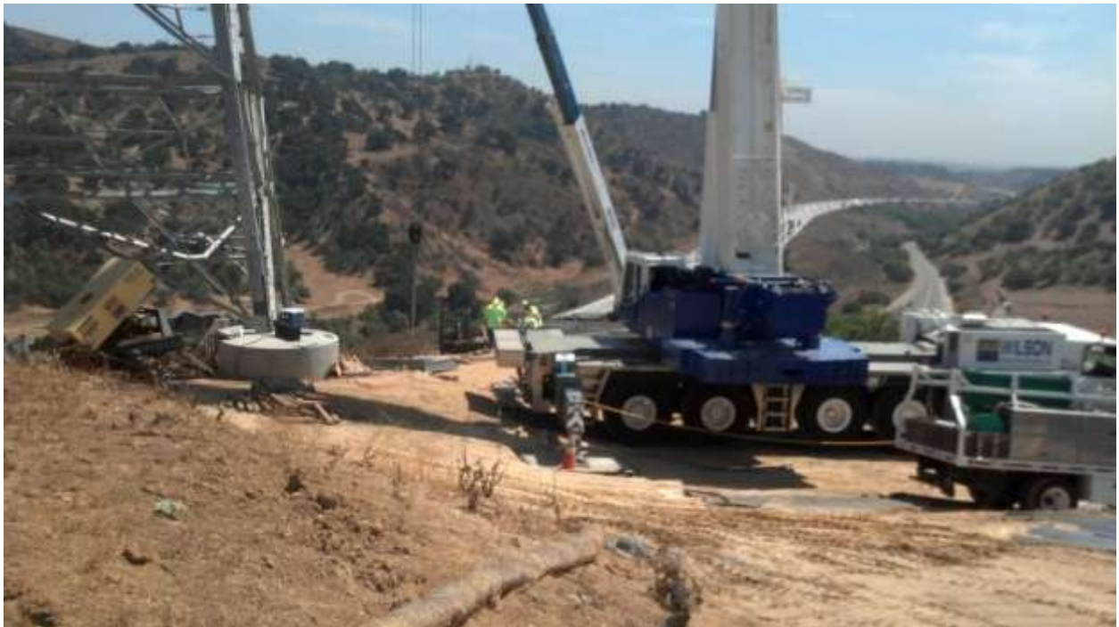
Figure 7: Assembly at Tower 55/1, Segment 8 Phase 4.
