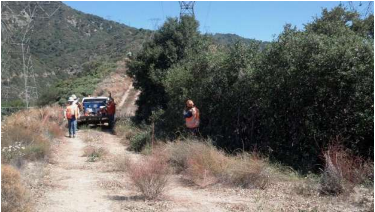
Figure 5: Vegetation trimming on Segment 6C.
