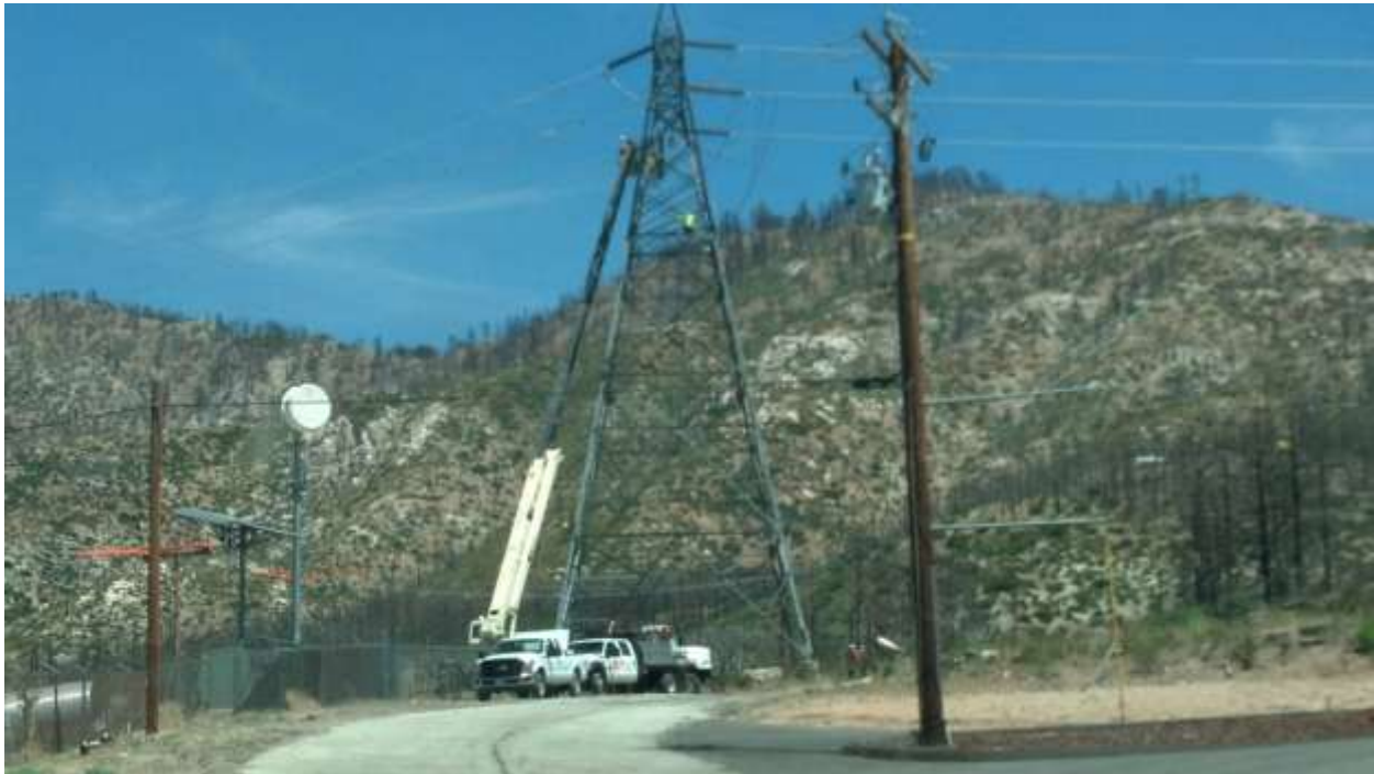
Figure 3: Crews removing wire on Segment 6, structure 35.
