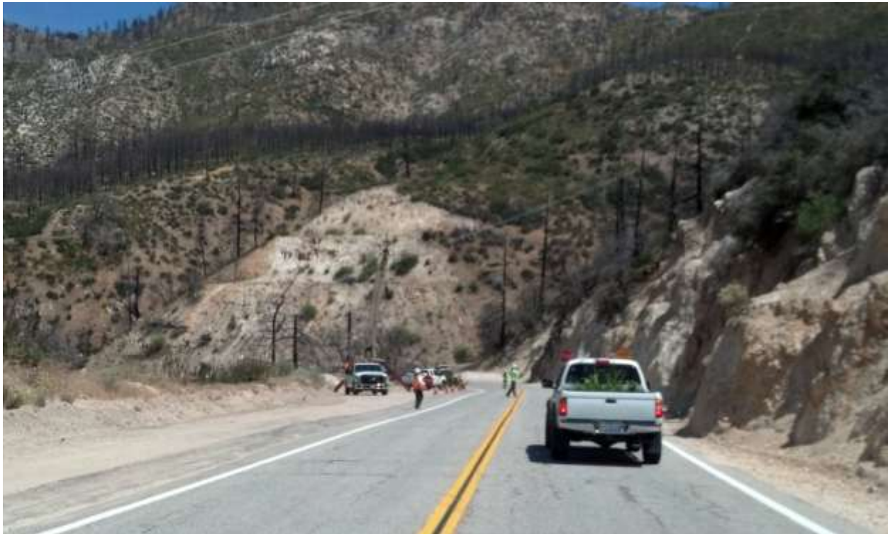
Figure 4: Traffic control on Angeles Crest Highway during Segment 6 during wire removal.
