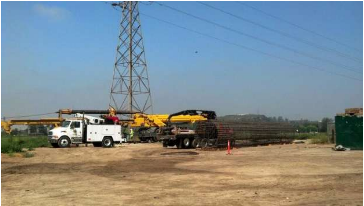
Figure 8: Tri-State crews preparing to set large cages at Tower 41/2, Segment 8 Phase 4.
