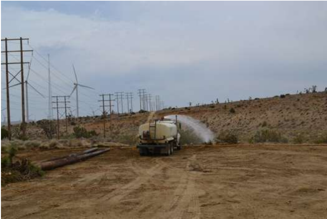
Figure 1: Grubbing at Wire Set up Site near Tower 62, Segment 3B.
