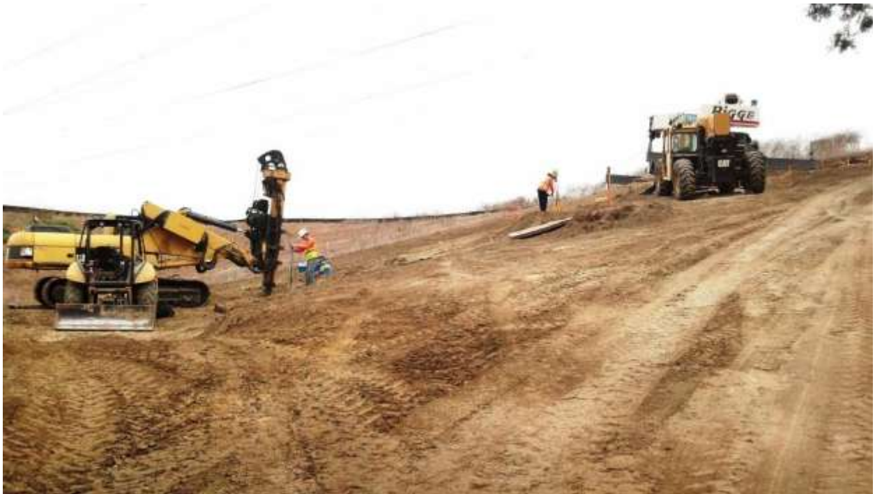
Figure 9: Foundation excavation on Segment 8, Phase 4.
