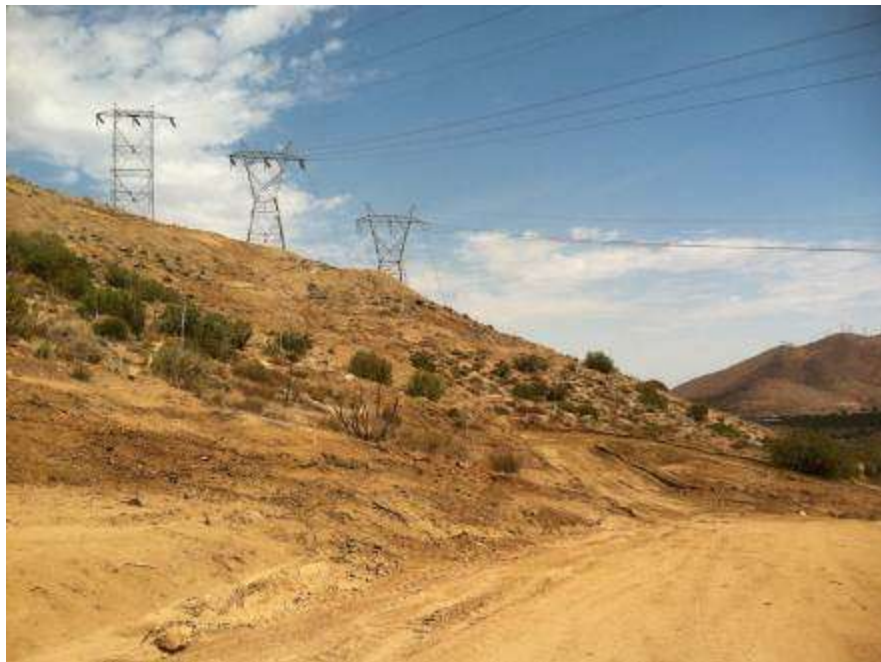
Figure 2: Completed grading at HSY 1/2 (north) on Segment 6A.
