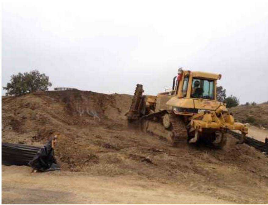
Figure 5: Crane pad building on Segment 8, Phase 4.
