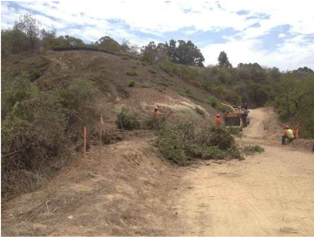
Figure 3: Vegetation trimming on Segment 8, Phase 4.
