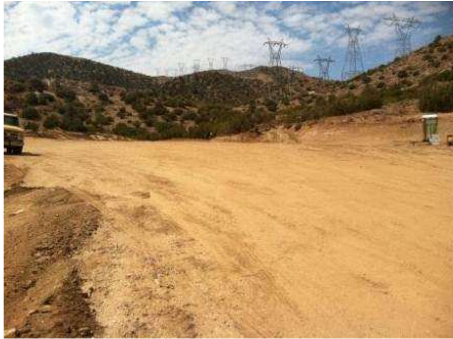
Figure 1: Completed grading at HSY 1/2 (south) on Segment 6A.
