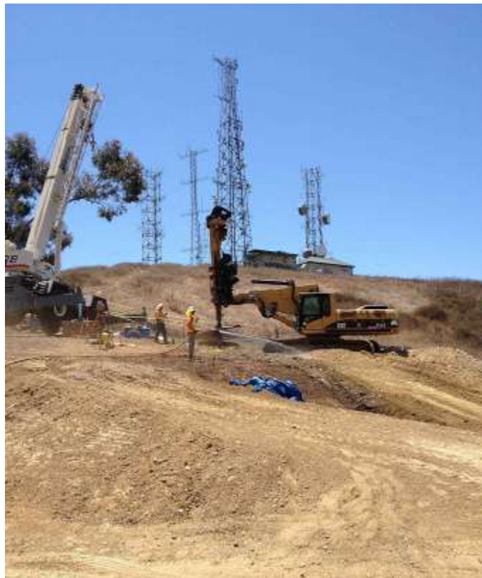
Figure 4: Foundation drilling, Segment 8, Phase 4.
