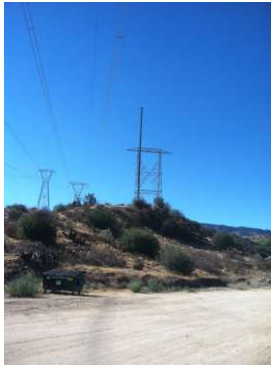
Figure 2: Structure removal of M79-T2 on Segment 6A.
