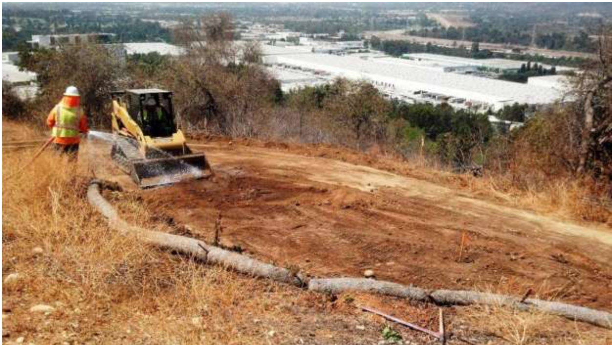
Figure 7: Dust control during grading at M43-T2, Segment 8, Phase 4.
