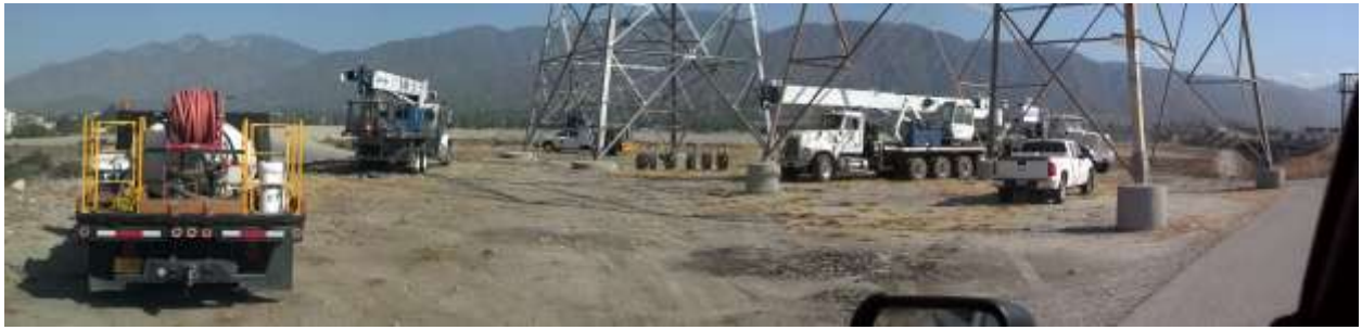
Figure 5: Preparations for wire pull on Segment 7.
