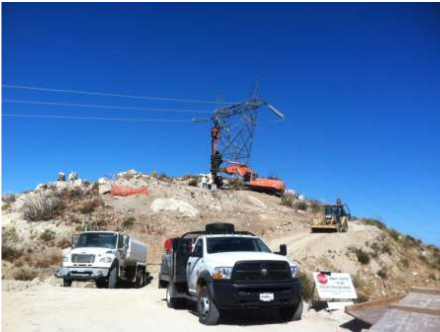
Figure 4: Foundation excavation at Construct 24 on Segment 6A.
