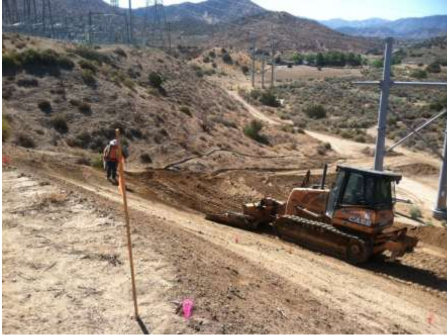
Figure 1: Access road grading at Construct 1 on Segment 6A.
