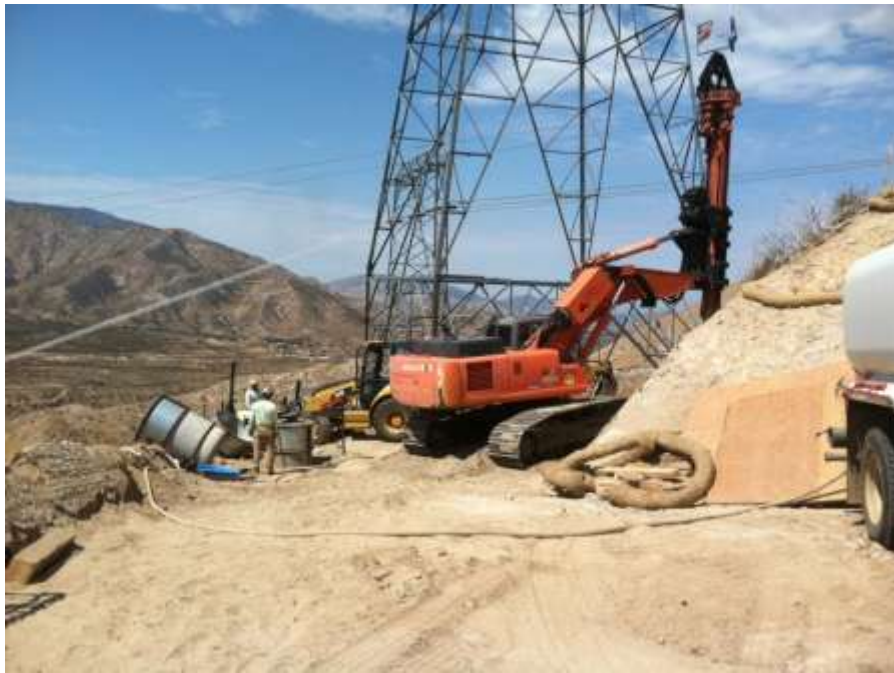
Figure 3: Foundation excavation at Construct 20 on Segment 6A.
