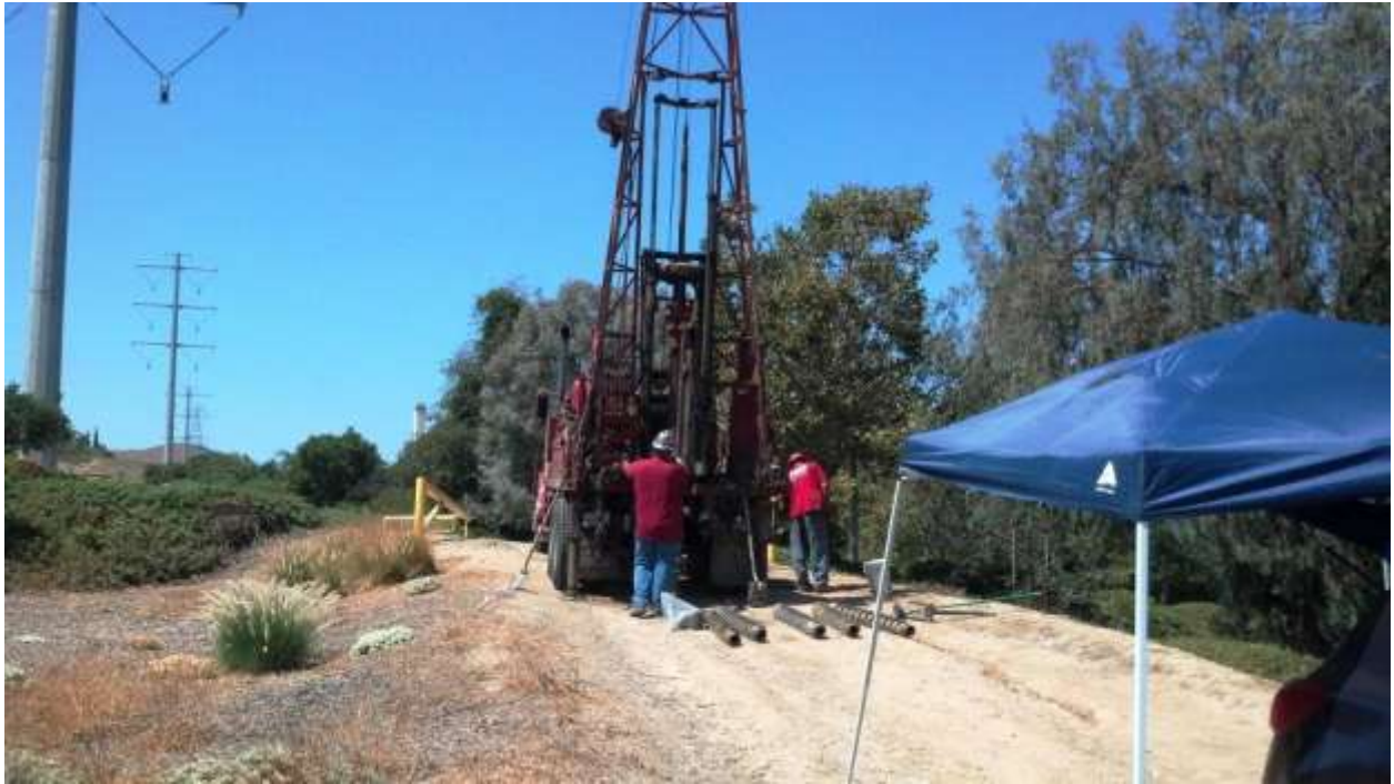
Figure 6: Geotechnical boring on Segment 8, Phase 1, in Chino Hills.
