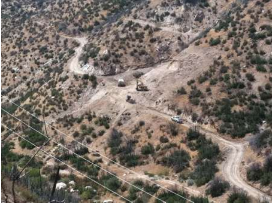
Figure 1: Grading activities occurring at Construct 33 on Segment 6A.
