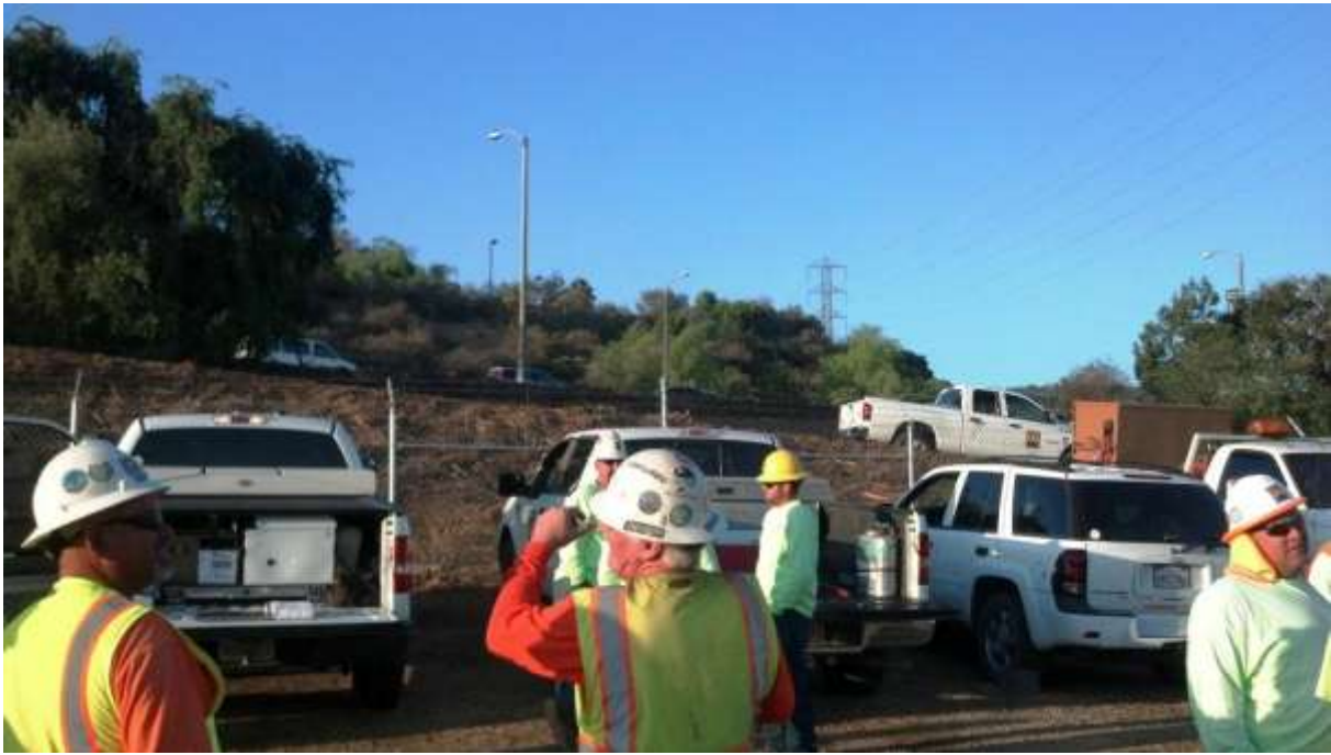
Figure 5: A stand of vegetation was mowed down at the Fullerton Construction Yard on Segment 8, Phase 4, making the yard visible from the adjacent public road.
