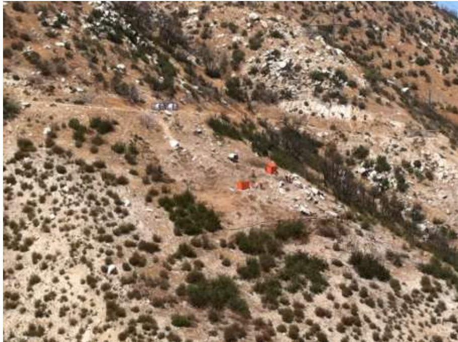
Figure 2: BMP installation at micropile preparation area at Construct 31 on Segment 6A.
