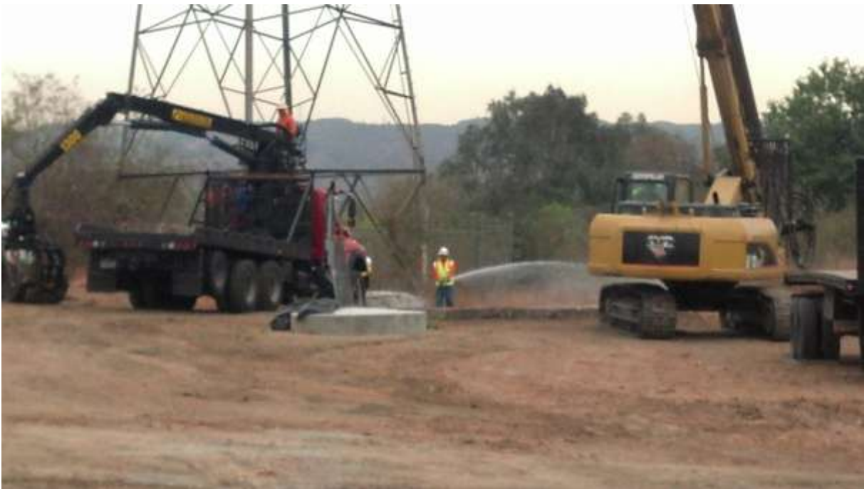
Figure 4: Dust control at Construct M40-T4 foundation work on Segment 8, Phase 4.
