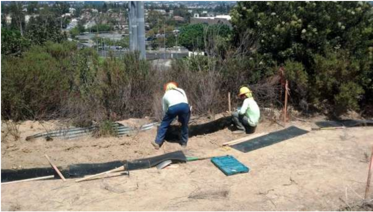
Figure 3: DCX crews install silt fence at Construct M41-T3 on Segment 7.
