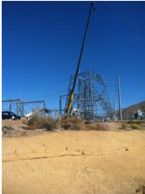
Figure 6: Segment 6 structure assembly at Construct 2.
