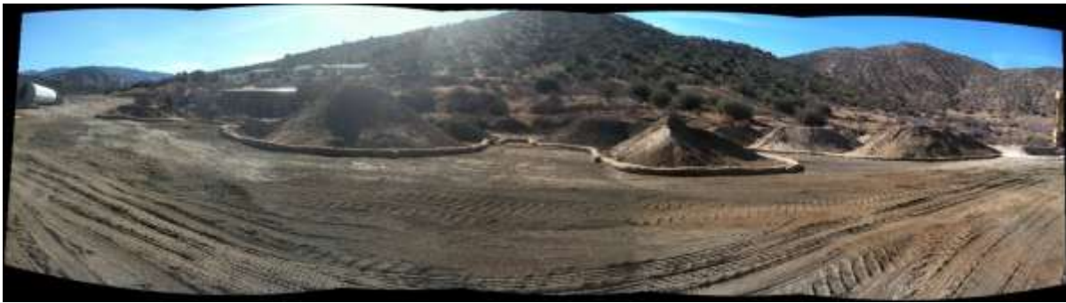
Figure 7: Segment 6 BMP installation at wire pull site between Construct 11 and 12.
