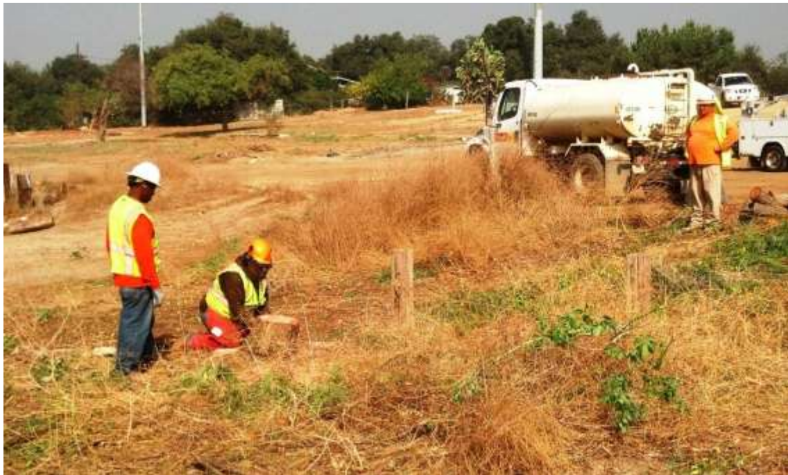
Figure 10: Crew performing tree removal at M40-T4 on Segment 7.
