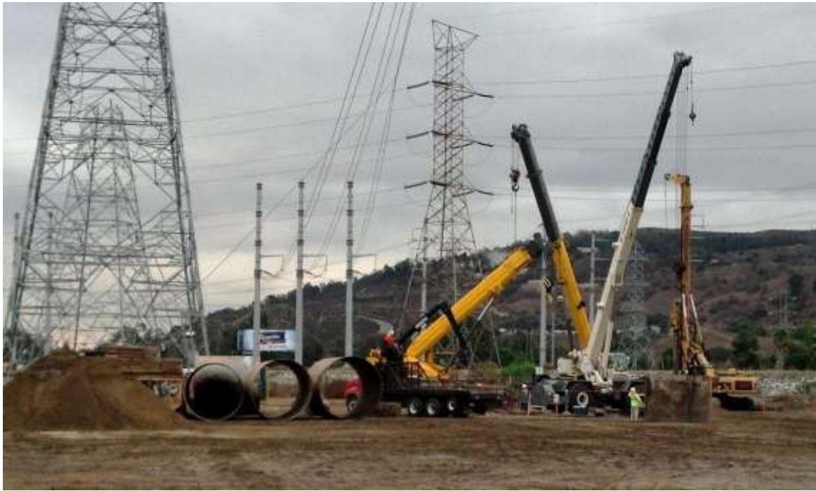
Figure 11: Foundation excavation at Tower M42-T5A, Segment 8, Phase 4.
