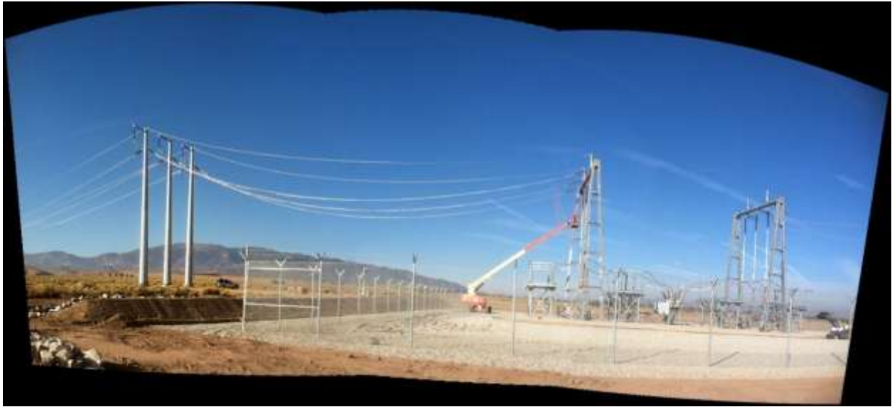
Figure 1: Segment 3B Wire Stringing operations at Construct 1 into Highwind Substation.
