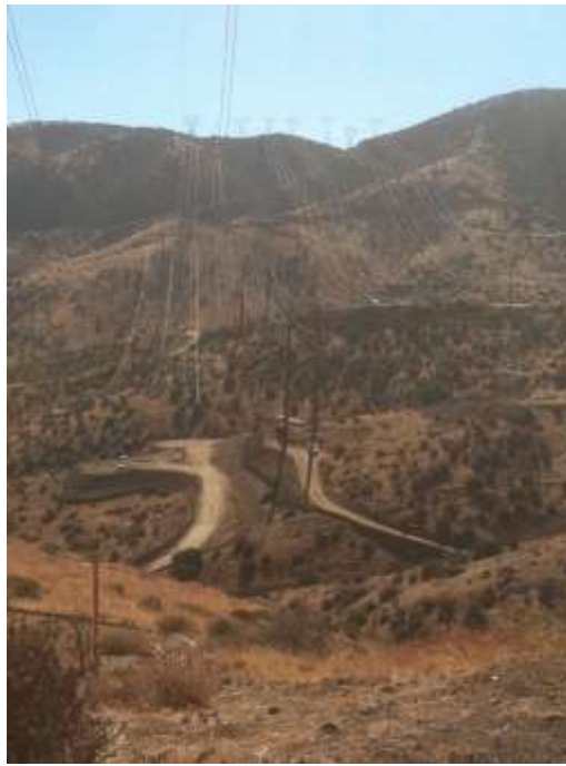
Figure 5: Sagebrush wire pulling activities at Construct 235A.
