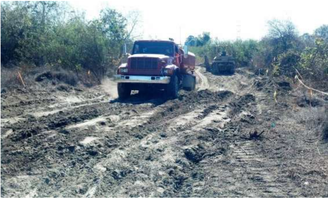
Figure 13: Access road construction at M42-T1A, Segment 8, Phase 4.
