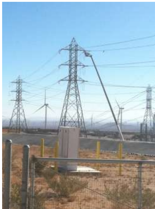
Figure 2: Segment 3B wire stringing operations at Construct 72 into Windhub Substation.
