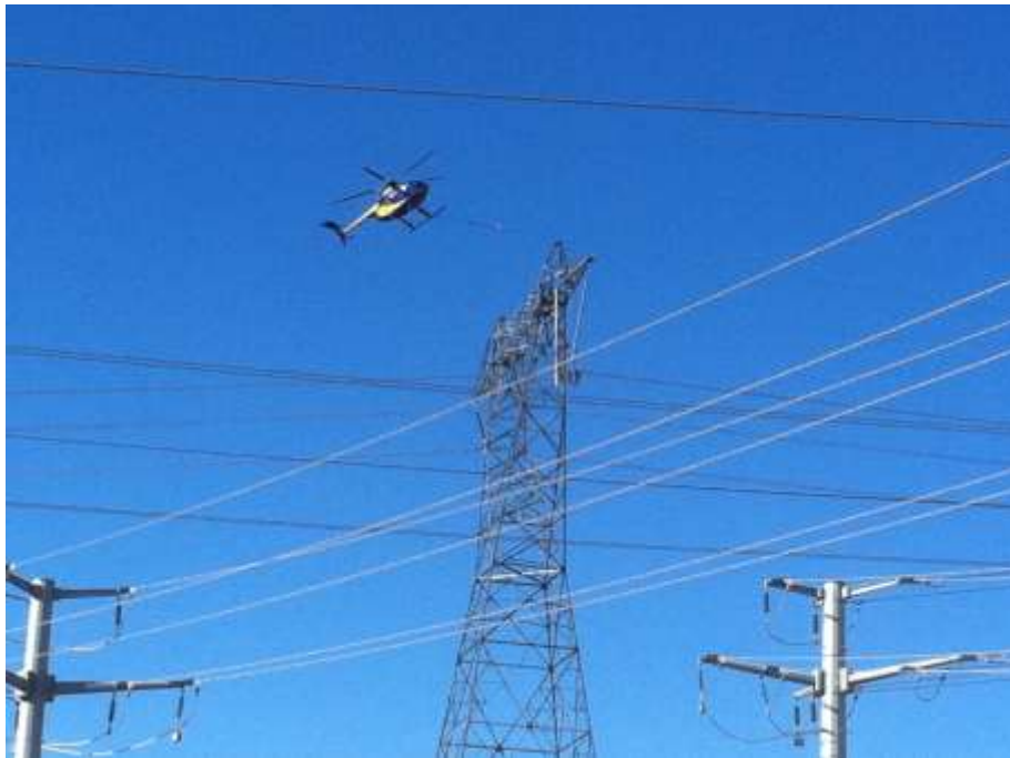
Figure 4: Segment 5 wire pulling operations at Construct 37.
