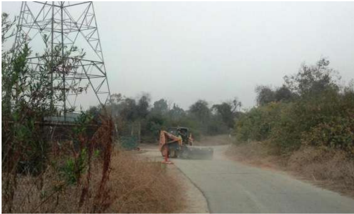
Figure 12: Cleaning up tracked-out dirt at Tower M42-T1A, Segment 8, Phase 4.
