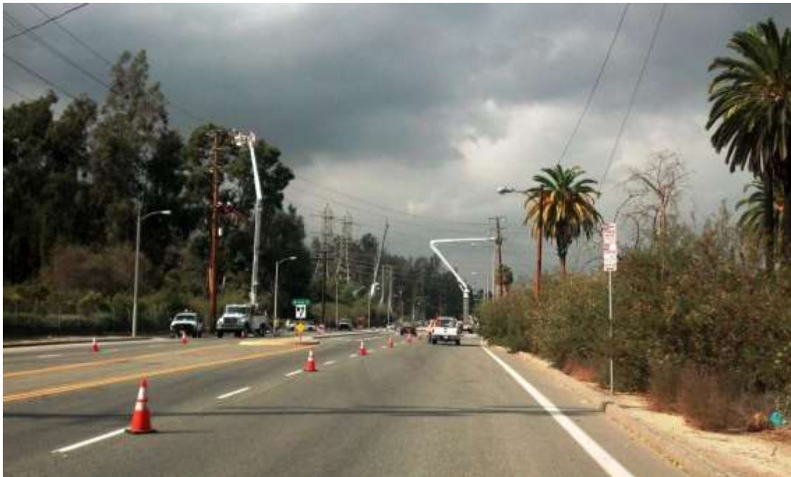
Figure 8: 66 kV work along San Gabriel Boulevard, Segment 7.
