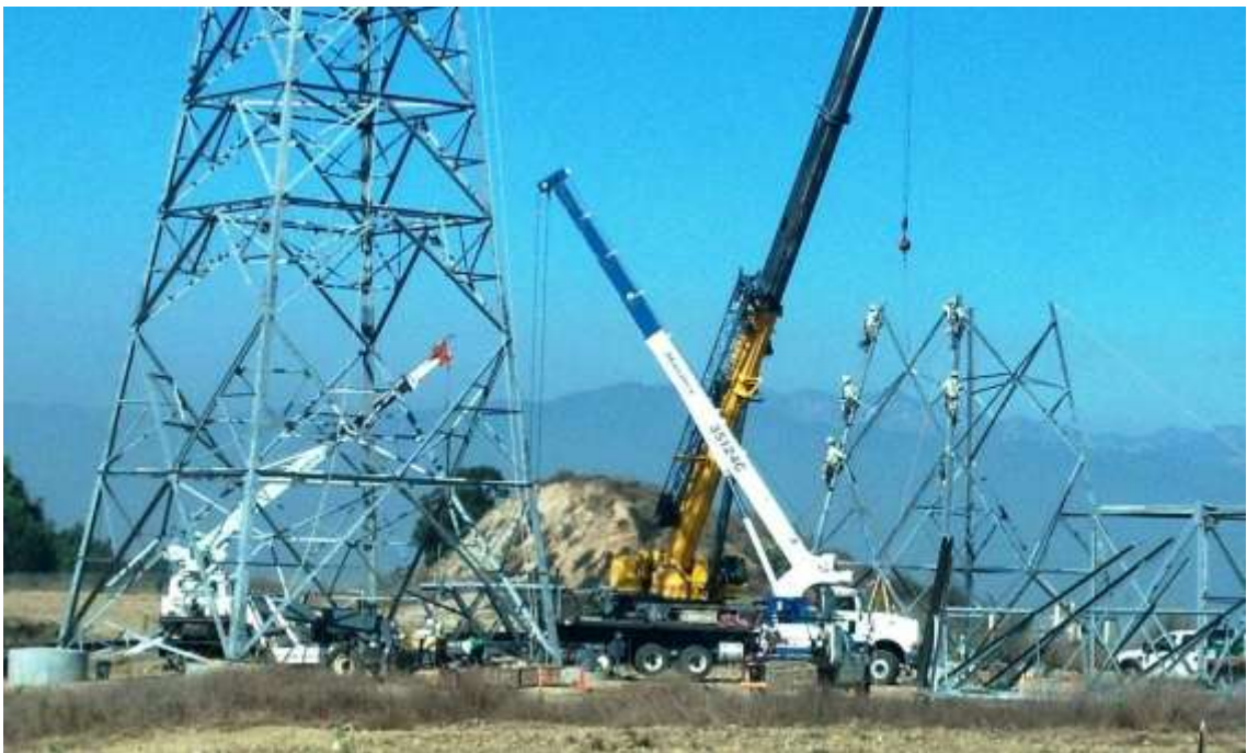
Figure 14: Tower erection at M45-T2, Segment 8, Phase 4.
