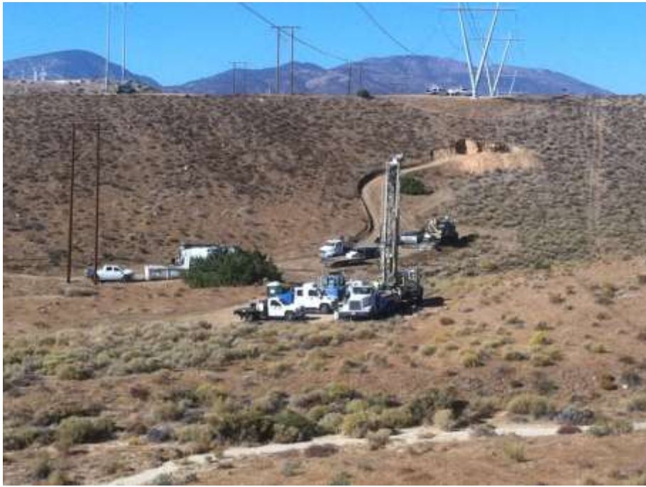
Figure 3: Segment 3B AC Mitigation well drilling operations.
