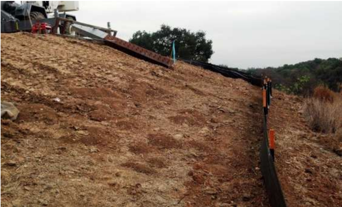
Figure 6: Silt fencing maintained at M45-T3, Segment 8, Phase 4.
