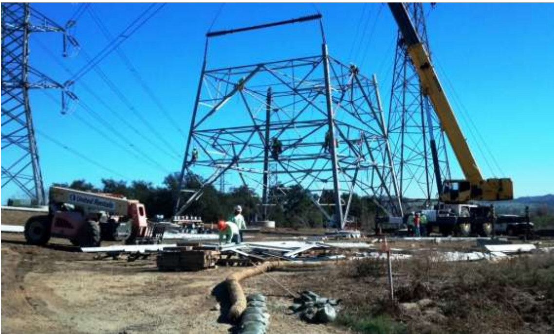
Figure 8: Tower assembly at M40-T4, Segment 8, Phase 4.
