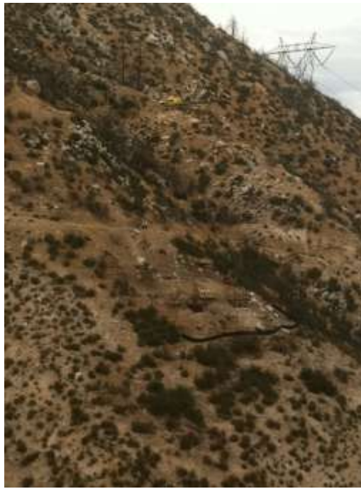
Figure 3: Segment 6 micropile operations at Construct 28.
