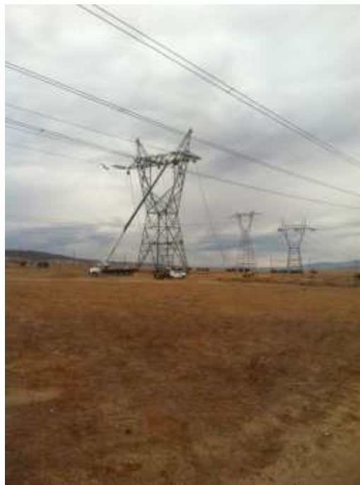
Figure 2: Segment 5 wire operations at Construct 7.
