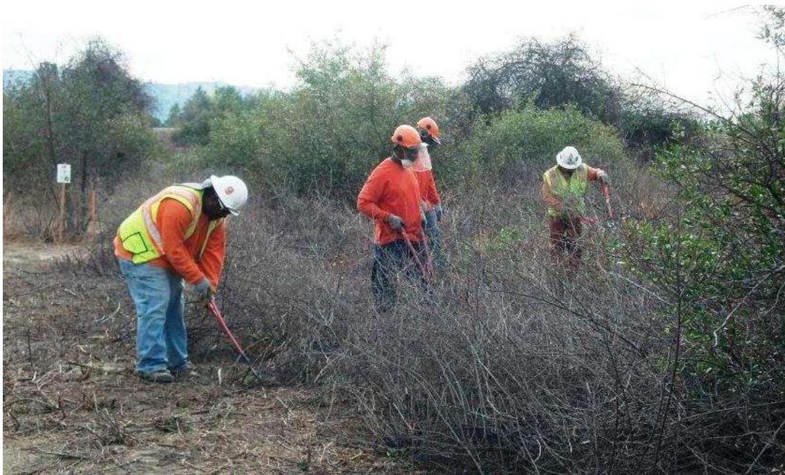
Figure 4: Vegetation clearing at Wire Setup Site 7.56, Segment 7.
