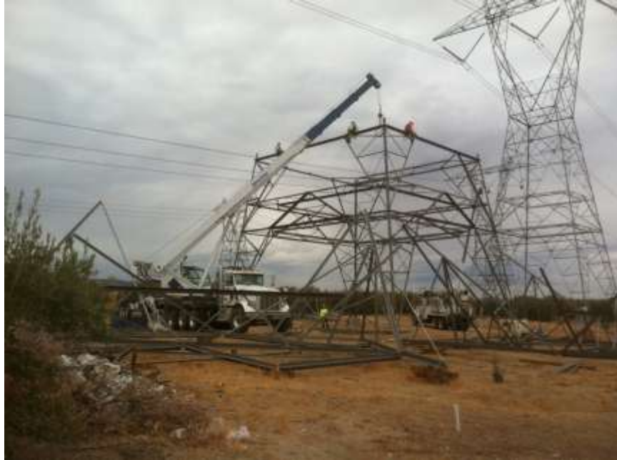
Figure 1: Segment 5 structure erection at Construct M90-T1X.
