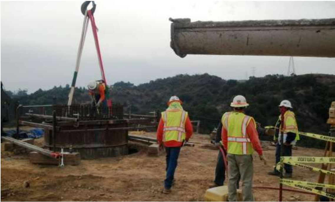
Figure 7: Foundation pouring at M45-T3, Segment 8, Phase 4.
